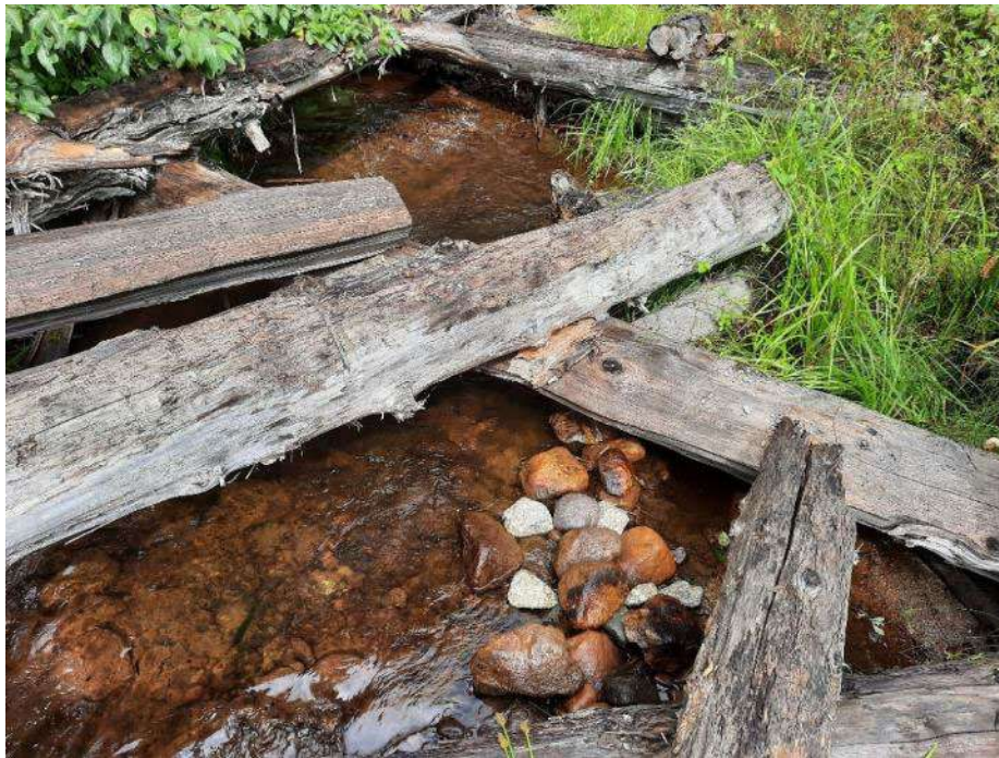
Figure 7. Cobble placement at the head of the side channel upstream of ALE-XS1 on August 06, 2020.
