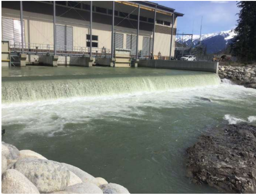
Figure 7. Looking upstream at ULL-TAILWQ on May 11, 2021.
