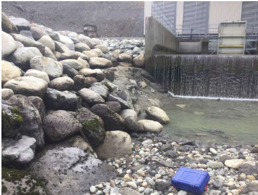
Figure 10. Looking upstream at ULL-TAILWQ on October 21, 2021.
