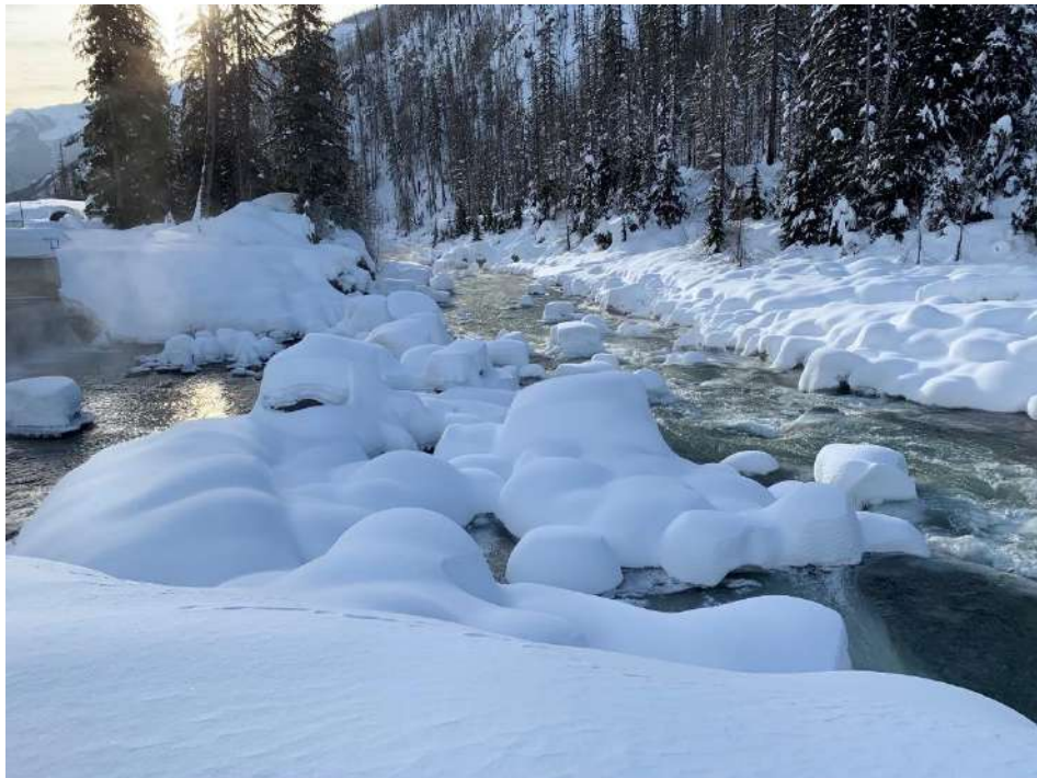
Figure 14. Looking downstream at Upper Lillooet from the tailrace on December 28, 2021.
