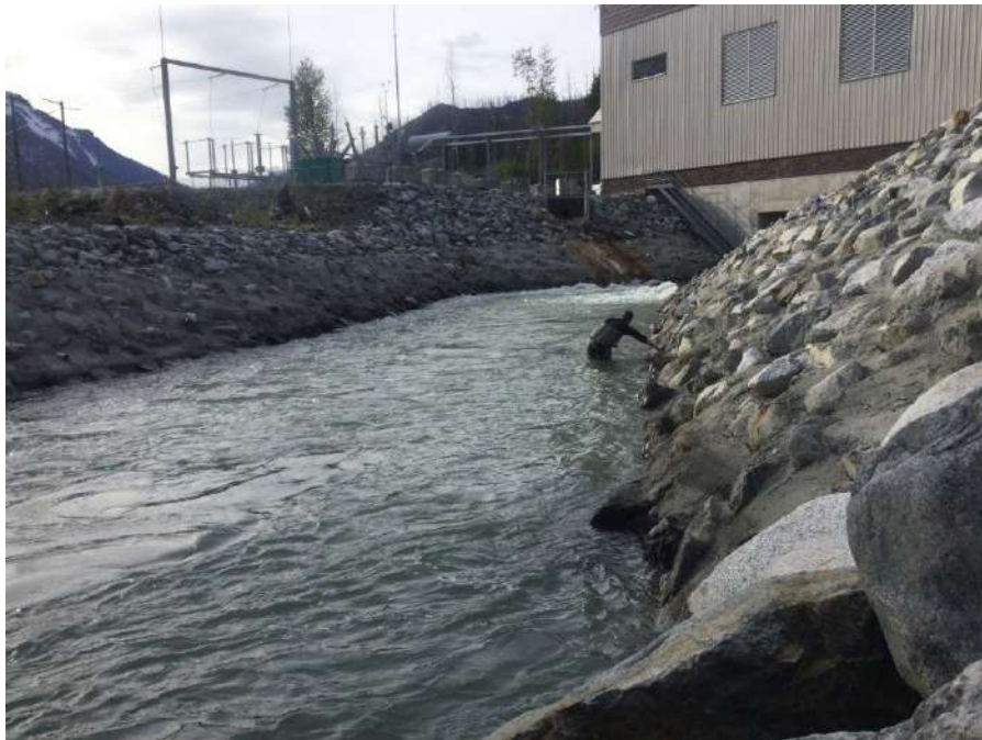
Figure 24. Looking upstream at BDR-TAILWQ on May 11, 2021.
