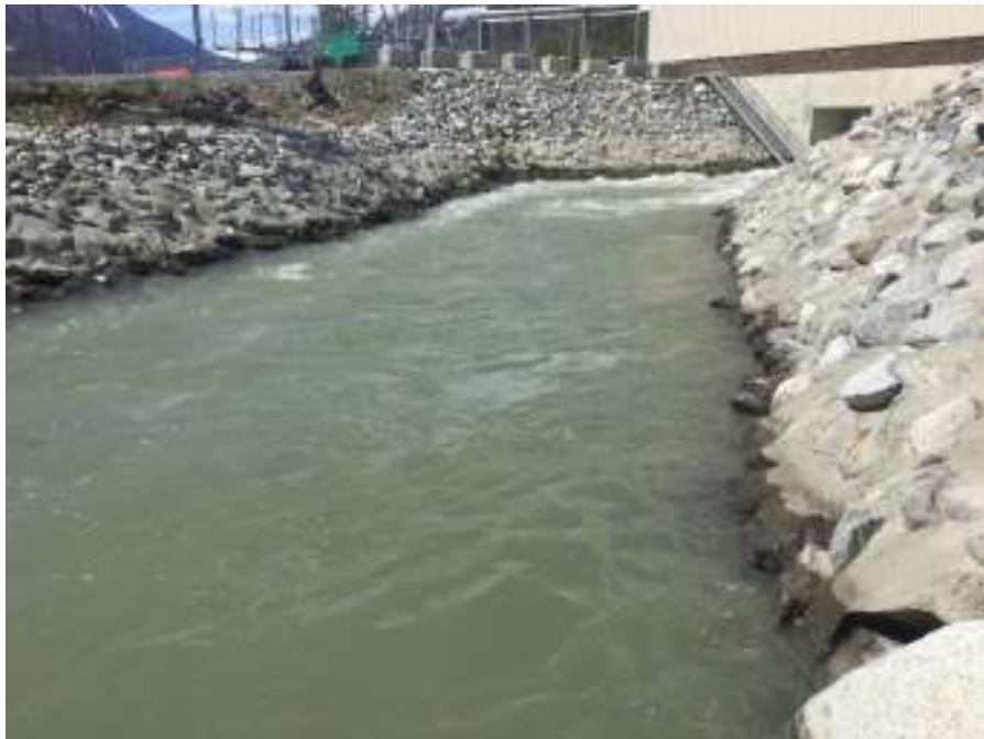
Figure 24. Looking upstream at BDR-TAILWQ on May 12, 2020.
