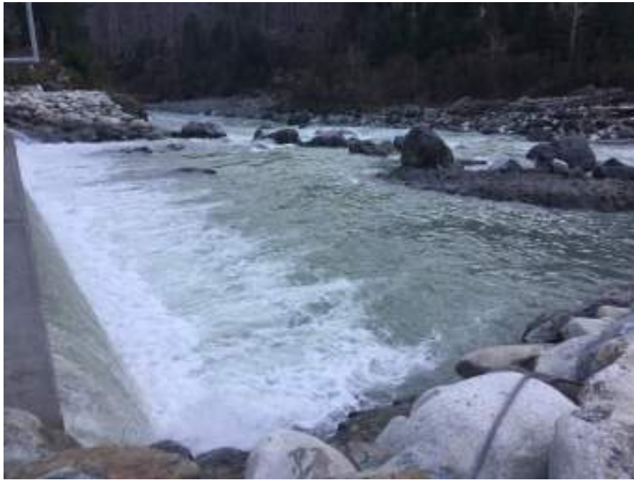
Figure 9. Looking at RR-RL at ULL-TAILWQ on October 22, 2020.
