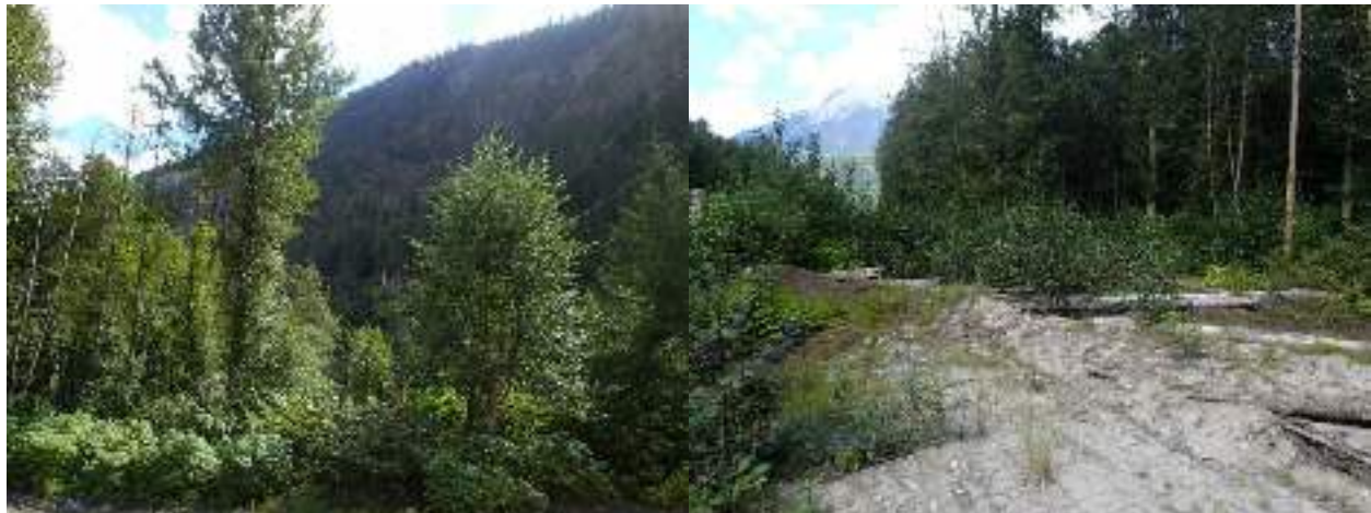
Figure 22. Vegetated screen along the transmission line at ULH-MAMCM14, assessed on August 24, 2020.
