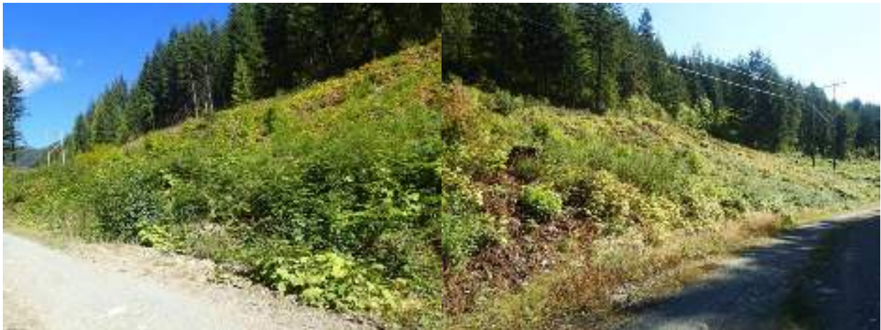
Figure 36. Vegetated screen along the transmission line at ULH-MAMCM23, assessed on August 25, 2020.
