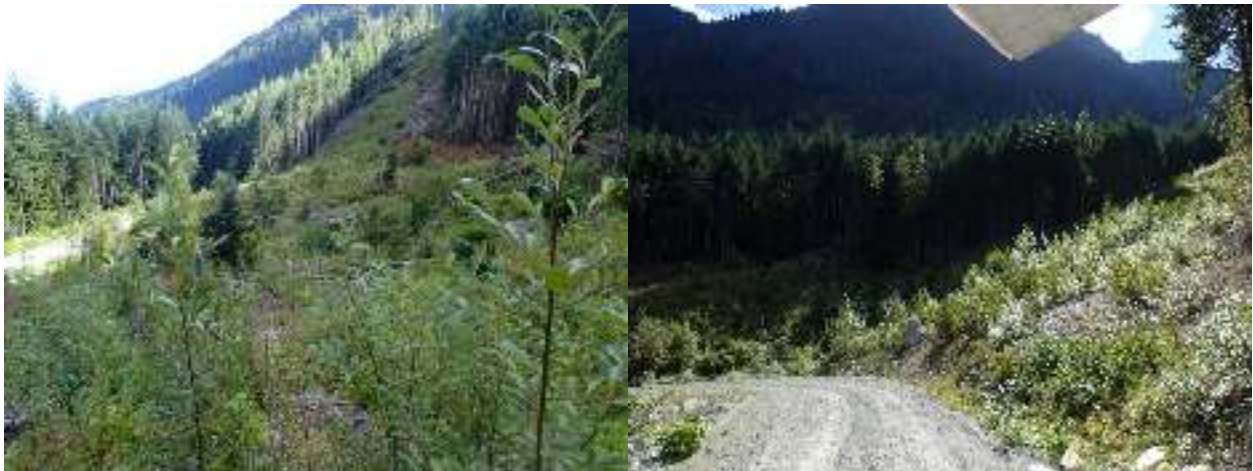
Figure 44. Vegetated screen along the transmission line at ULH-MAMCM27, assessed on August 25, 2020.
