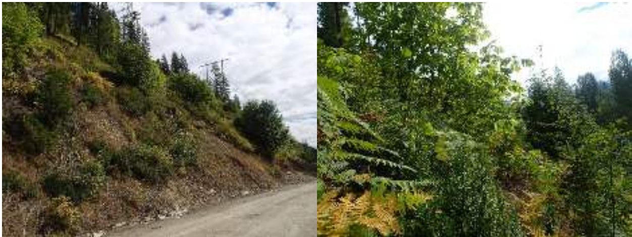
Figure 12. Vegetated screen along the transmission line at ULH-MAMCM08, assessed on August 24, 2020.
