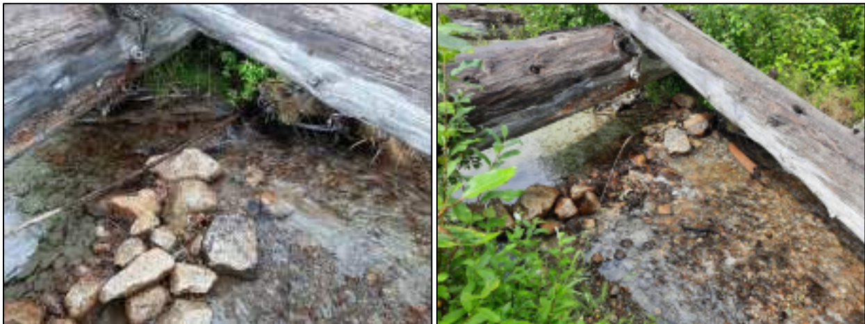
Figure 16. Restored riffle crest above ALE-XS7 before (left) and after (right) repair. Flow is from left to right.
