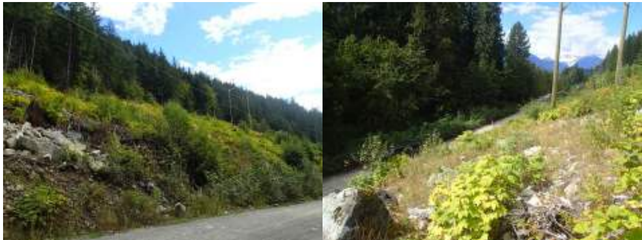
Figure 14. Vegetated screen along the transmission line at ULH-MAMCM09, assessed on August 24, 2020.
