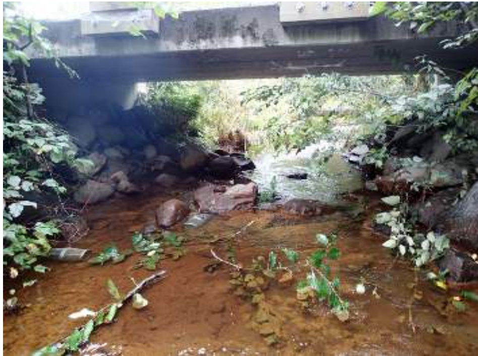
Figure 1. Looking downstream at ALE-BDGWQ on September 21, 2020.
