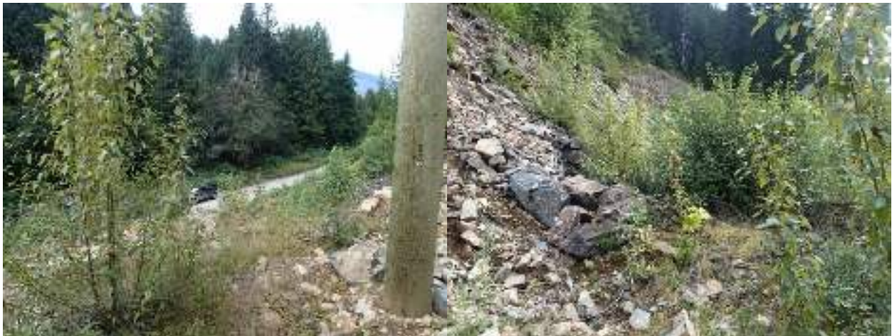
Figure 10. Vegetated screen along the transmission line at ULH-MAMCM07, assessed on August 24, 2020.
