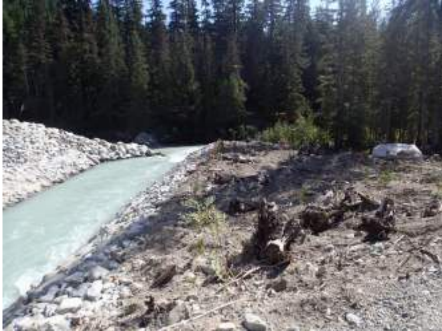
Figure 1. Representative site photo taken at 160° from BDR-PRM01 on September 6, 2018.
