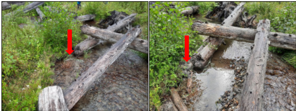
Figure 12. Bank erosion repair and gravel redistribution to create flow deflector near ALE-XS6, before (left) and after (right) repair. Flow is from bottom to top. Flow energy is concentrated away from eroding left bank and towards rootwads on river right.
