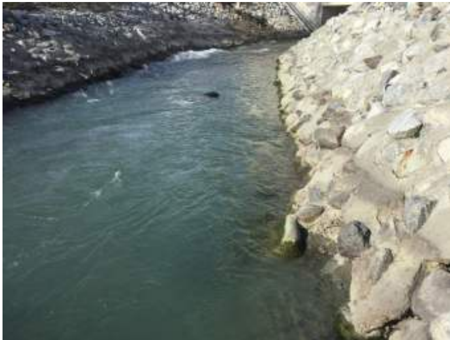
Figure 26. Looking upstream at BDR-TAILWQ on October 22, 2020.
