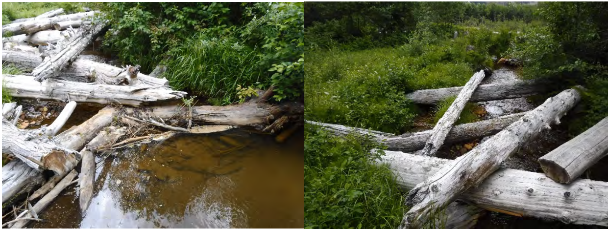
Figure 5. Log that has collapsed between ALE-XS1 and ALE-XS2 (left) causing moderate side-channel formation (right and shown in Figure 1 to Figure 4) and partial backwatering of a riffle. Photos taken on June 20, 2019.
