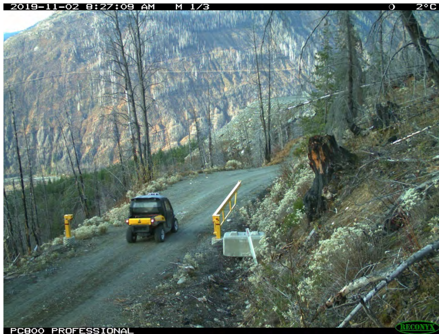
Figure 31. Lock block placed on the upslope side of the gate across the Boulder Creek HEF intake access road (BDR-CAM03) in 2019 to prevent potential motorized access around the gate.
