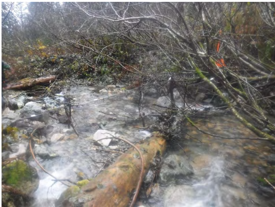
Figure 36. Looking downstream at ULL-HPTB87.0EF03 on October 20, 2019.
