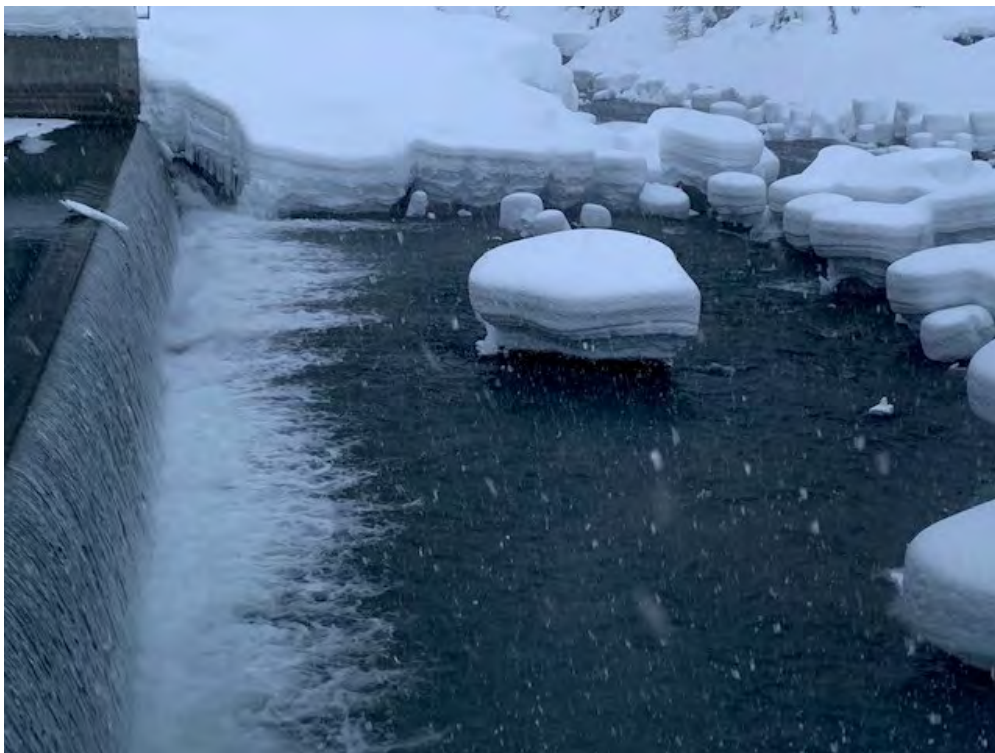
Figure 14. Looking at Upper Lillooet tailrace on January 18, 2020.
