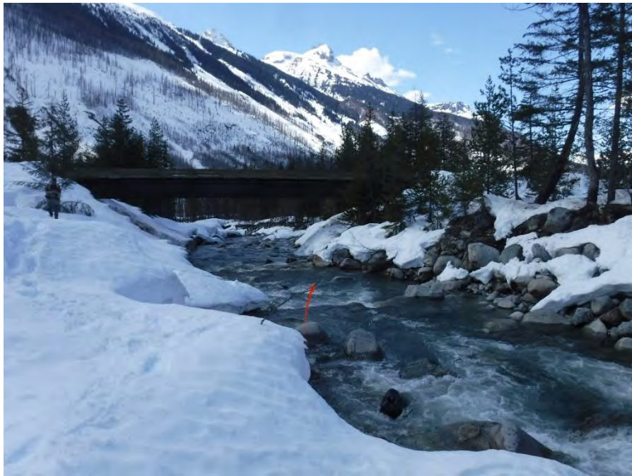
Figure 6. Looking downstream at BDR-DSSN03 on March 30, 2019.
