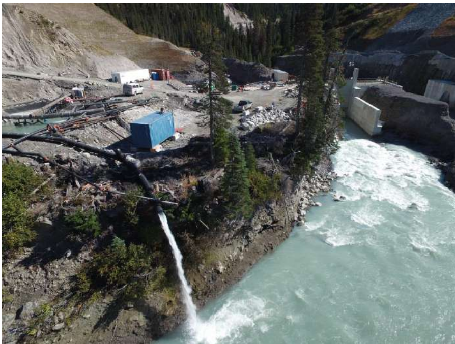
Figure 2. Upper Lillooet River HEF intake during construction, on September 22, 2016.
