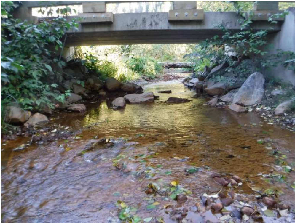
Figure 1. Looking upstream at Unit 1 on October 3, 2017.
