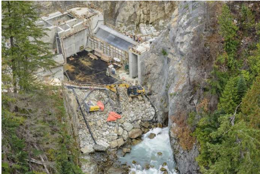
Figure 4. Boulder Creek HEF intake and diversion tunnel under construction, on September 7, 2016.
