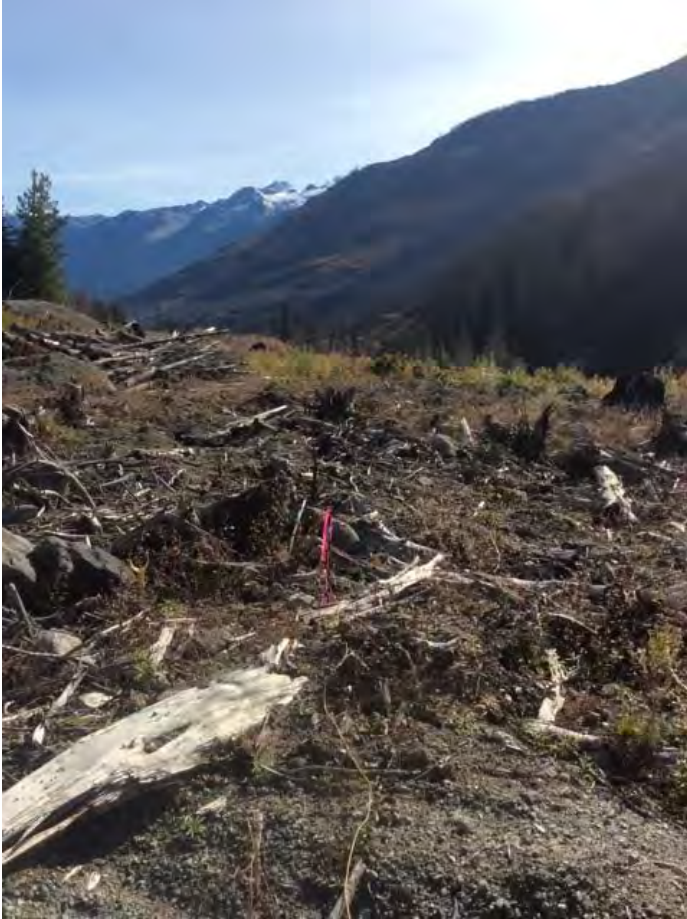
Card: Civil Works Stratum: 41.7km Laydown/Plot: M/Comments Overview photo looks South towards plot center. Sep 26, 2018 02.04.09 PM.jpg
