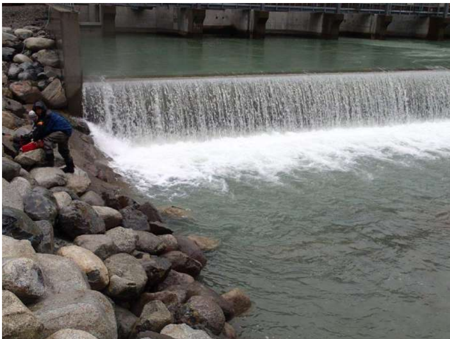
Figure 8. Looking upstream at ULL-TAILWQ on November 1, 2018.
