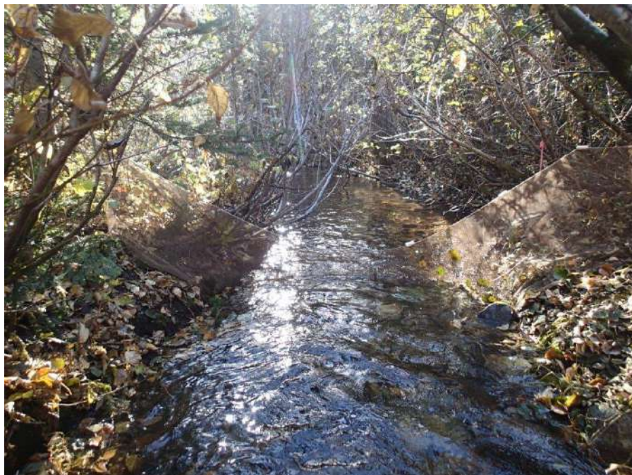
Figure 32. Looking downstream at ULL-HPTB87.0EF03 on October 17, 2018.
