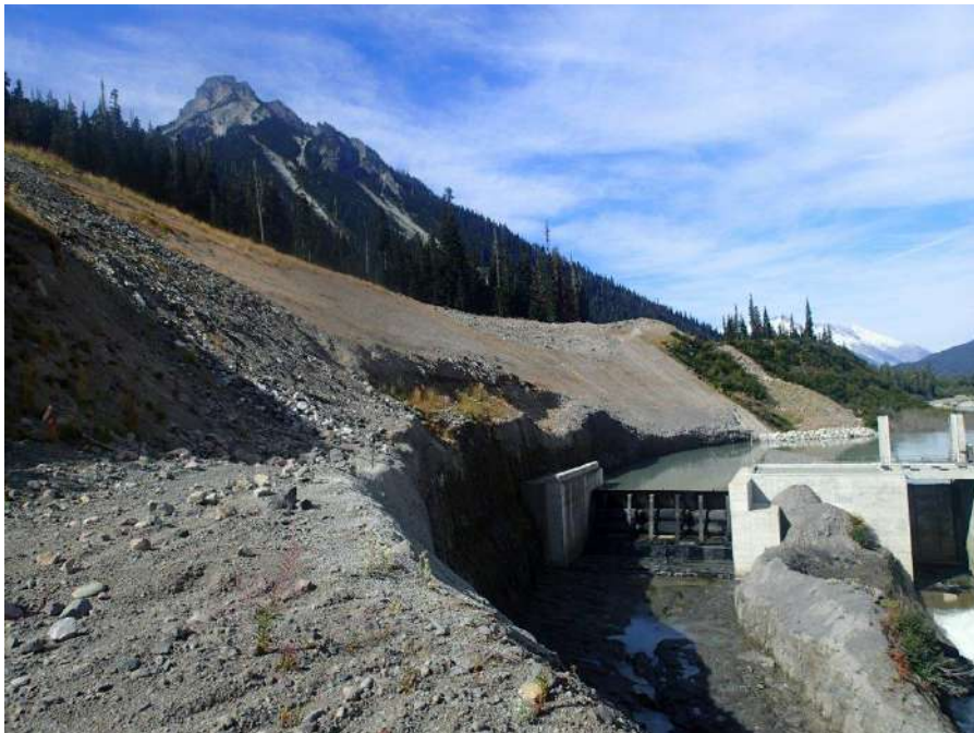
Figure 6. Looking upstream at the dam from ULL-PRM02 on September 7, 2018.
