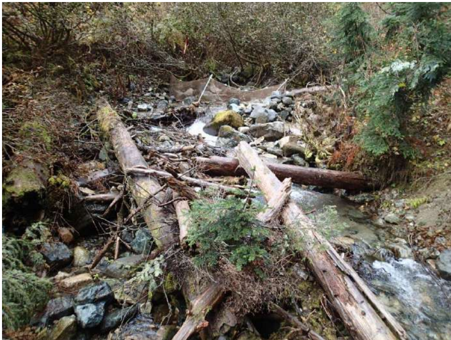
Figure 36. Looking upstream at top of ULL-HPTB87.0EF03 on October 17, 2018.
