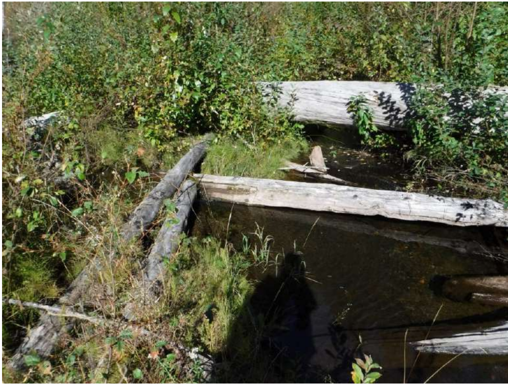
Figure 43. Looking upstream at Unit 21 on October 3, 2017.
