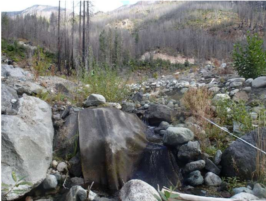
Figure 33. Exposed geotextile within the stream channel at ULL-ASTR04IM on August 31, 2019.
