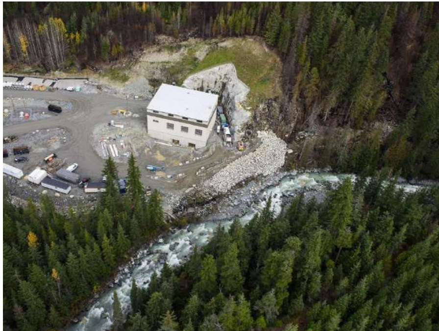
Figure 6. Boulder Creek powerhouse footprint during construction, on March 14, 2016.
