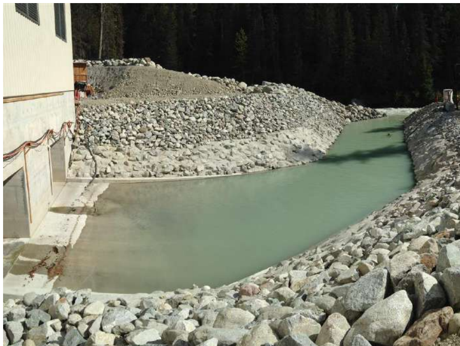
Figure 7. Boulder Creek HEF tailrace in the fall of 2016, after completion.
