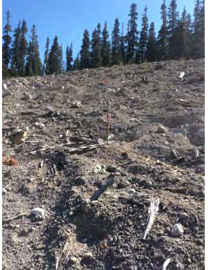
Card: Civil Works Stratum: Diversion Channel Slopes/Plot: 009/Comments Overview photo looks at plot from the North side. Sep 06, 2018 03.00.48 P
