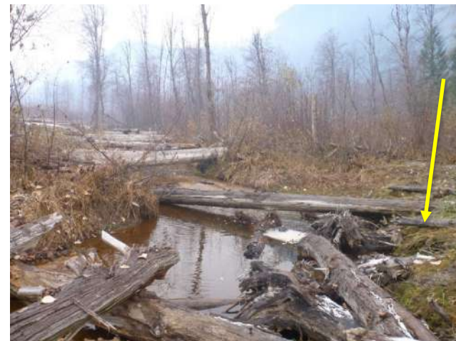
Figure 10. Looking upstream at bend at installed rootwads where bank has eroded on Nov 10, 2017.
