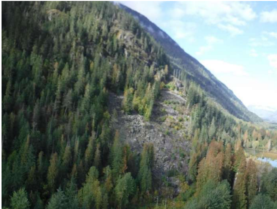
Figure 37. Transmission line below Peregrine Falcon nesting ledges at ULH-PEFACM03, on September 24, 2018. The nearest nesting ledges are approximately 300 m above the transmission line, not visible in this photo.
