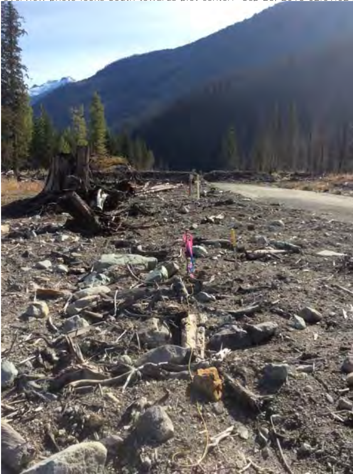
Card: Civil Works Stratum: Upper Lillooet Penstock/Plot: P/Comments Overview photo looks South towards plot center. Sep 26, 2018 02:59:52 P
