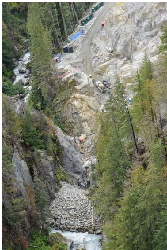
Figure 5. Boulder Creek HEF intake and access road, under construction on September 7, 2016.
