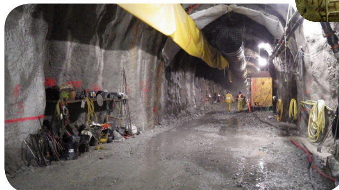
↑ Applying shotcrete to the tunnel face and walls for stability
