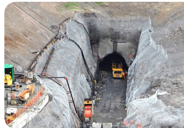
↑ Upper Lillooet Upstream Tunnel Portal
