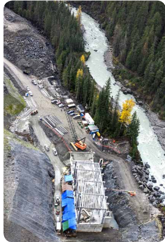
↑ Upper Lillooet River powerhouse structure as of October 2015
