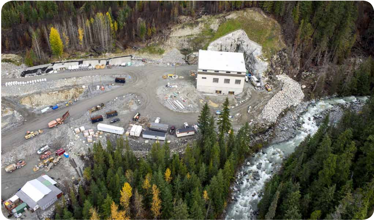
↑ Boulder Creek powerhouse structure completed in Fall 2015
