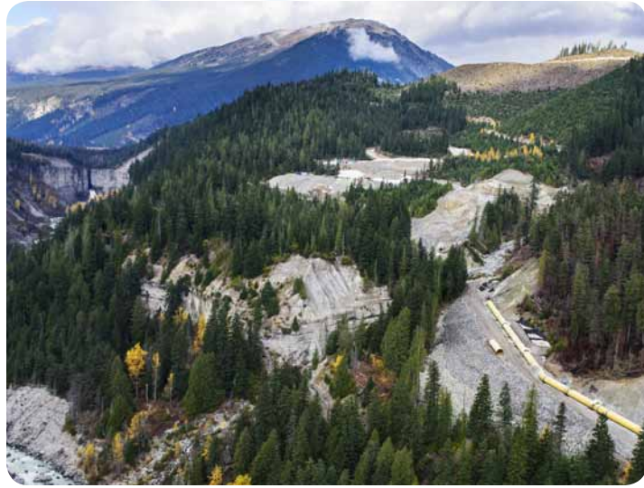
↑ Upper Lillooet River penstock construction now 80% completed
