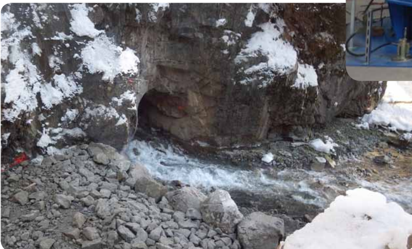
↑ Boulder Creek intake diversion completed
