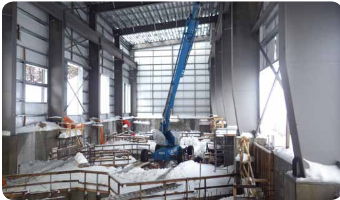
Upper Lillooet River powerhouse roof and cladding near completion →
