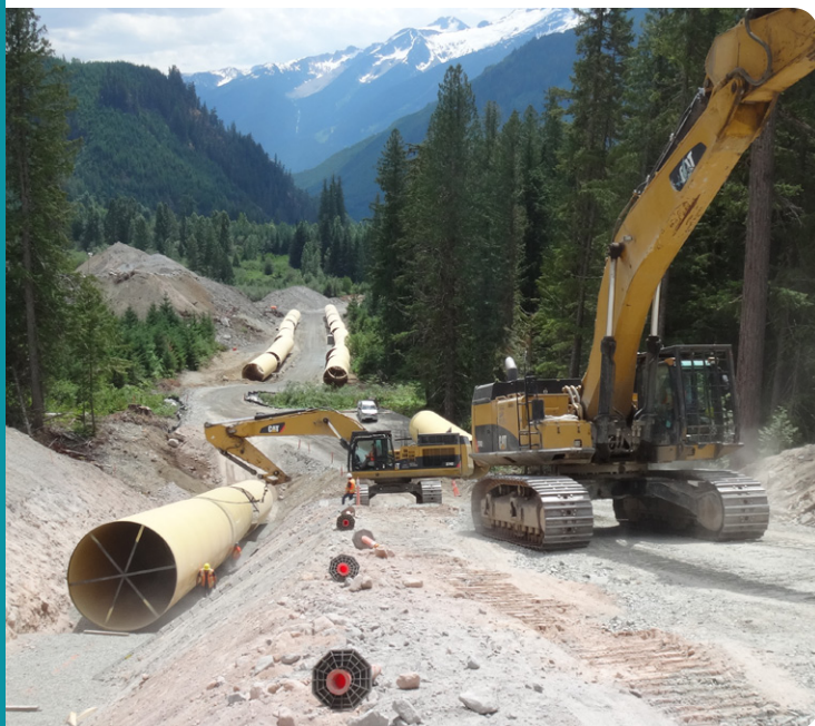
↑ June 29, 2015 - Upper Lillooet Penstock placement in trench.
