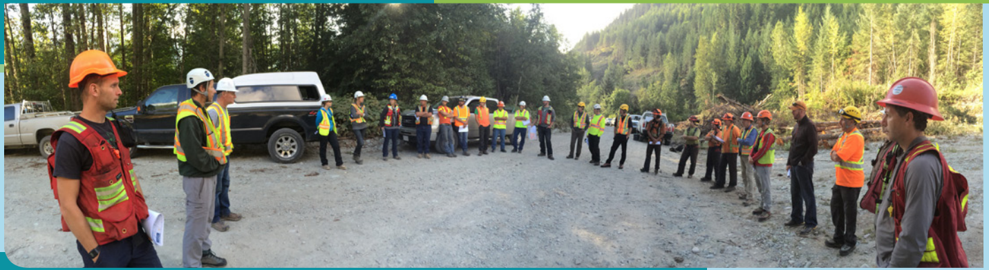
↑ Kick off meeting on site with Hedberg, GMS crew, Westpark, Mumleqs, Innergex and the IEM
