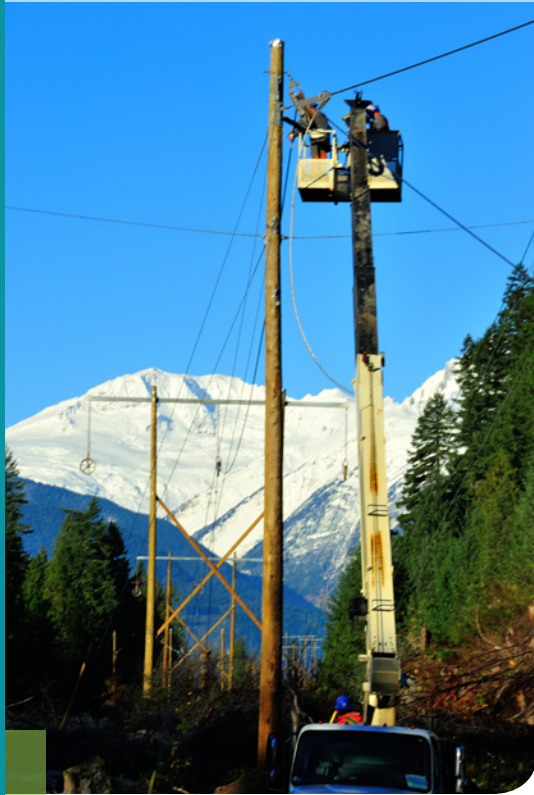
↑ Westpark crew hooking up conductor at top of pole
