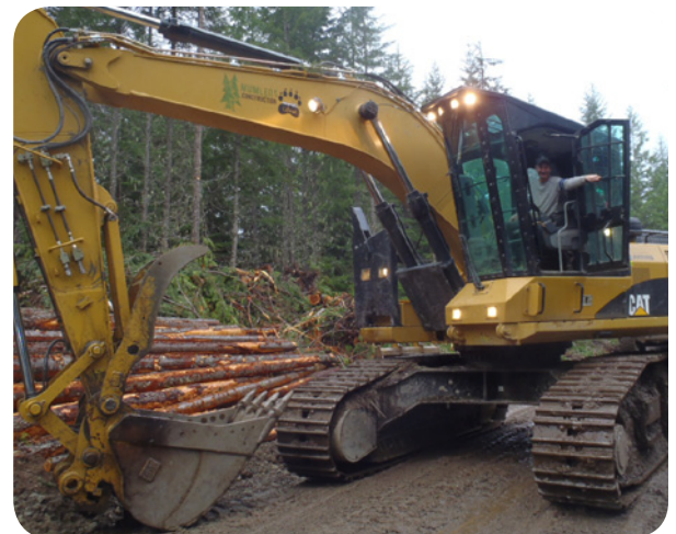
↑ Mumleqs owned excavator at work on the transmission line.
