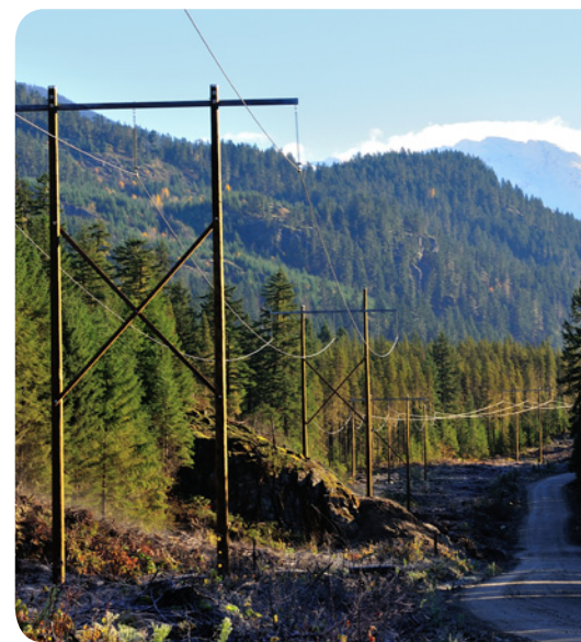
↑ Typical wooden H-pole and completed line
