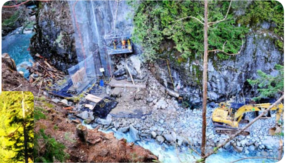
↑ Temporary diversion tunnel works at intake
