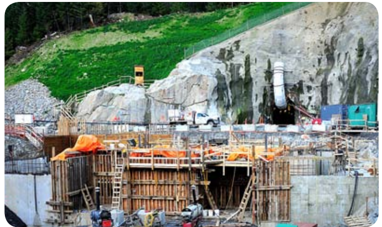
↑ Powerhouse construction and tunnel portal in background
