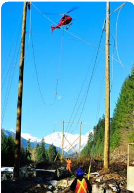
← Helicopter stringer conductor in Segment 5
