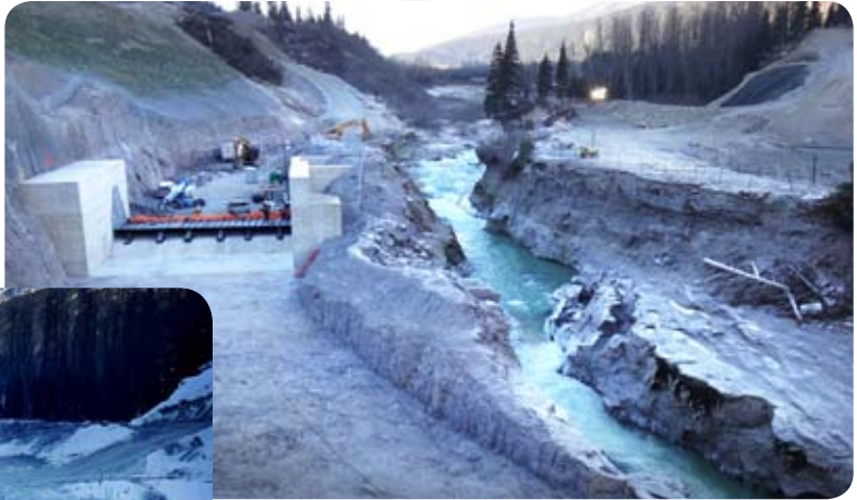
↑ Construction of the Obermeyer Weir in the Diversion Channel
