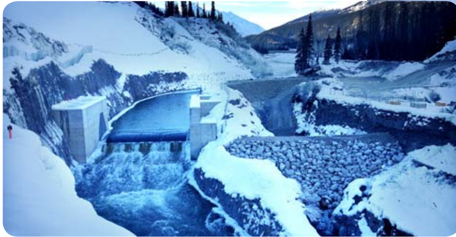
← Upstream and downstream cofferdams in place with Lillooet River flowing into newly constructed diversion channel
