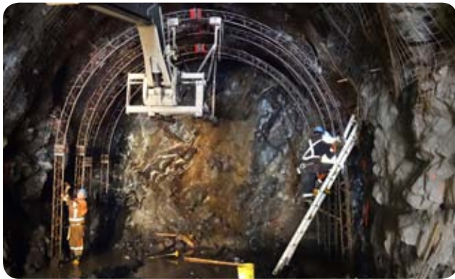
↑ Downstream tunnel support works
