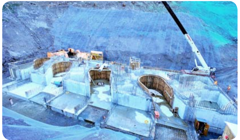
↑ Powerhouse construction as of November
