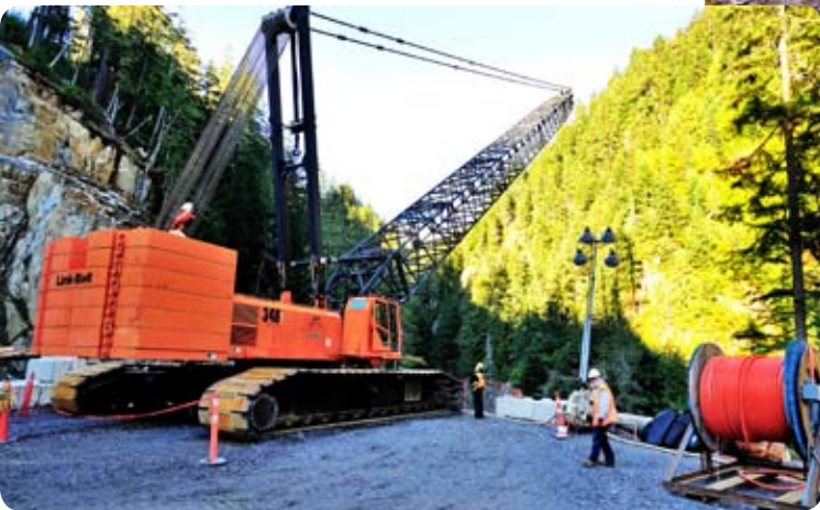
← 300 Tonne Crane at Boulder Intake
