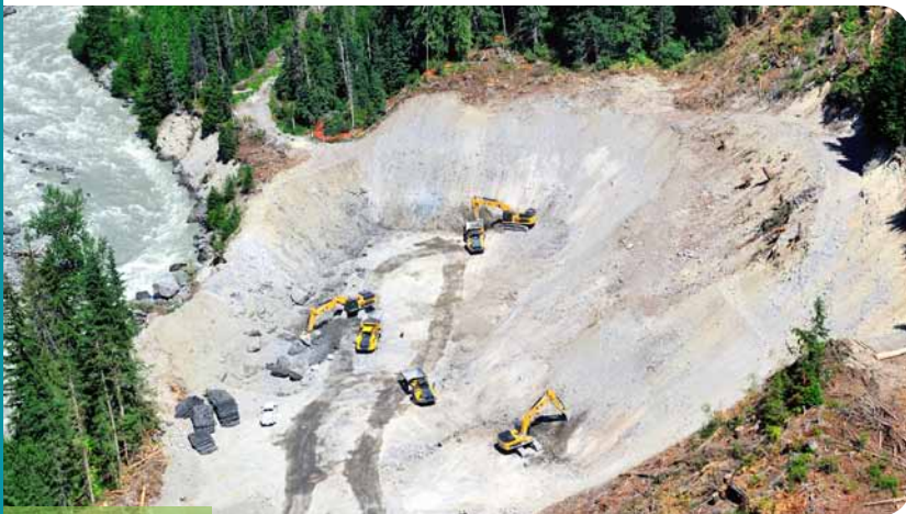
Upper Lillooet River powerhouse excavation site ↑
