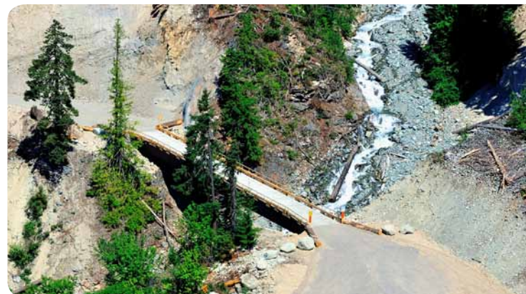
Newly installed bridge over Truckwash Creek ↓
