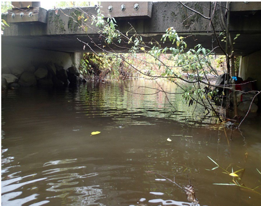
Figure 6. Looking upstream at ALE-BDGWQ on September 27, 2021.
