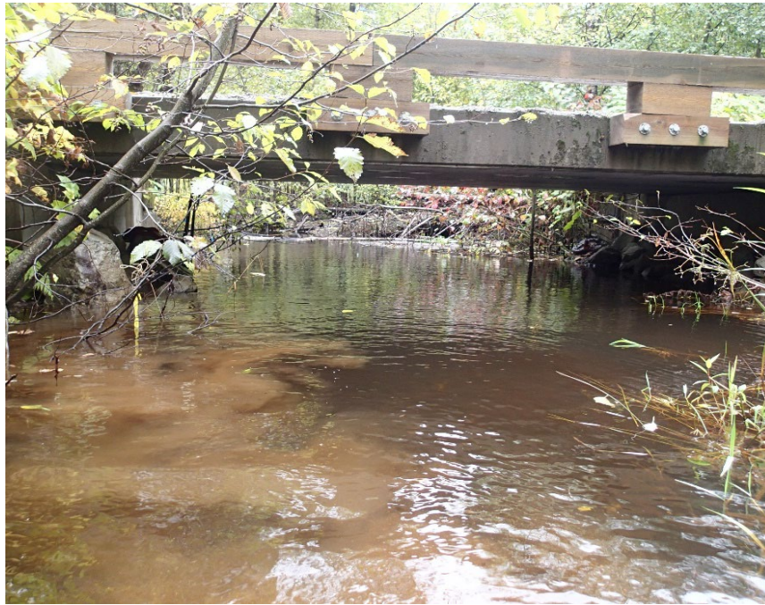
Figure 5. Looking downstream at ALE-BDGWQ on September 27, 2021.
