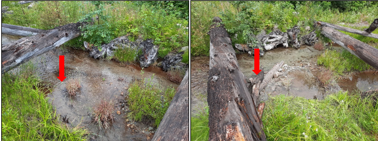
Figure 11. Instream repair near ALE-XS6, before (left) and after (right) repair. Flow is from right to left. Rock/wood flood deflector was installed to scour sand deposited under root wads and to focus flow back into the original channel alignment.
