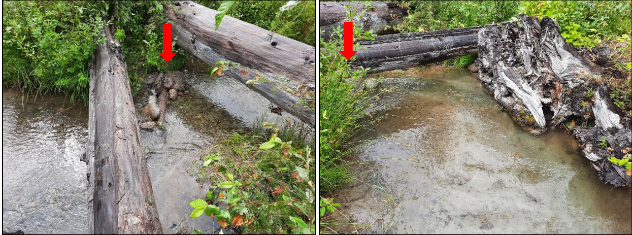
Figure 13. Flow deflector and bank stabilization installed at ALE-XS6, after repair. Flow in left photo is from right to left and arrow shows new deflector. Flow in right photo is from left to right and shows how redirected flow energy has already begun to clean out material deposited at base of root wads.
