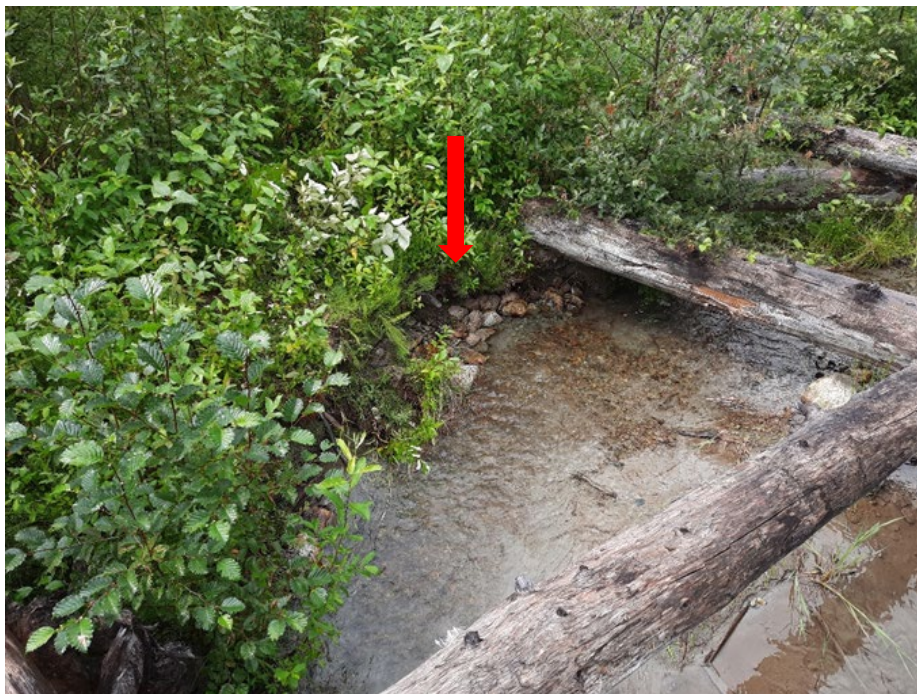
Figure 14. Bank stabilization repairs using cobble above ALE-XS7. Flow is from right to left.
