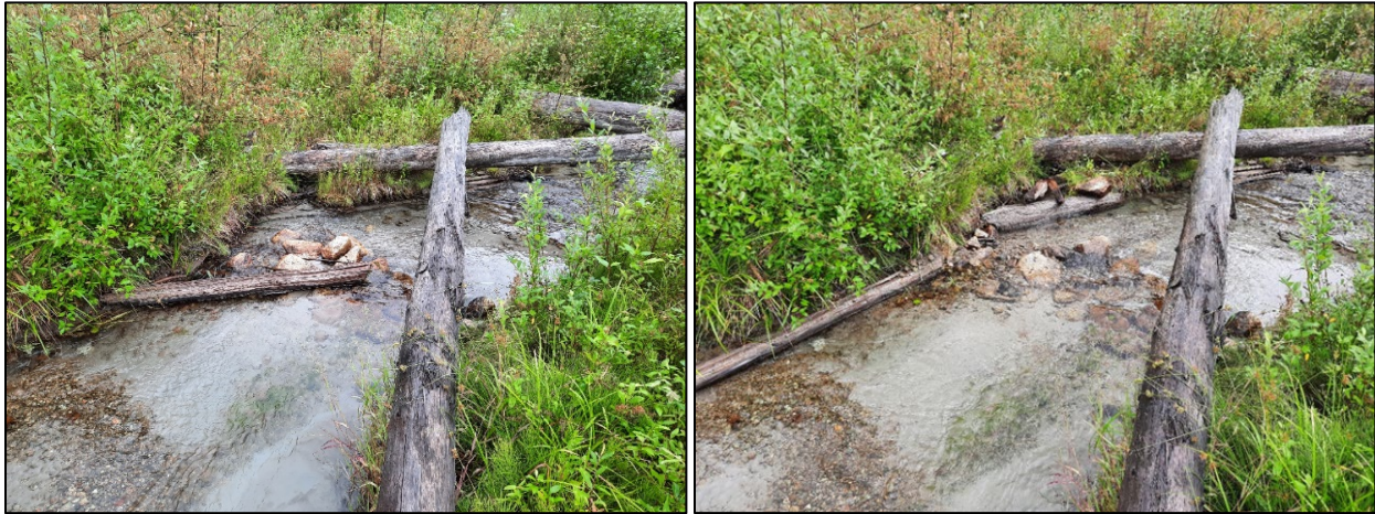
Figure 17. Restored riffle crest and bank protection near ALE-XS8, before (left) and after (right) repair. Flow is from left to right.
