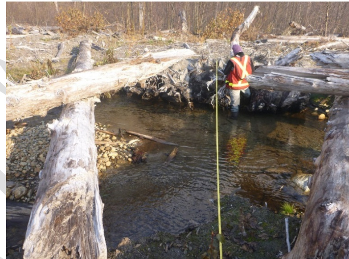
Figure 20. Looking upstream at riffle crest at 0+050 at breach along the RL bank on Nov 10, 2017.
