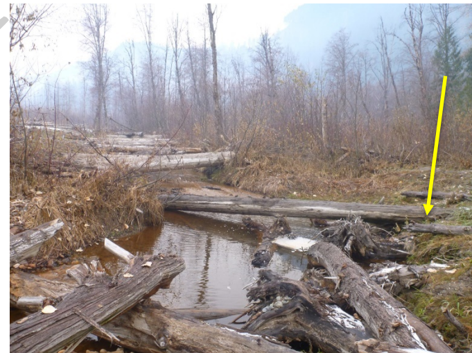
Figure 11. Looking upstream at bend at installed rootwads where bank has eroded on Nov 10, 2017.
