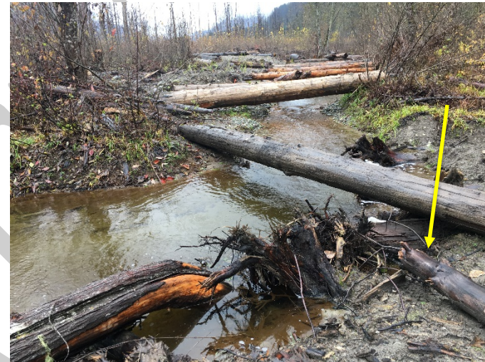
Figure 11. Looking upstream at bend at installed rootwads where bank has eroded on Nov 10, 2017.
