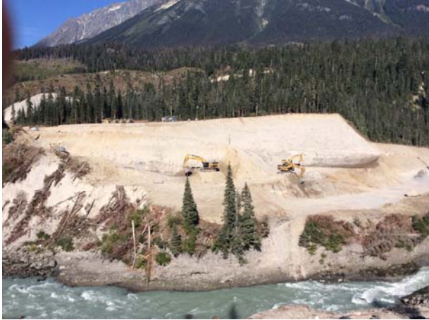
Photo 7 – Bulk excavation (September 11, 2014)
