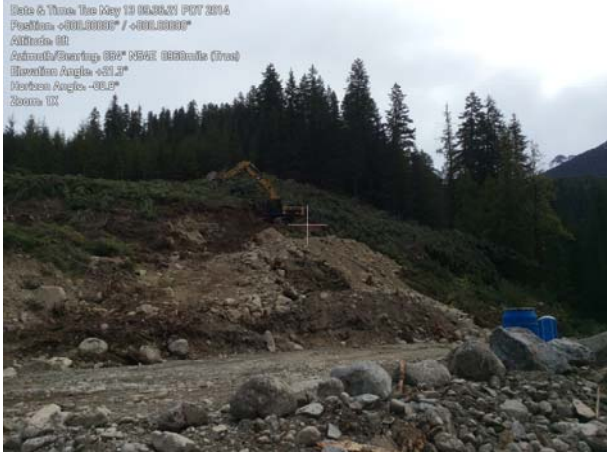
Photo 49 – Clearing the downstream tunnel portal (May 13, 2014)
