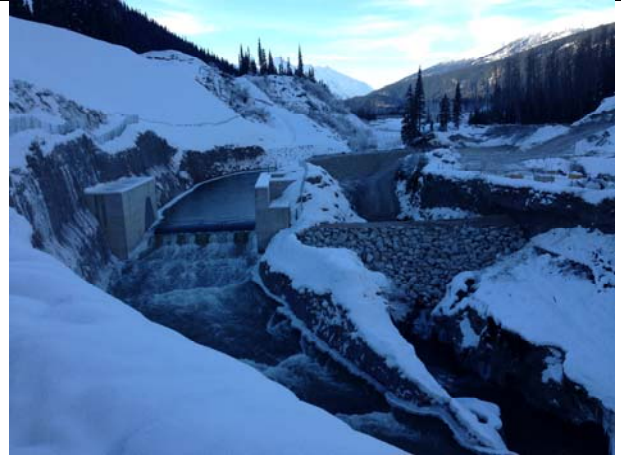
Photo 4 – Intake diversion channel in use (December 2, 2014)
