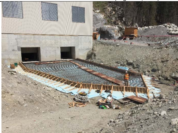
Photo 59 – Construction of Boulder tailrace (May 17, 2016)
