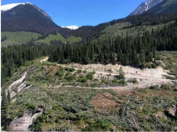
Photo 1 – Clearing river left (June 5, 2014)
