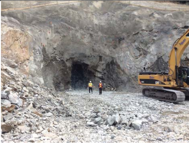
Photo 51 – Beginning of lower tunnel portal excavation (June 24, 2014)
