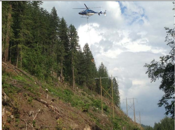
Photo 66 – Stringing conductor in Segment 5 (May 26, 2015)
