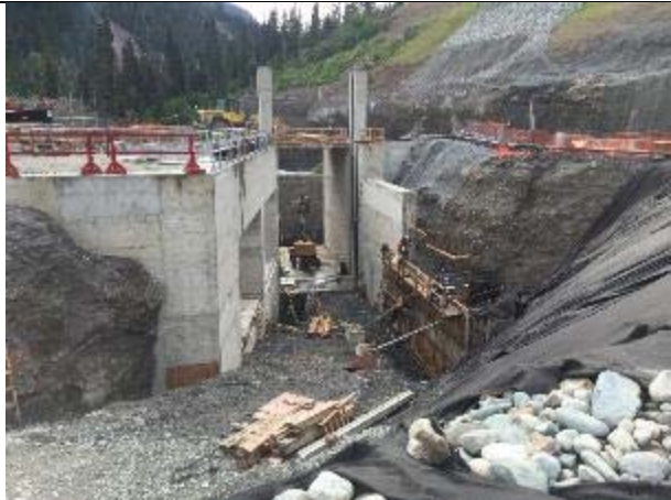
Photo 5 – Intake structure construction (June 14, 2016)
