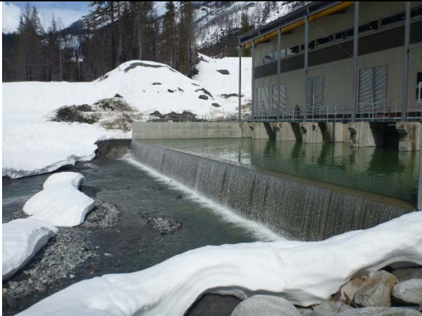
Photo 35 – Tailrace in Operation (April 14, 2017)
