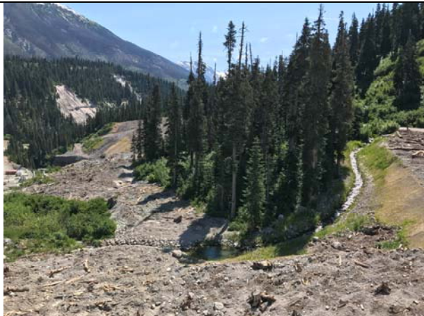
Photo 17 – Final Condition of Right Bank Temporary Work Spaces (July 14, 2017).
