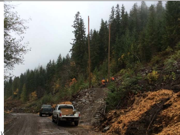
Photo 65 – Setting pole structures in Segment 4 (October 28, 2014)
