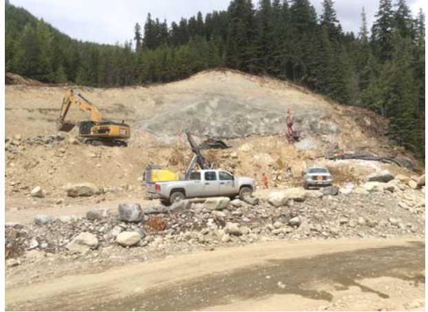
Photo 56 – Bulk excavation of the powerhouse footprint (June 12, 2014)
