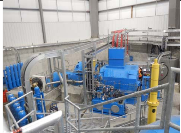
Photo 34 – Inside Completed Powerhouse Structure (March 2, 2017)
