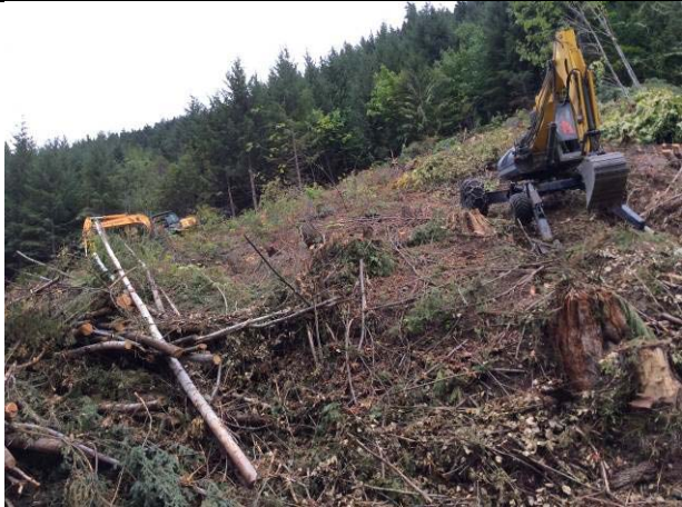
Photo 64 – Excavating pole structure foundations in steep terrain (August 30, 2014)
