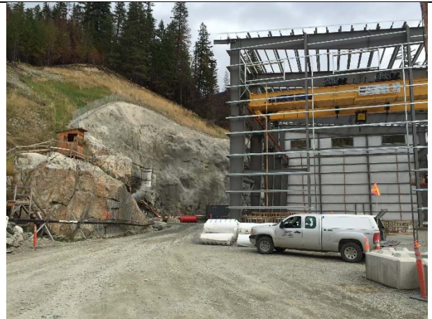
Photo 58 – Powerhouse structure construction (September 7, 2015)
