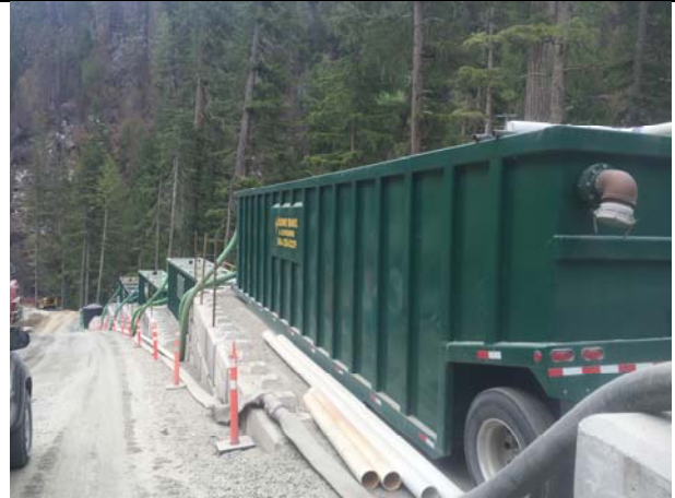
Photo 46 – Dewatering system (May 26, 2016)
