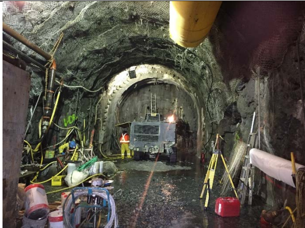
Photo 9 – Active tunneling works (May 10, 2016)
