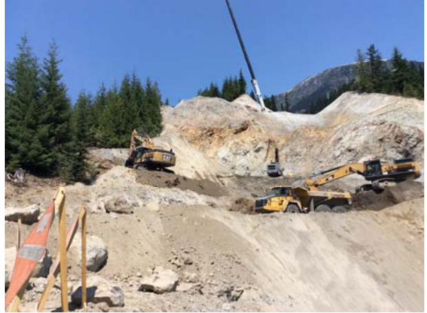
Photo 20 – Bulk Excavation of downstream portal (July 14, 2014)
