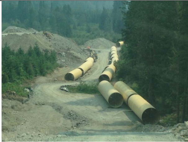
Photo 27 – Penstock staged near ASTR-04 stream crossing (June 16, 2015).
