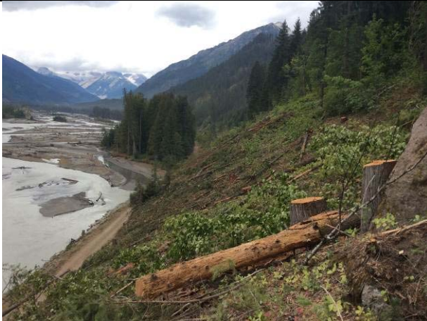
Photo 63 – Hand falling steep areas of the Segment 5 right of way (August 29, 2014)
