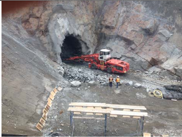
Photo 21 – Start of downstream tunneling and portal consolidation (August 16, 2014)
