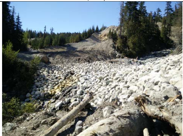
Photo 30 – Truckwash Creek Encased Concrete Penstock Crossing protected with rip-rap (May 20, 2017)
