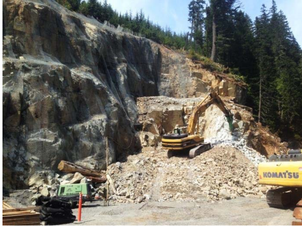
Photo 43 – Start of bulk excavation at the intake access ramp (May 9, 2015)
