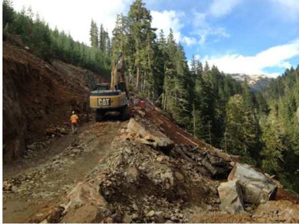
Photo 37 – Clearing and start of bulk excavation (September 25, 2014)
