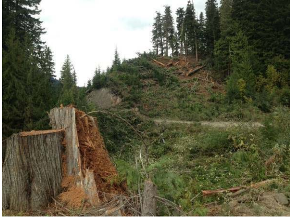
Photo 25 – Penstock right of way clearing (October 1, 2014)
