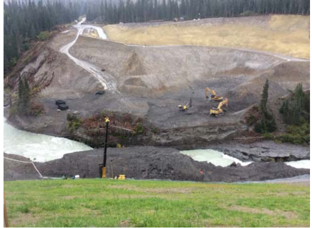
Photo 2 – Bulk excavation river left (September 23, 2014)
