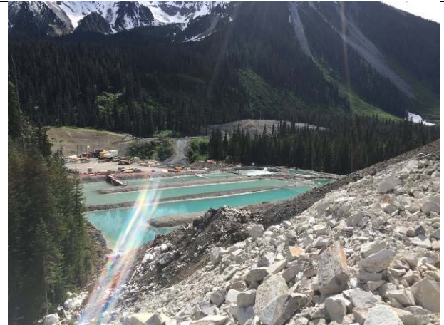
Photo 10 – Dewatering treatment ponds (June 15, 2016)
