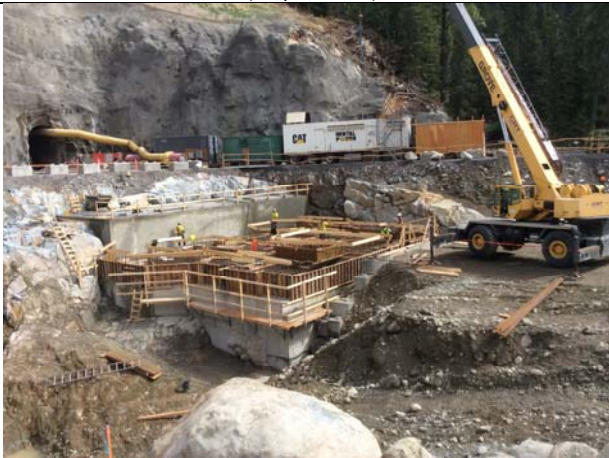
Photo 57 – Powerhouse foundation (August 31, 2014)
