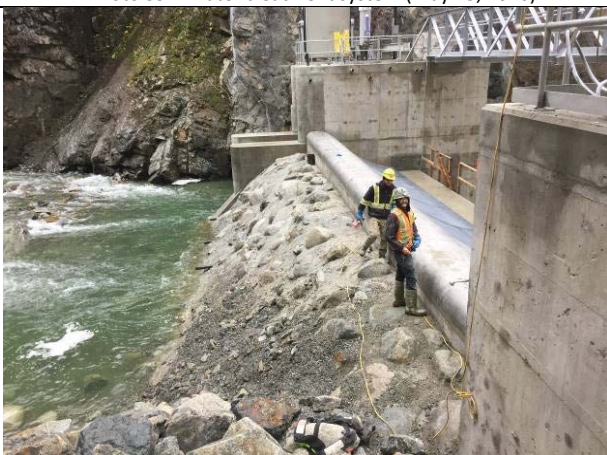
Photo 41 – Final grouting following installation of the Coanda screen (November 5, 2016)
