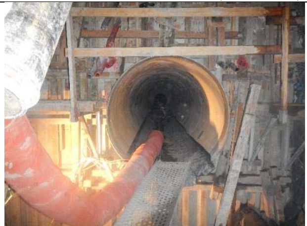
Photo 54 – Steel Liner and Tunnel Plug inside the BDRHEF tunnel (December 9, 2016)
