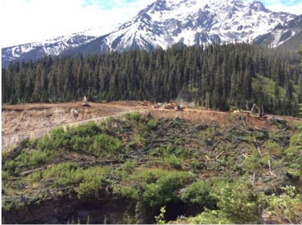
Photo 13 – Clearing right bank (June 6, 2014).
