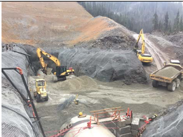
Photo 11 – Buried Concrete Arch Support Installation (October 29, 2016)
