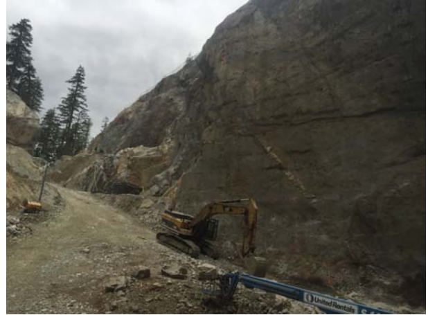
Photo 44 – Bulk Excavation (May 25, 2016)
