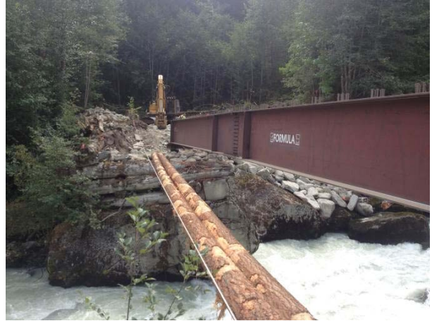
Photo 62 – Installation of the Ryan River clear span bridge (August 16, 2014)
