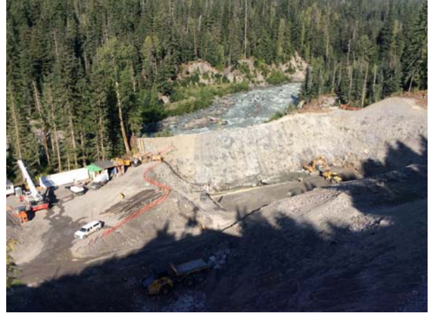
Photo 32 – Bulk excavation of powerhouse footprint (August 26, 2014)
