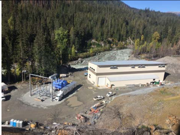
Photo 33 – Completed structure exterior (September 28, 2016)
