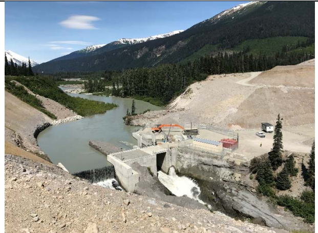
Photo 6 – Overview of the final condition of the intake (July 14, 2017)
