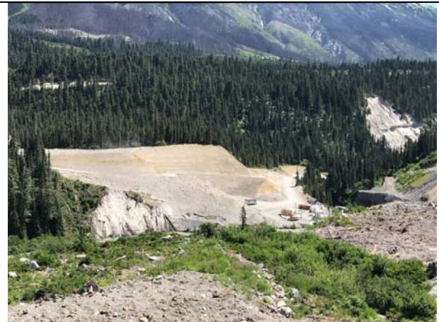
Photo 18 – Final Condition of Left Bank Temporary Work Spaces (July 14, 2017).
