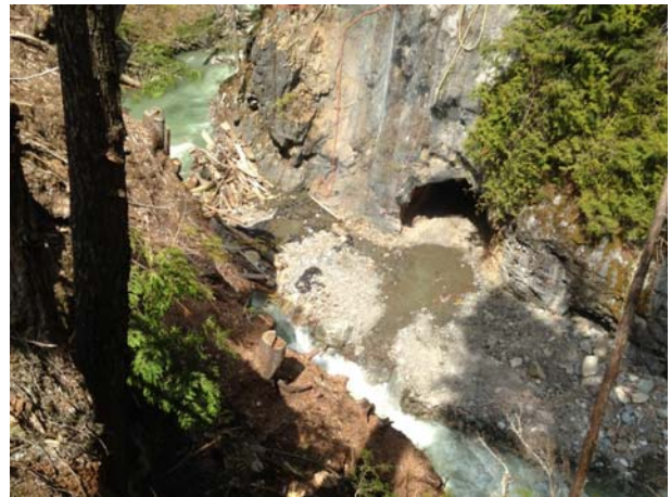
Photo 38 – Excavation of diversion tunnel (May 11, 2015)
