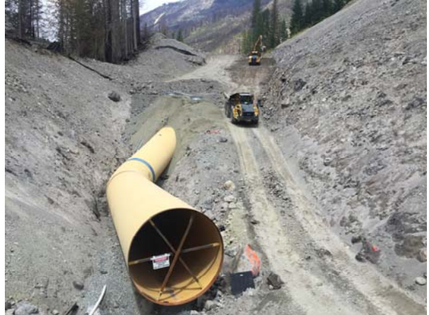
Photo 26 – Fill Placement and penstock installation (June 15, 2016)
