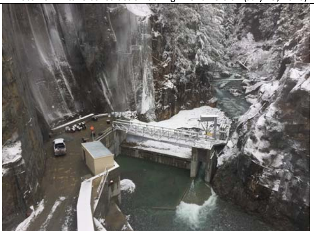
Photo 42 – Completion of intake structure construction (November 11, 2016)
