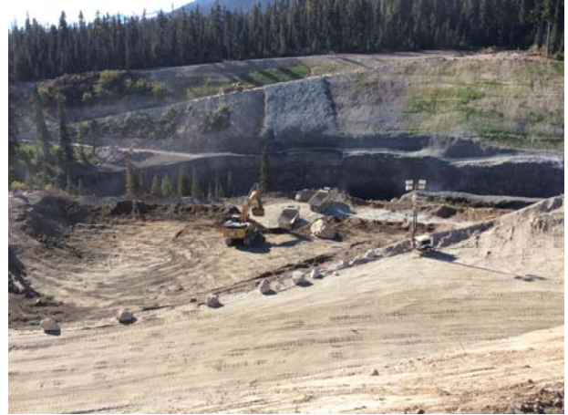
Photo 8 – Bulk Excavation (September 22, 2014)
