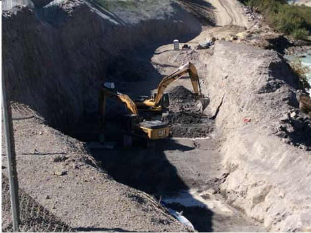
Photo 3 – Diversion Channel Excavation (September 11, 2014)
