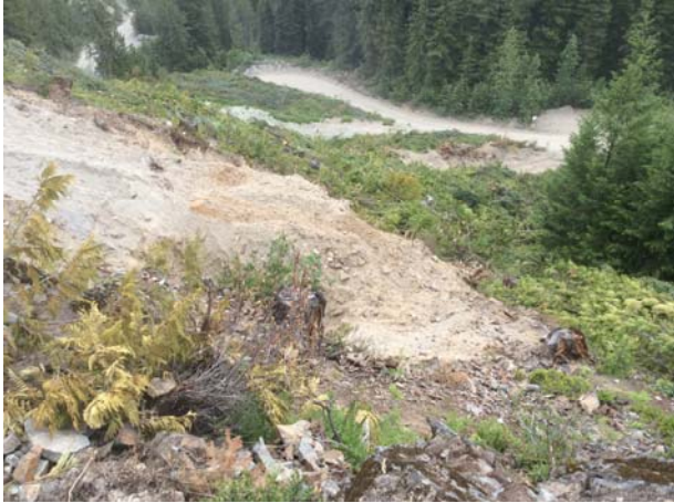
Photo 19 – Clearing and test pit excavation (June 13, 2014)
