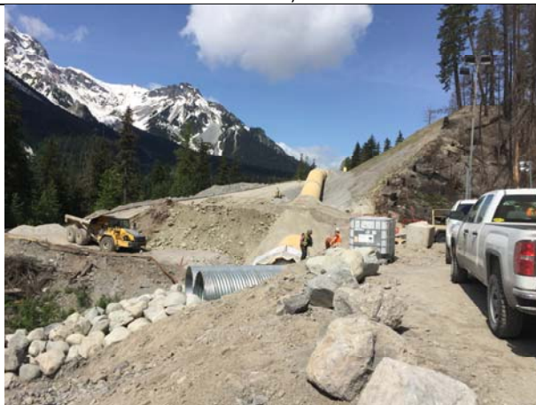
Photo 29 – Stream ASTR-03/ Penstock Overdrain (May 25, 2016)
