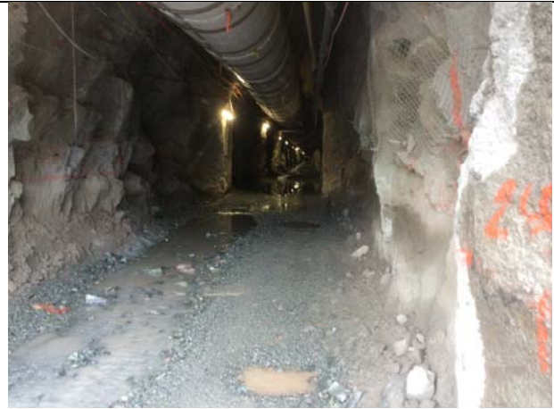
Photo 52 – Entrance to the downstream tunnel (October 16, 2014)
