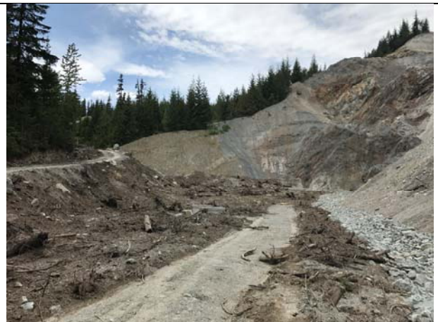
Photo 24 – Final conditions following reclamation (June 22, 2017)
