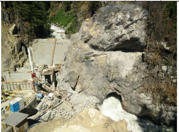
Photo 40 – Intake construction during river diversion (July 29, 2016)
