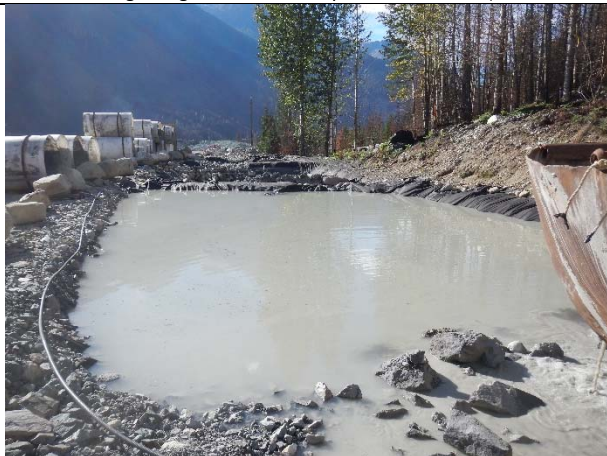
Photo 53 – Boulder downstream tunnel infiltration ponds (September 21, 2015)
