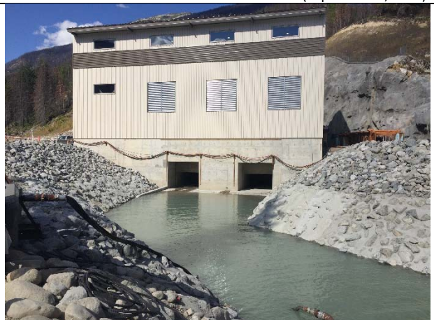
Photo 60 – Completed Boulder powerhouse and tailrace (September 2, 2016)
