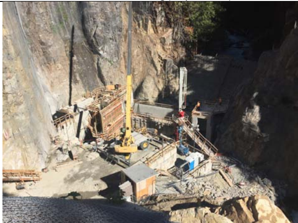
Photo 47 – Regulation chamber and intake structure construction (August 19, 2016)
