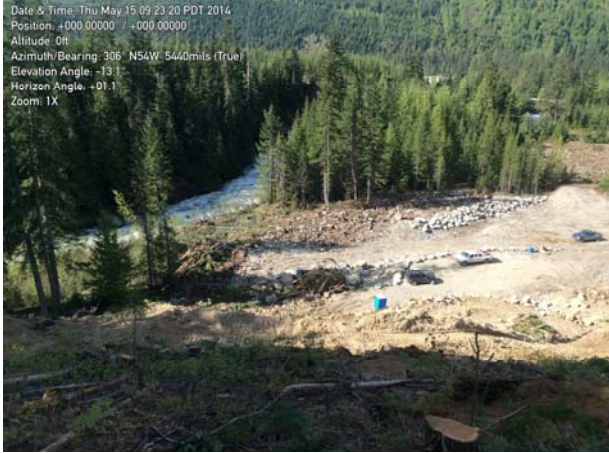
Photo 55 – Clearing footprint for the Boulder Powerhouse and tailrace (May 15, 2014)
