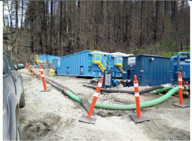
Photo 22 – Dewatering system (May 23, 2016)
