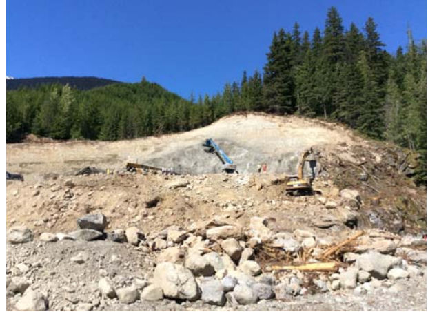
Photo 50 – Bulk Excavation and Slope Stabilization (June 5, 2014)
