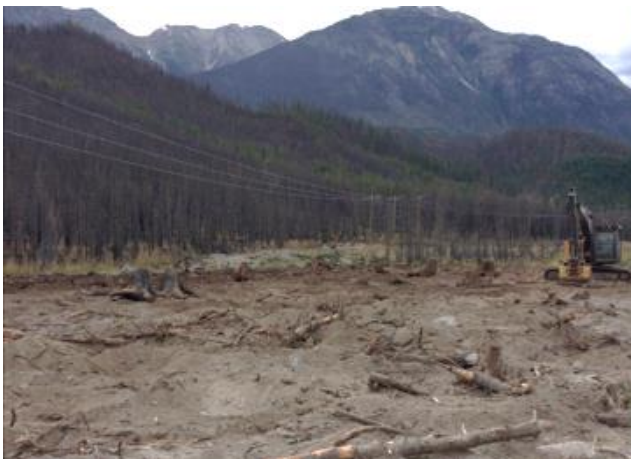
Photo 12 – Final reclamation of the KM39.5 laydown (September 2, 2017)
