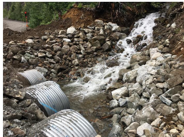
Photo 2 – Completed excavation and rock armouring of the KM41.2 culvert inlets (June 2, 2017).
