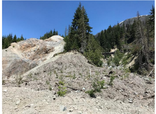
Photo 6 – Final condition of the ULRHEF downstream tunnel portal and Truckwash Creek Mountain goat migration corridor and riparian area (July 14, 2017).
