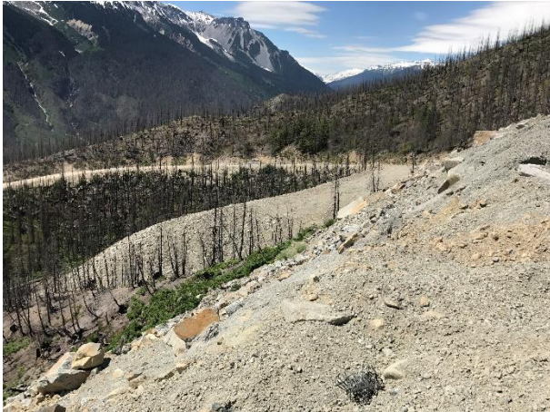
Photo 9 – Final condition of the two main BDRHEF intake spoil areas. Alder seed has been spread (July 14, 2017).
