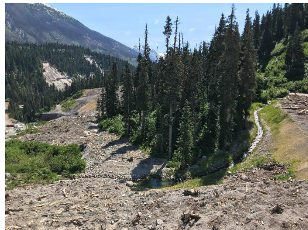
Photo 4 – Overview of the final condition of the ULRHEF intake river right area (July 14, 2017).
