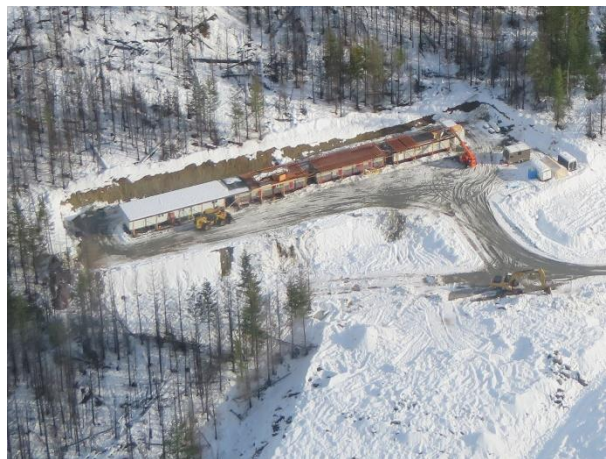
Photo 13 – Completed residence (November 16, 2017).
