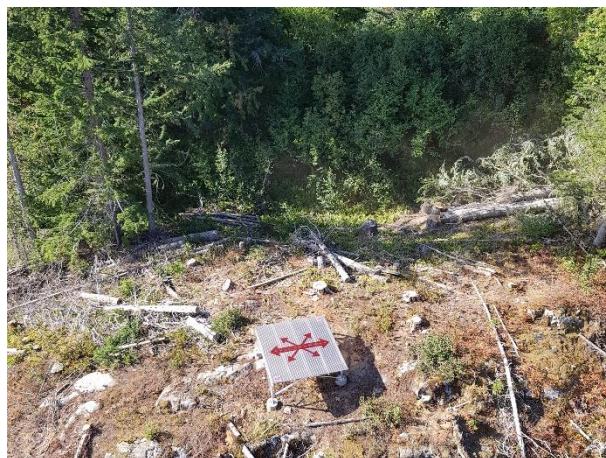
Photo 22 – Helipad H376 final condition (September 15, 2017).
