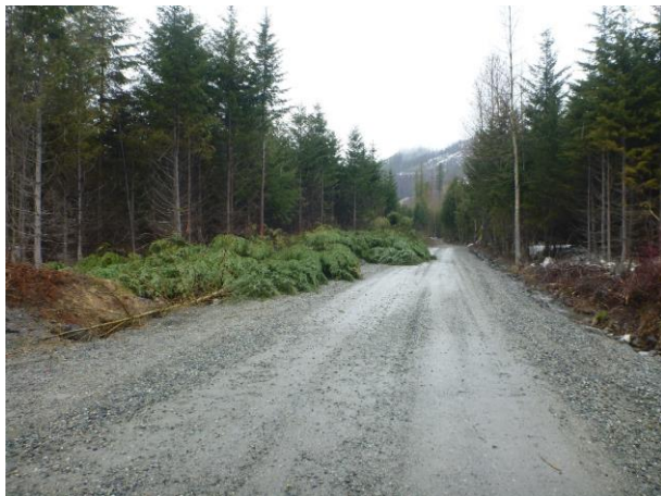
Photo 3 – Tree clearing at KM42 for road widening and raising (May 1, 2017).
