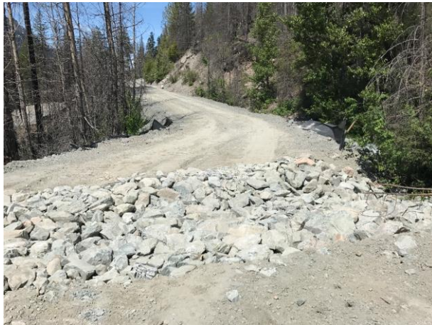
Photo 7 – Deactivated Truckwash 2 access road (May 29, 2017).
