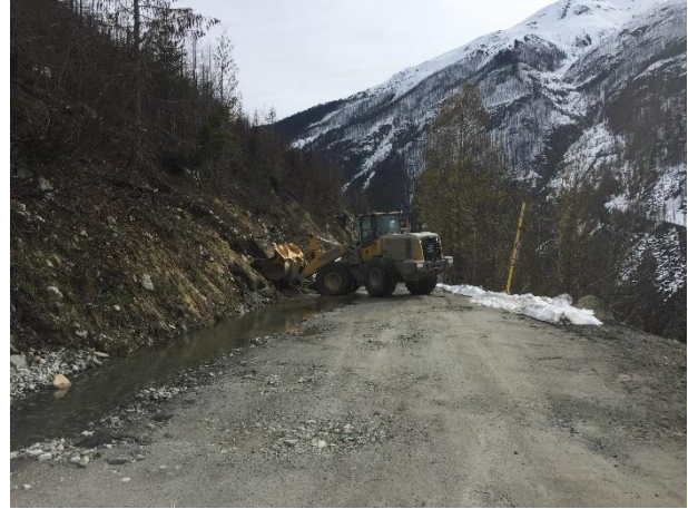
Photo 11 – Ditch maintenance on the BDRHEF intake access road (May 9, 2017)
