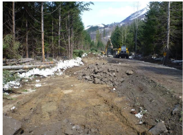
Photo 4 – Grubbing for road widening at KM42 (May 3, 2017).
