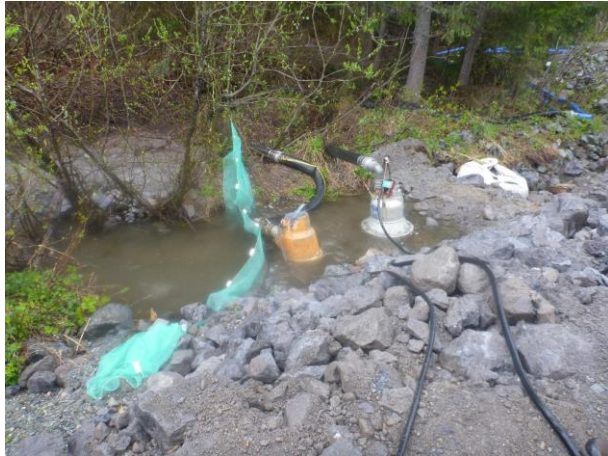
Photo 5 – Ditch isolation and pump around at KM42 (May 12, 2017).
