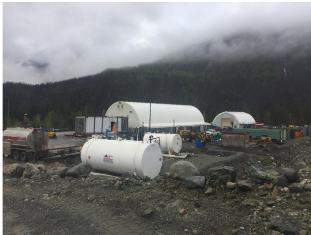
Photo 1 – Mechanics shop and KM38 laydown (May 8, 2017).
