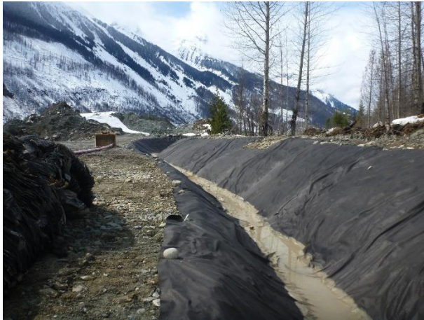
Photo 15 – Drainage and final grading around the BDRHEF powerhouse (April 14, 2017)
