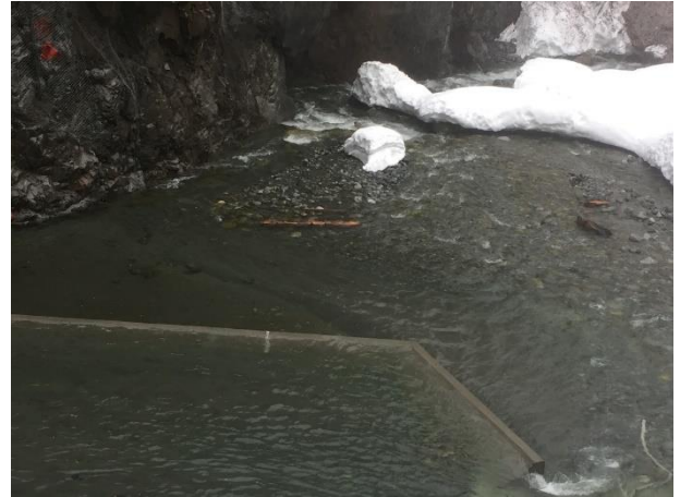
Photo 14 – Sand from the regulation chamber deposited directly downstream of the BDRHEF intake (April 18, 2017)
