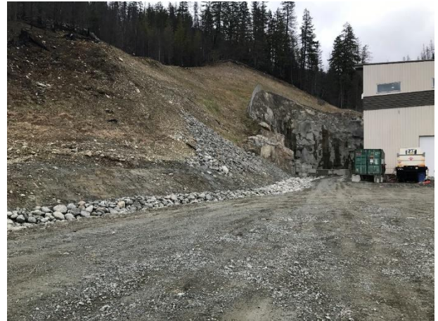
Photo 16 – Completed drainage at the BDRHEF powerhouse (April 26, 2017)
