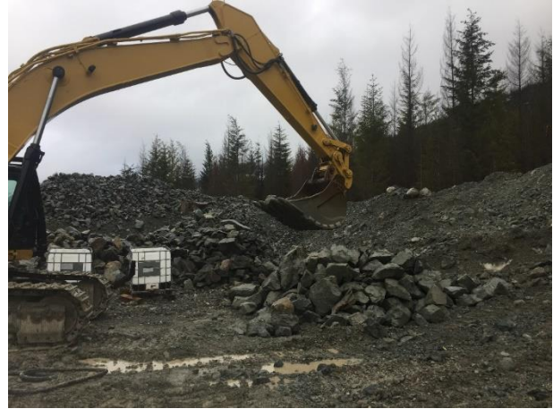
Photo 2 – CE washing BDRHEF tunnel rock at KM38 (April 18, 2017)
