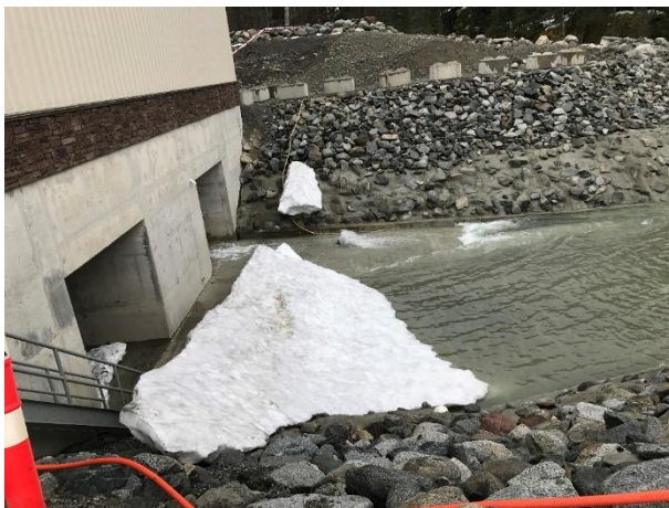
Photo 17 – First flush of water through the BDRHEF generating equipment (April 26, 2017)
