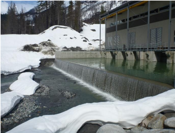
Photo 8 – Current conditions at the ULRHEF powerhouse (April 14, 2017)
