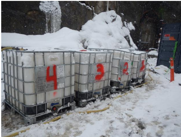
Photo 8 – 1000L totes used to store flushing water until water quality results were received (March 11, 2017).
