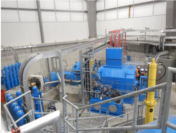
Photo 4 – Condition of the ULRHEF powerhouse during the first water release (March 2, 2017).
