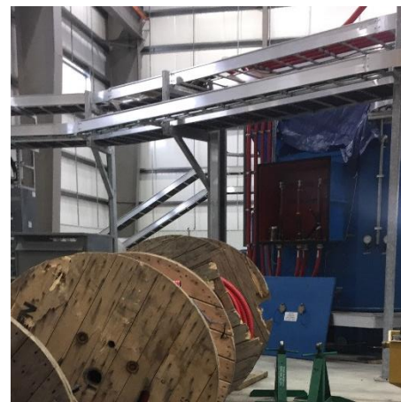
Photo 11 – BDRHEF powerhouse electrical works (March 30, 2017).
