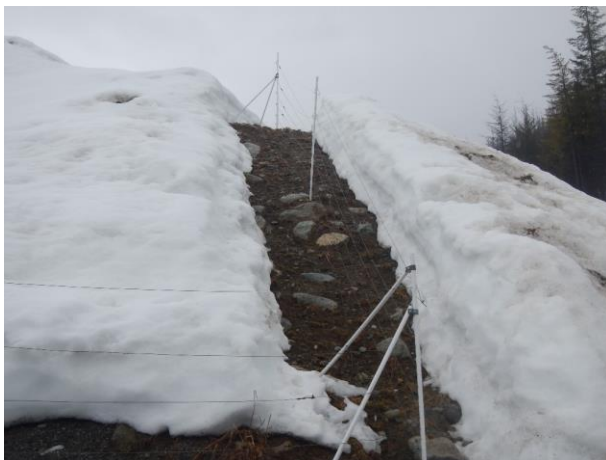
Photo 3 – Maintenance and snow removal around the construction camp electric fence (March 22, 2017).
