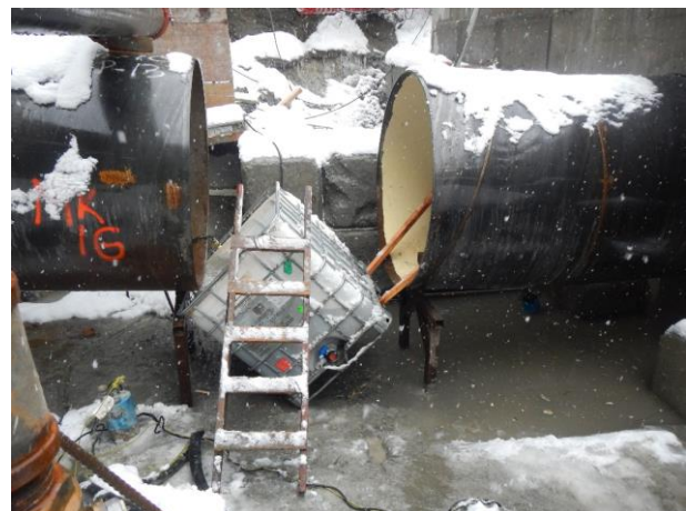
Photo 7 – 1000L tote with a 2" pump used to capture all flushing water (March 11, 2017).
