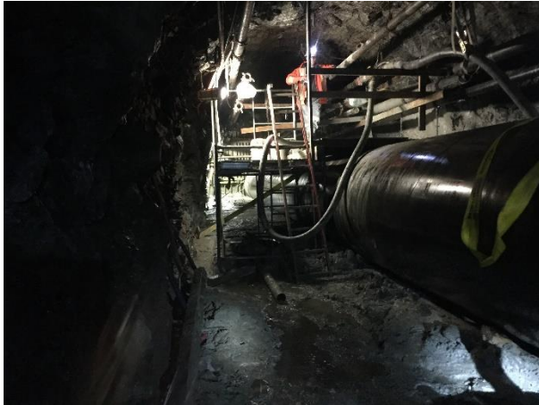
Photo 13 – Cellular concrete injection to encase the BDRHEF steel tunnel liner (February 23, 2017).
