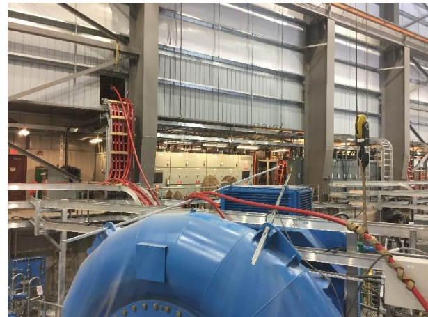
Photo 10 – Electrical works within the ULRHEF powerhouse (February 14, 2017).
