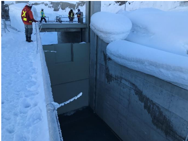
Photo 5 – Lowering sluice gate in a stepwise manner during headpond filling (February 2, 2017)
