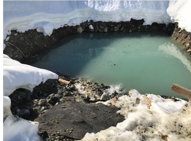
Photo 14 – Process water from the BDRHEF tunnel continues to infiltrate to ground within the infiltration ponds (February 23, 2017).
