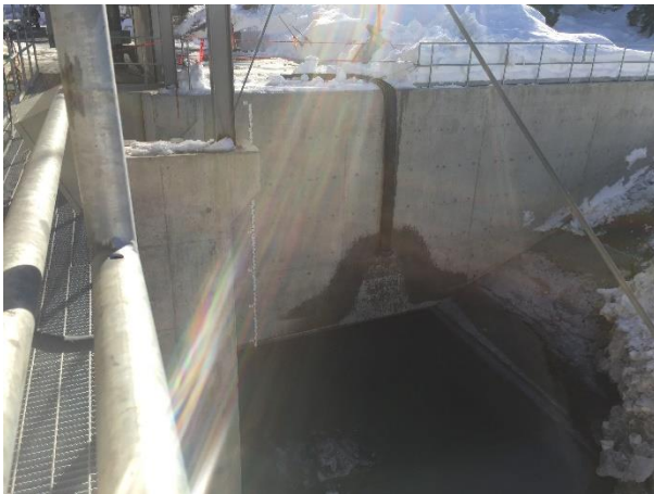
Photo 9 – Filling the tailrace with water from the powerhouse dewatering sump (February 23, 2017).
