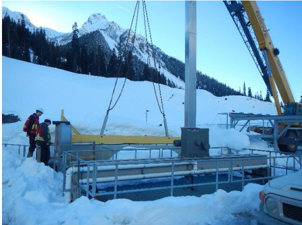
Photo 7 – Waterway filling began by slowly removing stop logs (February 23, 2017)
