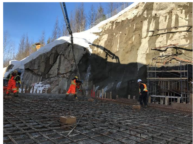
Photo 12 – Pouring concrete for bifurcation encasement at the BDRHEF tunnel portal (February 23, 2017).
