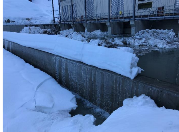
Photo 8 – Tailrace filled as part of waterway filling procedure (February 27, 2017).
