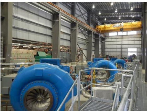
Photo 18 – Current conditions of the ULRHEF Powerhouse (December 11, 2016).
