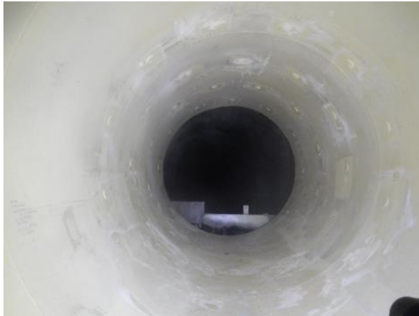
Photo 12 – Completed penstock repair (December 15, 2016).
