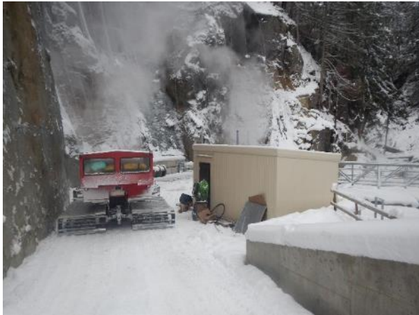
Photo 20 – Commissioning works at BDRHEF intake (December 10, 2016).
