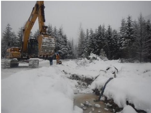
Photo 5 – Removal of PAG spoil pile culvert at KM41.7 (December 10, 2016).
