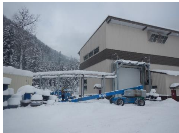
Photo 19 – Switchyard works (December 19, 2016).
