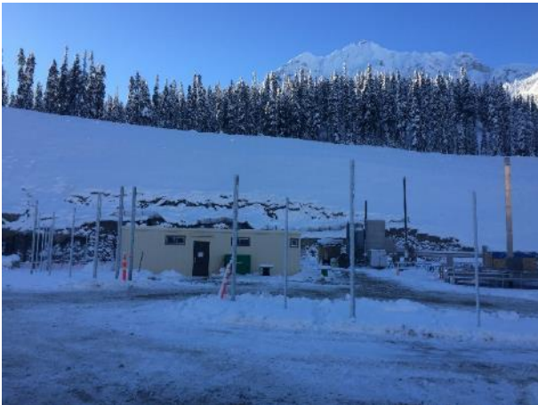
Photo 9 – Pole installation in preparation for perimeter fence (December 6, 2016).
