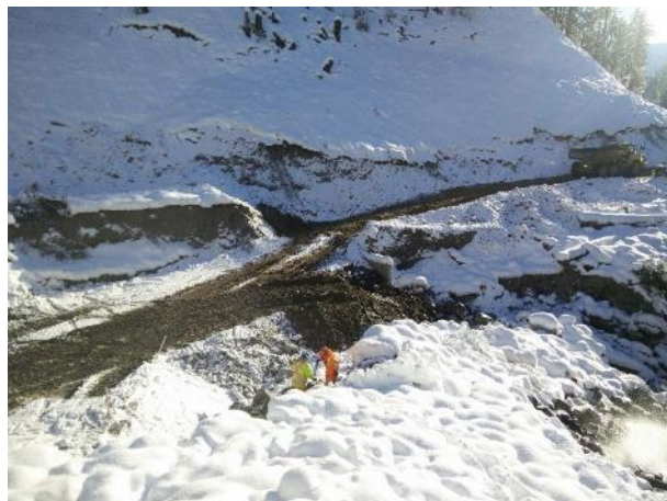
Photo 14 – CE digging small sump at the Truckwash Creek over-drain (December 5, 2016).
