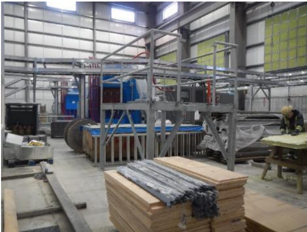
Photo 24 –Electrical works inside the BDRHEF Powerhouse (December 12, 2016).
