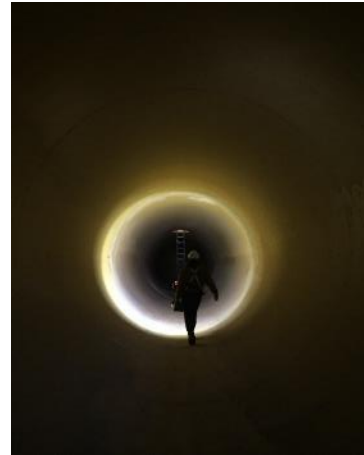
Photo 13 – Final penstock walkthrough with CE (December 15, 2016).
