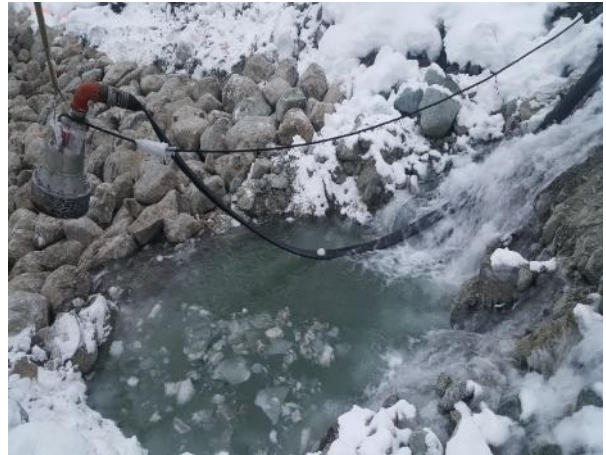
Photo 17 – Removal of pumps and rewatering of Truckwash Creek (December 9, 2016).
