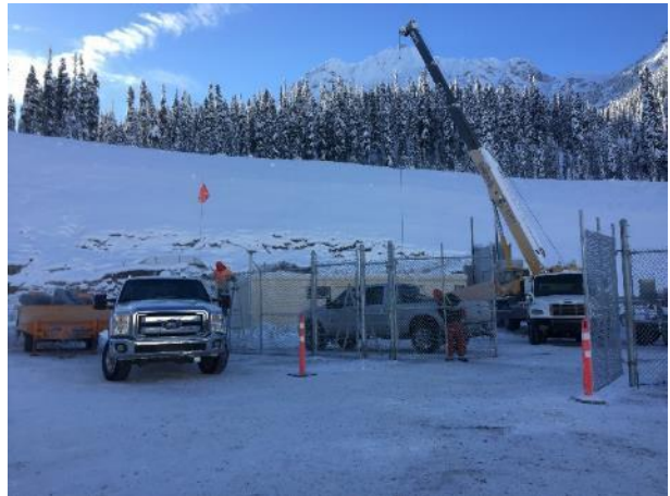
Photo 10 – Installation of gated perimeter fence around ULRHEF Intake (December 15, 2016).
