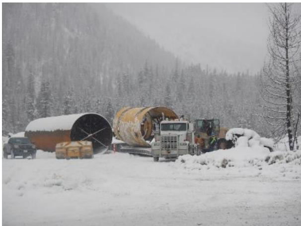
Photo 1 – CE removal of excess penstock pipe from KM41.7 (December 10, 2016).
