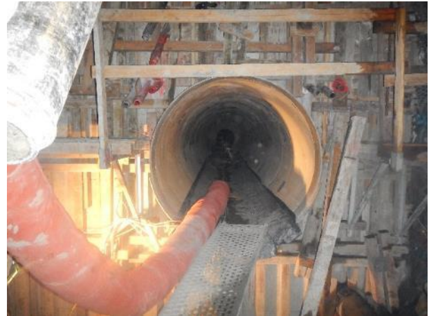
Photo 23 – Steel Liner and Tunnel Plug inside the BDRHEF tunnel portal (December 9, 2016).
