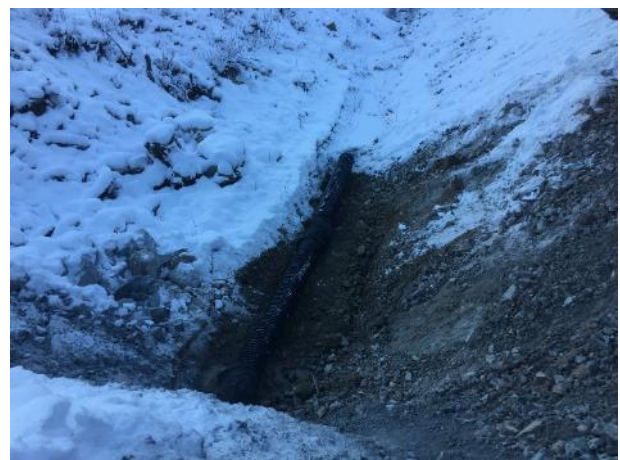
Photo 27 - BDRHEF Spoil Pile culvert installation (December 13, 2016).
