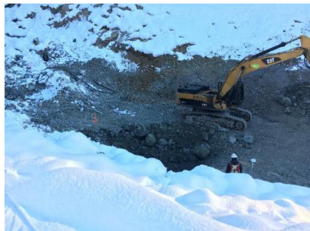
Photo 15 – Excavating of key to install geomembrane at Truckwash Creek over-drain (December 6, 2016).
