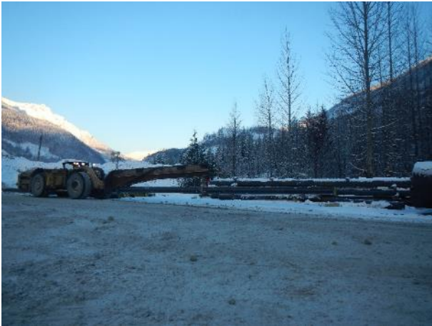
Photo 22 – Installation of the flushing pipe into BDRHEF tunnel (December 12, 2016).
