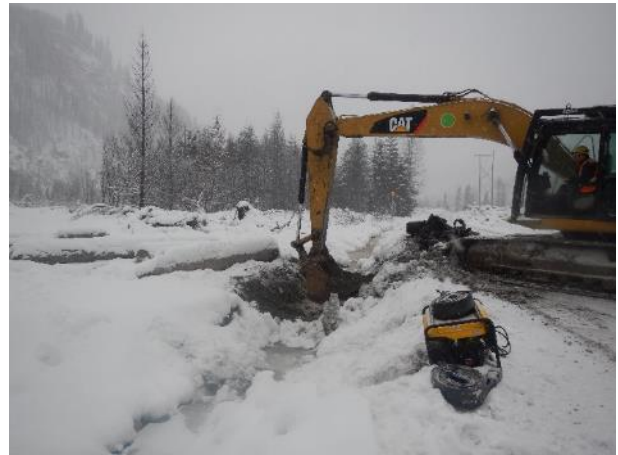
Photo 6 - Removal of PAG spoil pile culvert at KM41.7 (December 10, 2016).
