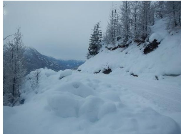
Photo 21 – Current conditions of the BDRHEF intake access road (December 10, 2016).
