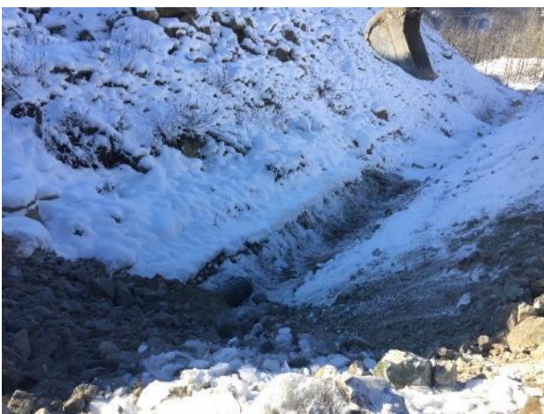
Photo 26 – BDRHEF Spoil Pile culvert installation (December 12, 2016).
