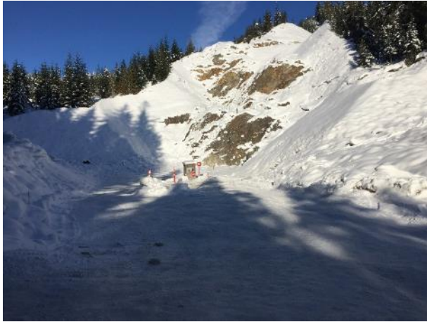
Photo 11 – Winter conditions at the ULRHEF Downstream Tunnel Portal (December 15, 2016).
