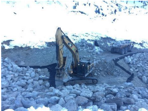
Photo 16 – Geomembrane and riprap placement at Truckwash Creek over-drain (December 7, 2016).
