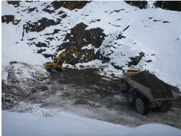
Photo 10 – Backfill of the penstock - lower tunnel portal connection (December 1, 2016)
