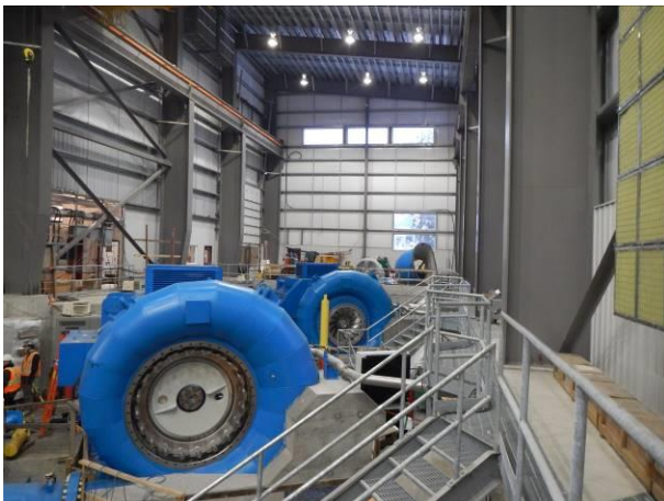
Photo 17 – Mechanical and electrical works in the ULRHEF powerhouse (November 25, 2016)
