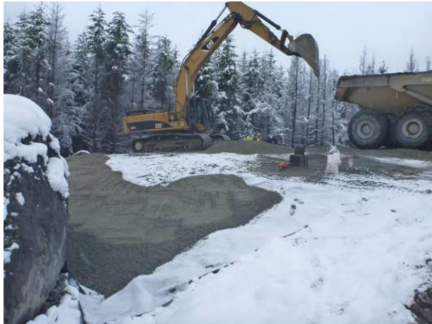
Photo 1 – Capping the PAG storage pile at KM41.7 (November, 27, 2016).
