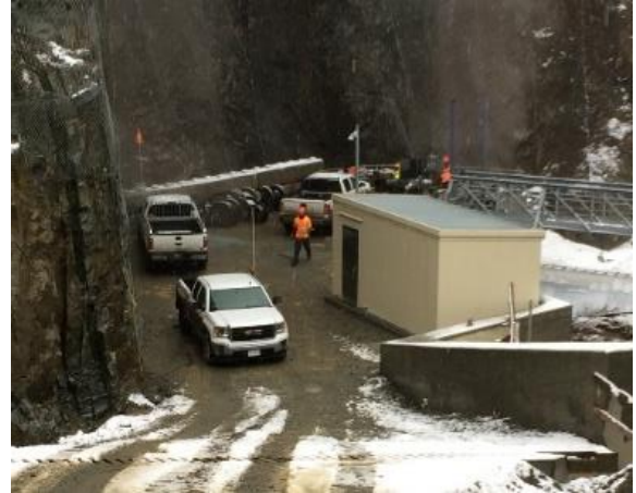
Photo 21 – Crews installing electrical components at BDRHEF intake (November 20, 2016).
