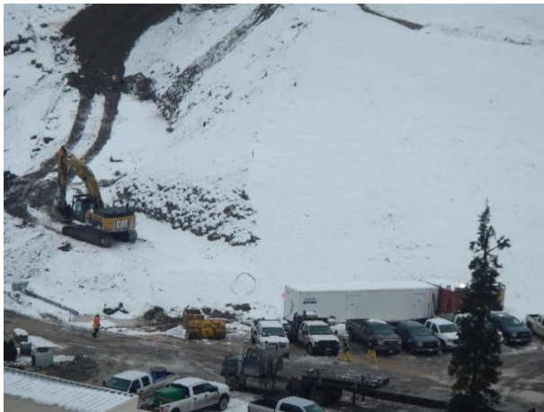
Photo 7 – Deactivation of the temporary access road to the ULRHEF intake (November 21, 2016).
