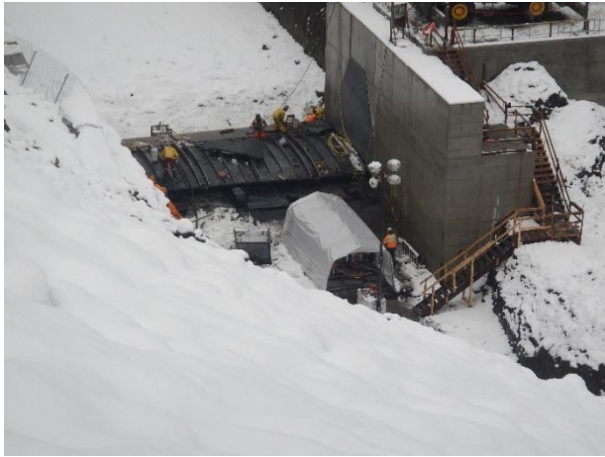
Photo 5 – Repair works on the Obermeyer weir (November 21, 2016).
