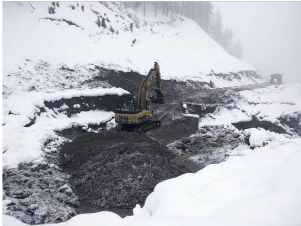
Photo 16 – Rebuilding the penstock over drain to design specifications post-flood event (December 3, 2016).
