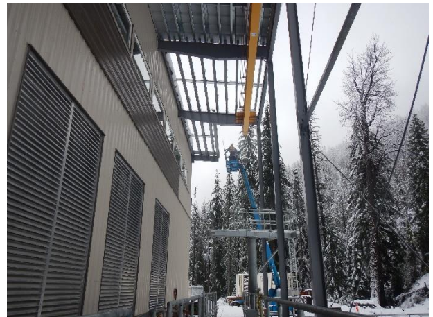
Photo 18 – CE addressing deficiencies on the ULRHEF powerhouse superstructure (November 25, 2016)
