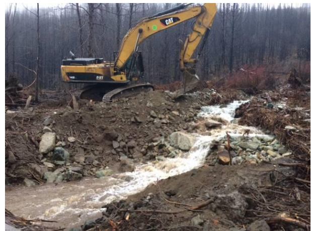
Photo 23 – Diverting stream 9 back into the original channel (November 22, 2016).
