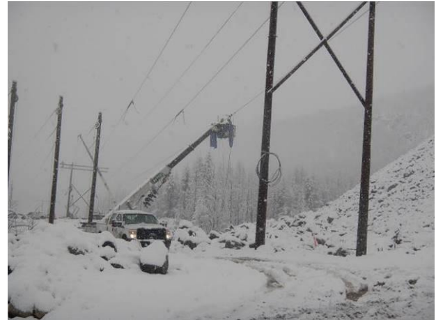
Photo 30 – Crews working on the switch at structure 17 in Segment 2 (November 22, 2016).
