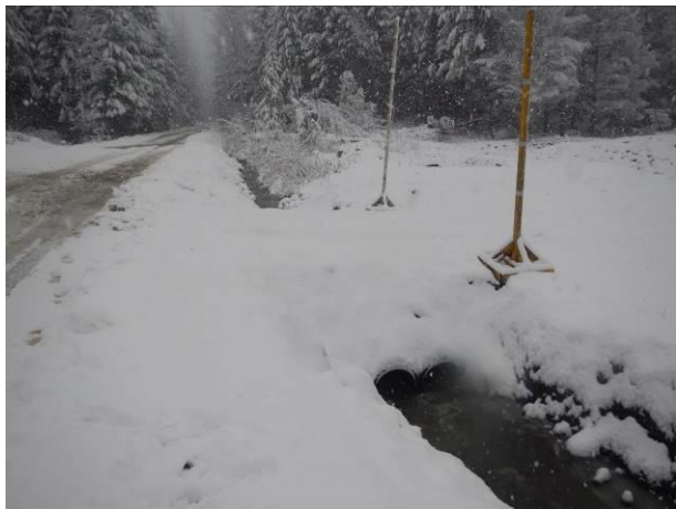
Photo 3 – Newly installed culverts at the PAG storage access road (November 24, 2016).
