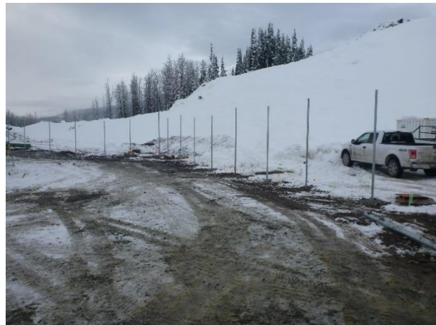
Photo 8 – Installation of chain linked fence around the ULRHEF intake (November 30, 2016).
