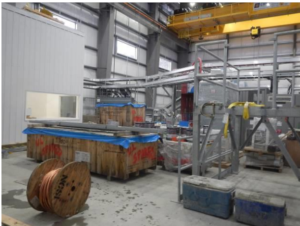
Photo 25 – Electrical works in the BDRHEF powerhouse (November 24, 2016).
