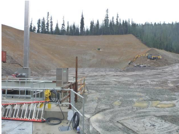
Photo 7 – Completed back fill of the BEBO tunnel wall (November 14, 2016).
