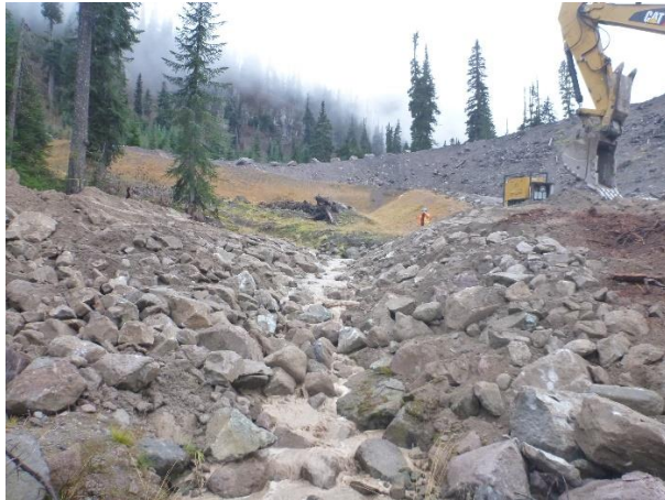
Photo 13 – Commissioning the newly constructed channel following culvert removal (November 15, 2016).
