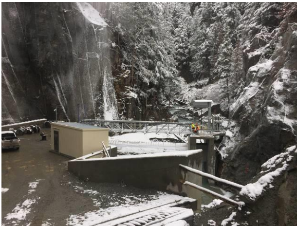
Photo 23 – Electrical works at the BDRHEF intake (November 19, 2016).
