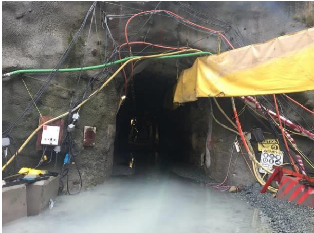
Photo 25 – BDRHEF downstream tunnel portal (November 19, 2016).
