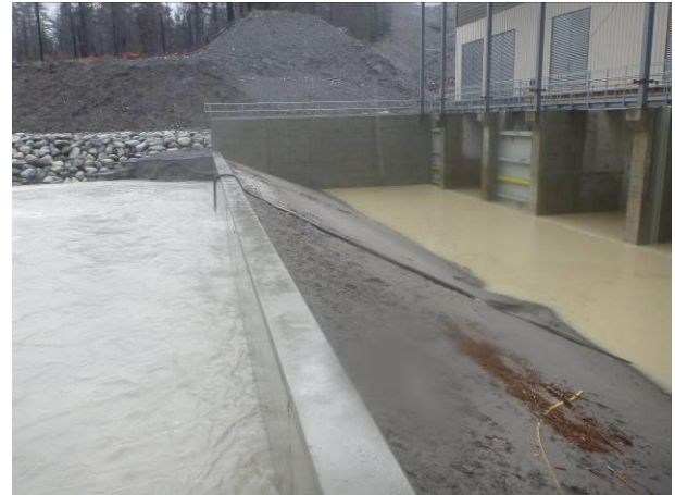
Photo 21 – Dewatering the ULRHEF tailrace (November 12, 2016).
