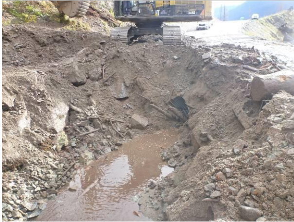
Photo 1 – Removal of debris blocking the invert of the KM44 culvert (November 10, 2016).
