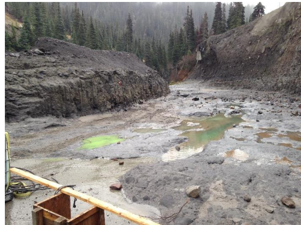
Photo 16 – Spilled sealant in ponds downstream of the Obermeyer structure (November 18, 2016).
