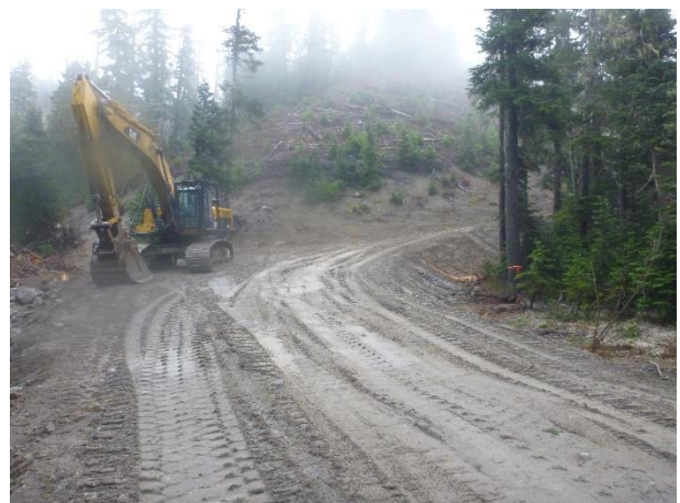
Photo 6 – Newly completed access to the ULRHEF intake (November 11, 2016).
