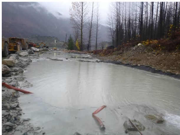
Photo 27 – BDRHEF downstream tunnel settling ponds (November 13, 2016).
