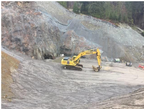
Photo 17 – Crews backfilling the downstream tunnel portal (November 18, 2016).
