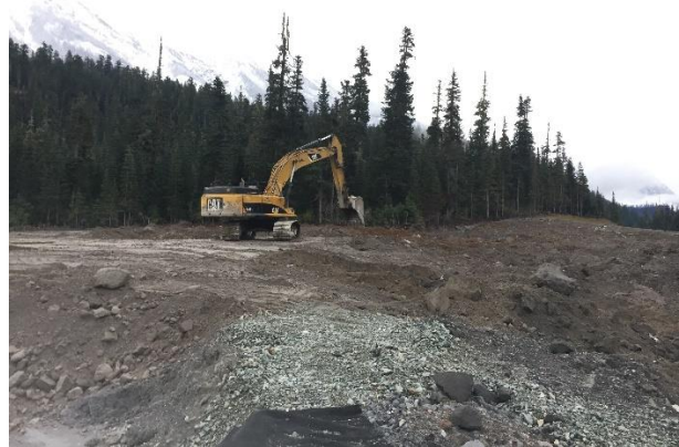
Photo 14 – Reclamation of the upstream tunnel settling ponds (November 18, 2016).
