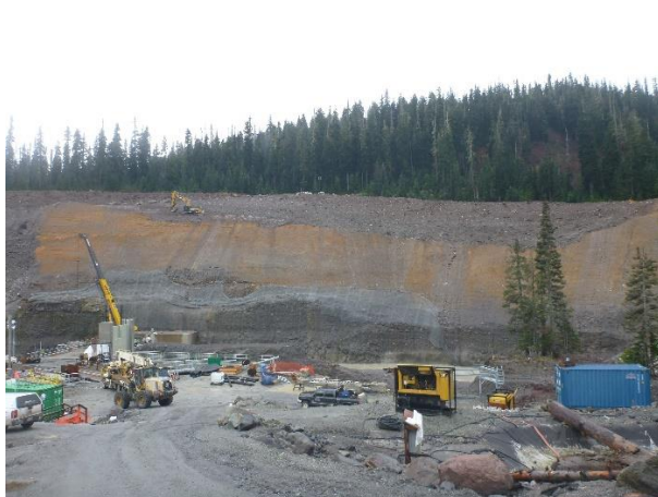
Photo 11 – Re-working the slope on river right of the intake (November 13, 2016).
