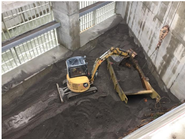
Photo 9 – Crews removing sand deposited behind the coarse trash rack (November 18, 2016).
