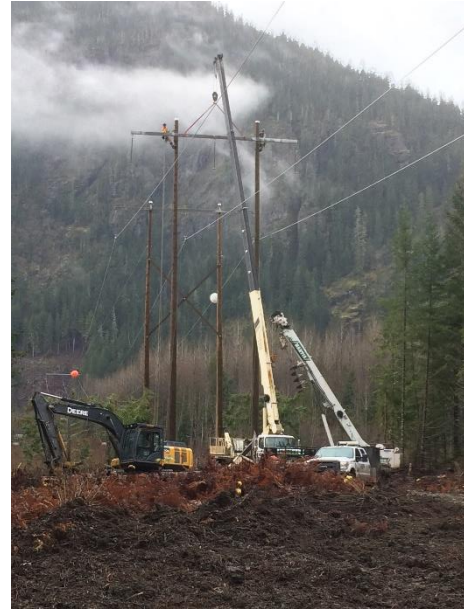
Photo 29 – Repairing structures damaged in the November 8 and 9 heavy rain event (November 13, 2016).
