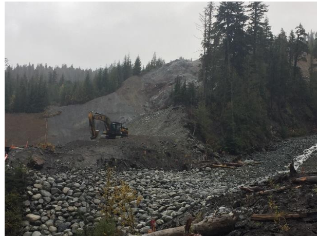
Photo 12 – Backfill of the Mountain Goat corridor on the right bank of Truckwash Creek (October 26, 2016).
