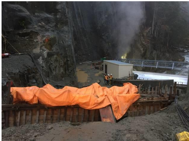
Photo 19 – Formwork and concrete for the BDRHEF intake cross-ditch (November 1, 2016).
