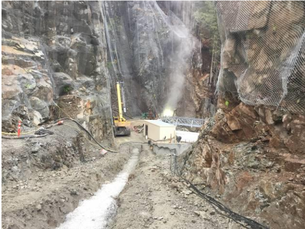
Photo 17 – Buried conduit excavation on the BDRHEF intake access road (October 26, 2016).
