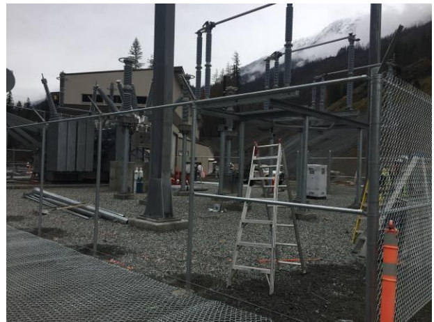
Photo 15 – Installation of the chain link fence surrounding the ULRHEF switchyard (October 26, 2016).
