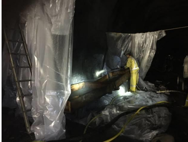
Photo 5 – Final shotcrete application in the ULRHEF tunnel (November 1, 2016).
