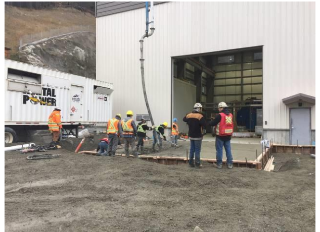
Photo 22 – Concrete pour for the BDRHEF service bay entrance (November 5, 2016).
