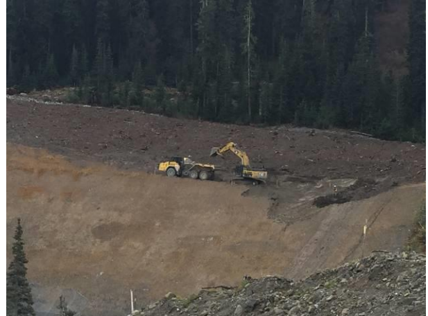
Photo 6 – Excavation above the Obermeyer channel (November 4, 2016).
