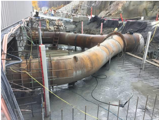
Photo 21 – Manifold installation at the BDRHEF powerhouse (November 5, 2016).
