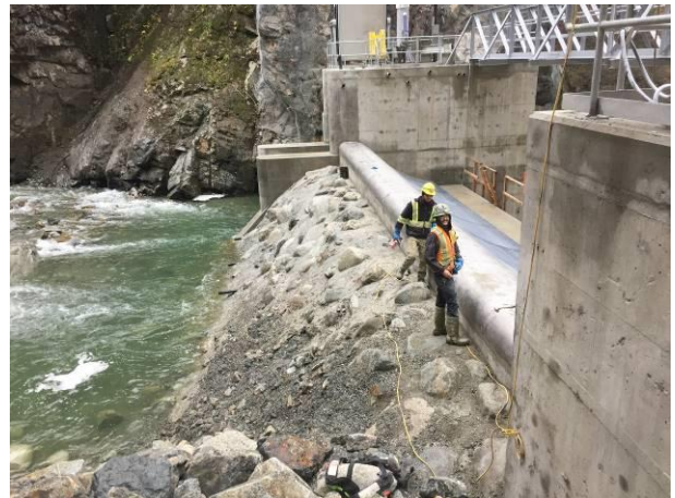
Photo 20 – Hand grouting the BDRHEF Coanda (November 5, 2016).
