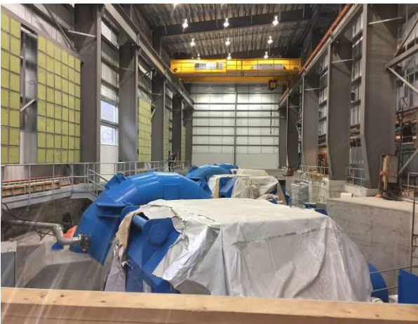
Photo 14 – Andritz mechanical and electrical works in the ULRHEF powerhouse (November 4, 2016).
