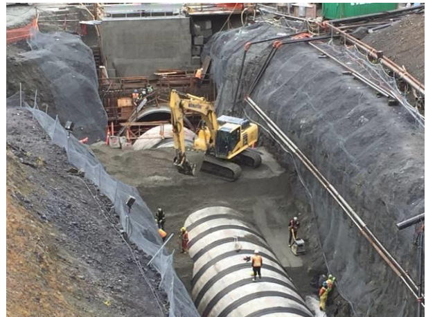
Photo 4 – Back fill of the BEBO tunnel wall (October 28, 2016).
