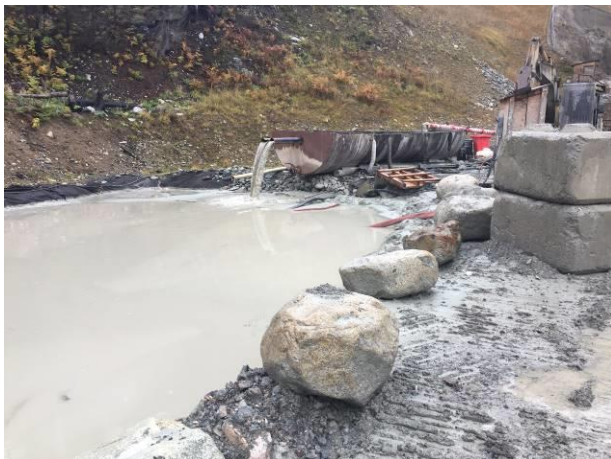
Photo 23 – BDRHEF downstream tunnel settling ponds (October 23, 2016).
