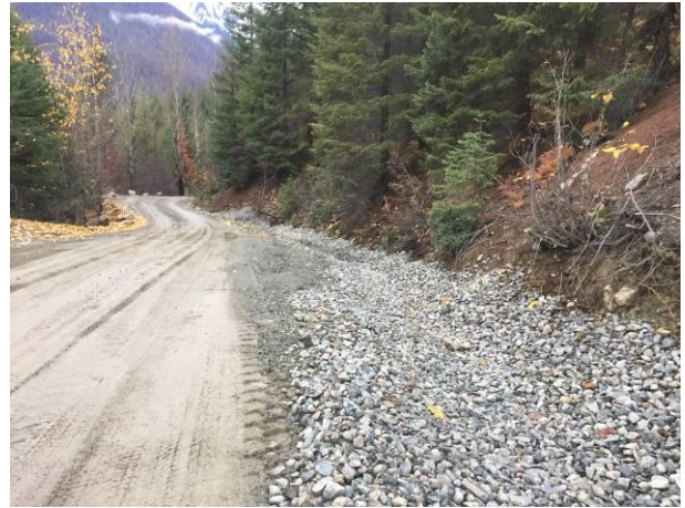
Photo 18 – Rock lined ditching along the BDRHEF intake access road (November 4, 2016).
