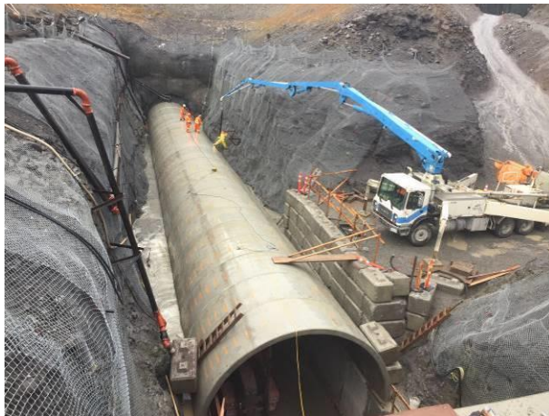
Photo 3 – BEBO tunnel arch installation and grouting (October 25, 2016).
