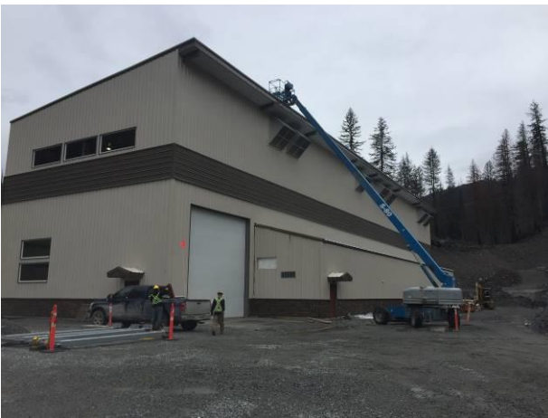
Photo 16 – Crews addressing deficiencies on the superstructure of the ULRHEF powerhouse (November 4, 2016).
