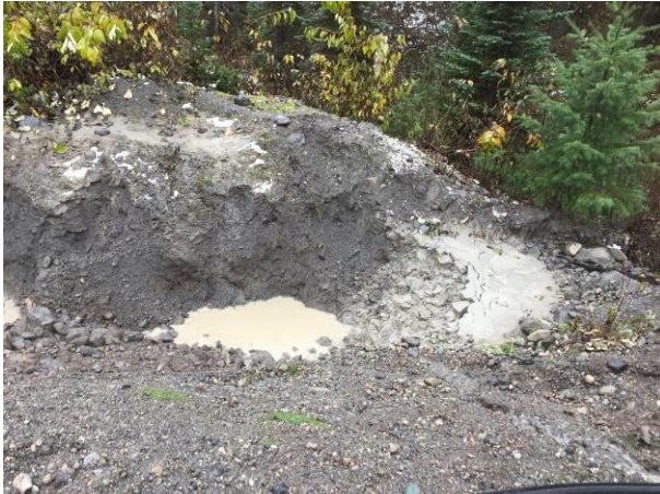
Photo 3 – Infiltration pond re-excavated on river left of KM49 bridge (October 15, 2016).
