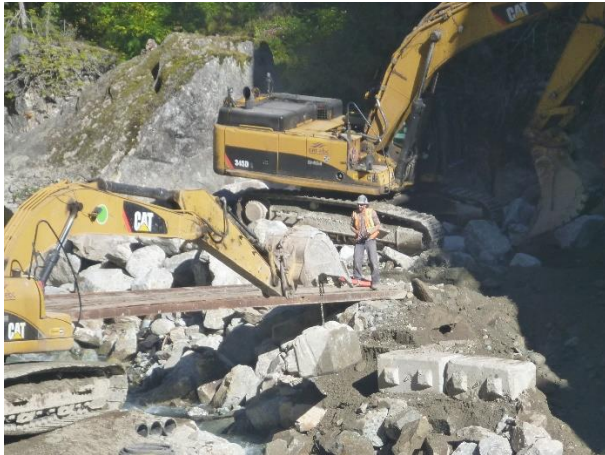
Photo 21 – Removal of the temporary bridges at the BDRHEF upstream cofferdam (October 10, 2016).
