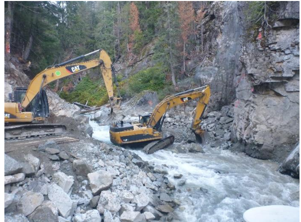
Photo 22 – One time wet crossing at the BDRHEF upstream cofferdam (October 10, 2016).
