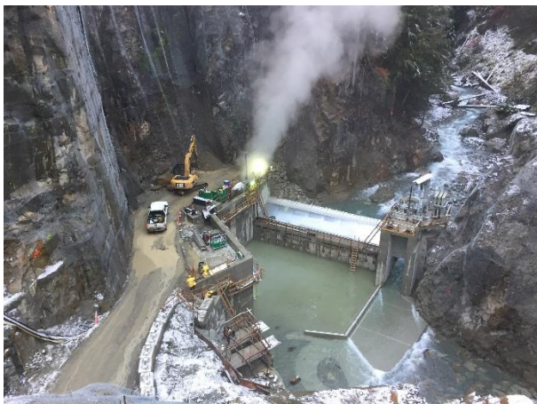
Photo 23 – View of Boulder Creek flowing through the BDRHEF sluice way (October 16, 2016).
