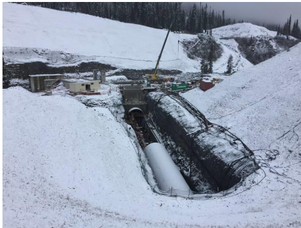
Photo 7 – BEBO tunnel formwork, rebar, concrete works, and arch installation (October 18, 2016).
