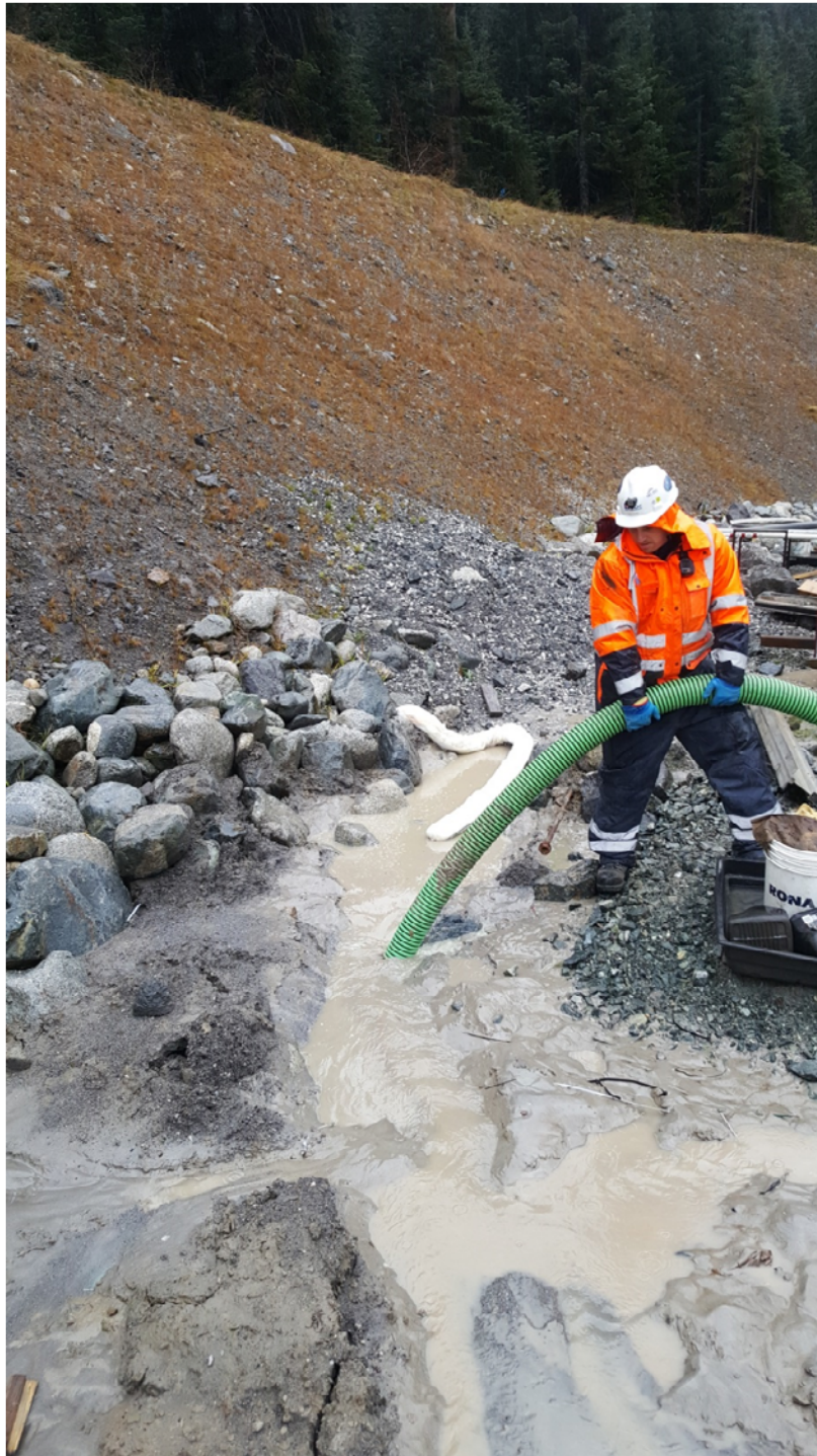
Figure 5: Vacuum truck removing contaminated water and sediment from ditch-line
