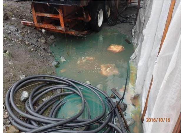
Photo 4 – Diesel spill from overflowing the generator at KM48.5 (October 16, 2016).
