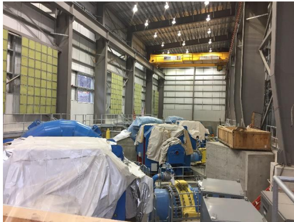
Photo 17 – Andritz mechanical and electrical works in the ULRHEF powerhouse (October 21, 2016).
