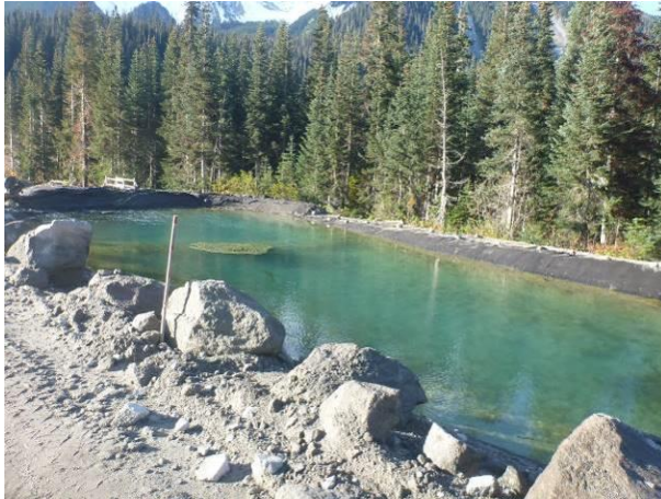
Photo 9 – ULRHEF upper tunnel water treatment system, pond No. 7 (October 10, 2016).
