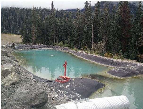
Photo 7 - ULRHEF water treatment system, pond No. 7 (September 25, 2016).
