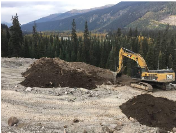
Photo 1 – Reclamation of the KM49.5 spoil pile (October 1, 2016)
