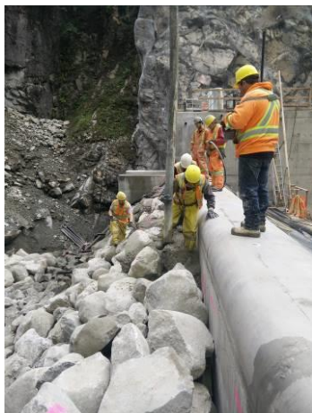
Photo 15 – Grouting rip rap upstream of the BDRHEF intake structure (September 26, 2016).
