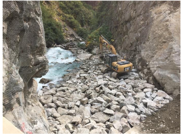
Photo 18 – Rip rap placement downstream of the BERHEF intake structure (September 29, 2016).
