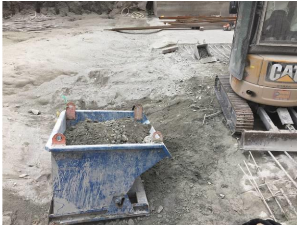
Photo 5 – Cleanup of demolished concrete at the ULRHEF Obermeyer structure (October 1, 2016).
