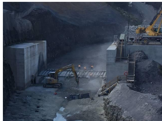
Photo 4 – Concrete demolition for the Obermeyer repair works (September 30, 2016).
