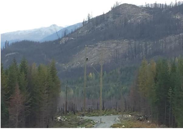
Photo 29 – Fiber optic cable installation in Segment 1 (October 1, 2016).
