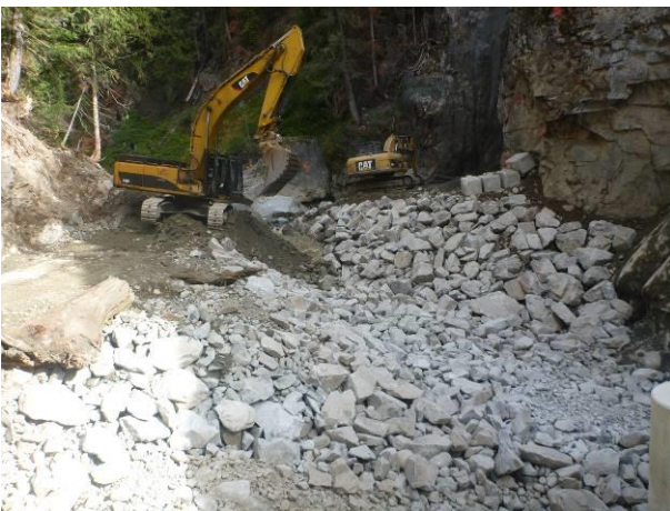
Photo 19 – Excavation and rip rap placement of the upstream coffer dam (October 3, 2016).
