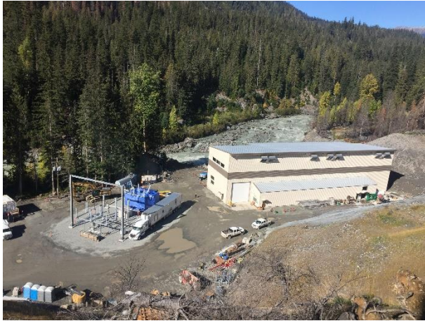
Photo 12 – ULRHEF powerhouse and switch yard (September 28, 2016).
