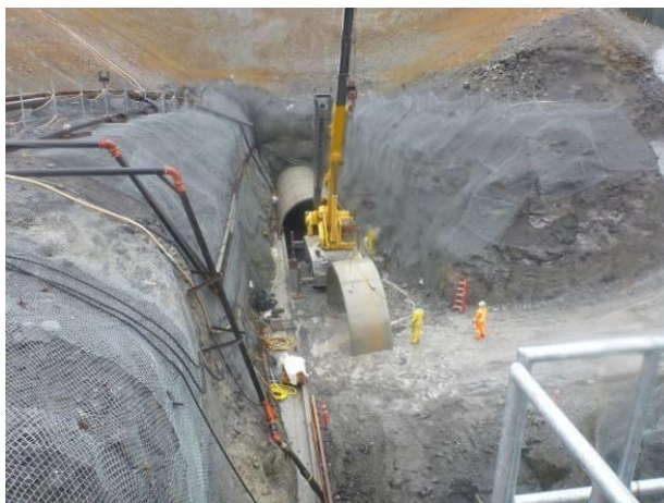
Photo 3 – BEBO tunnel arch installation (October 8, 2016).
