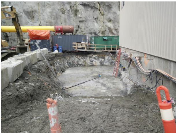
Photo 27 – Excavation and mudslab pour for the BDRHEF bifurcation (September 25, 2016).
