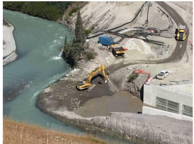
Photo 8 – Crews deploying and cleaning up the hydraulic spill (September 12, 2016).
