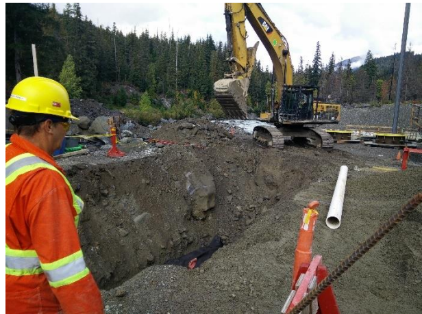
Photo 18 – Backfill of the ULRHEF powerhouse septic field (September 22, 2016).
