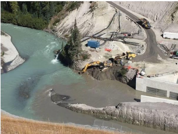
Photo 9 – Crews finishing the ULRHEF upstream cofferdam removal (September 13, 2016).
