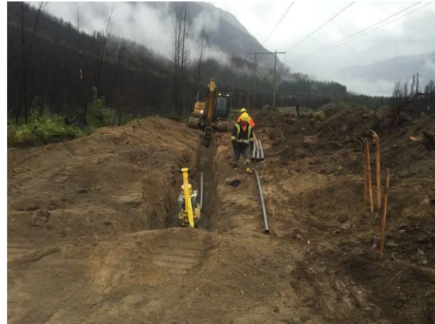
Photo 24 – Conduit installation between BDRHEF powerhouse and intake access road (September 17, 2016).
