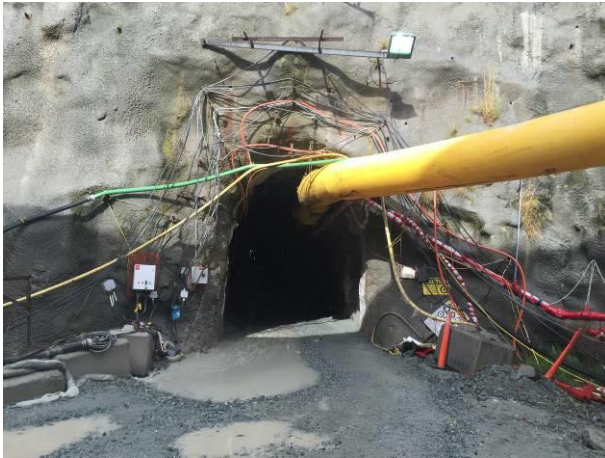
Photo 23 – BDRHEF lower-tunnel portal (September 17, 2016).
