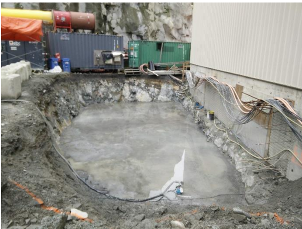
Photo 25 – BDRHEF bifurcation excavation and mud slab cure (September 24, 2016).
