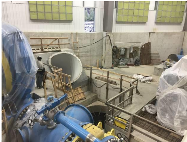
Photo 17 – Andritz electrical works in the ULRHEF powerhouse (September 17, 2016).
