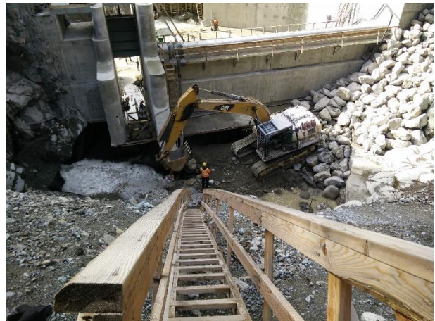
Photo 22 – Installation of scour protection upstream of the BDRHEF intake (September 24, 2016).
