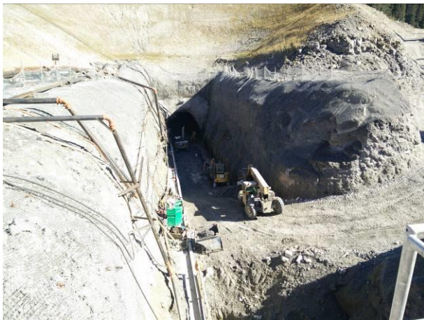
Photo 3 – ULRHEF upper tunnel portal and BEBO tunnel wall (September 14, 2016).
