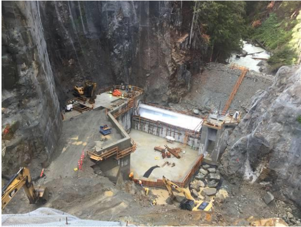
Photo 19 – Excavation of the BDRHEF intake crane pad (September 17, 2016).
