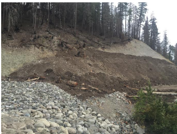
Photo 16 – Reconstructed left bank of Truckwash Creek (September 16, 2016).
