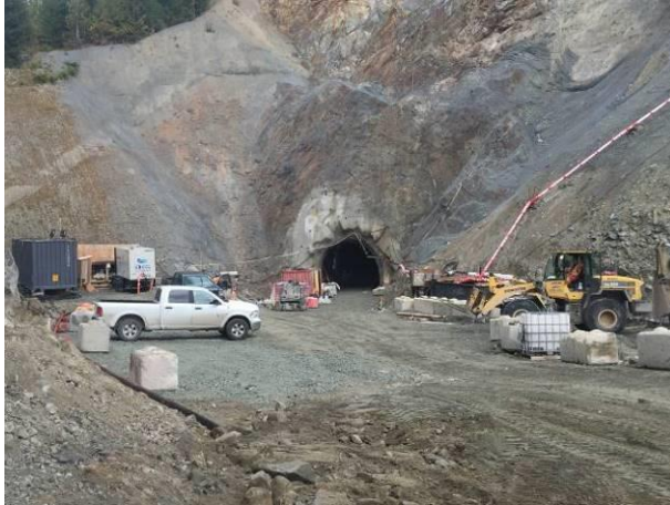
Photo 15 – ULRHEF lower tunnel portal (September 16, 2016).
