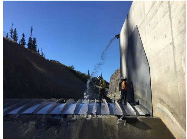
Photo 12 – Discharge of 3-inch pump directed to the Obermeyer diversion channel (September 15, 2016).
