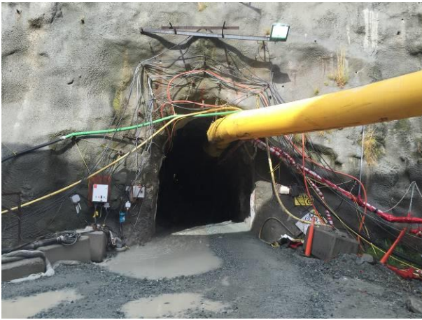
Photo 21 – BDRHEF lower-tunnel portal (August 29, 2016).
