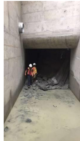
Photo 22 – BDRHEF tunnel breakthrough at the intake structure (August 29, 2016).
