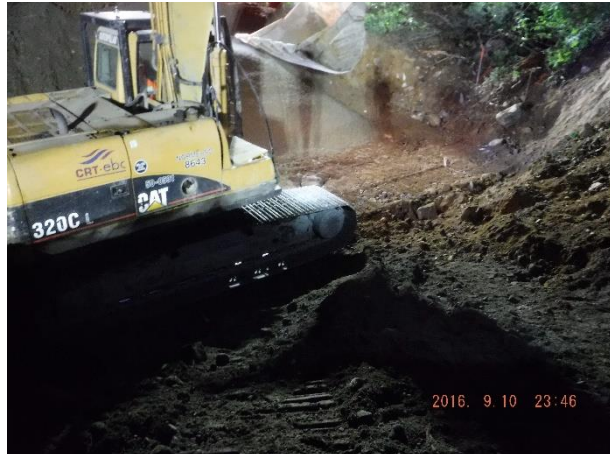
Photo 3 – Excavation for the replacement of the KM41.2 stream crossing (September 10, 2016).
