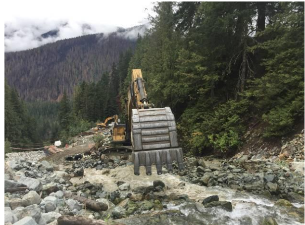
Photo 12 - Diverting Truckwash Creek into the newly constructed penstock over drain (September 2, 2016).
