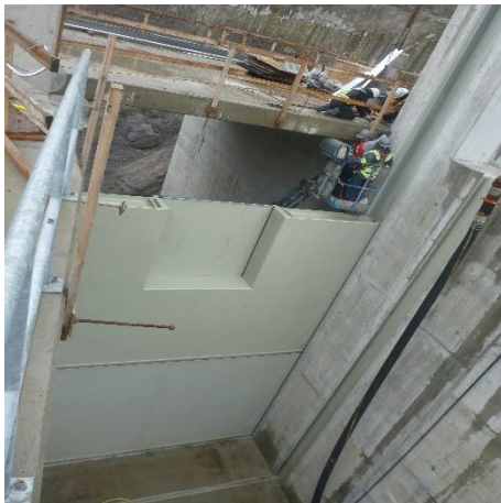
Photo 7 – Installation of the ULRHEF sluice gate (September 7, 2016).
