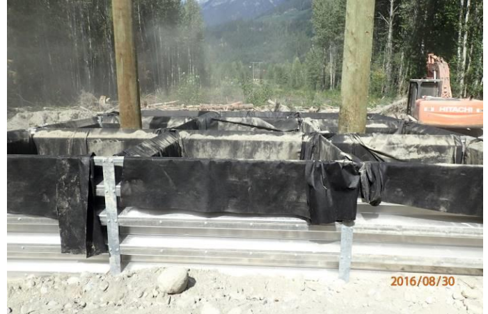
Photo 25 – Nearing completion of the armouring for pole structure 140 (August 30, 2016).
