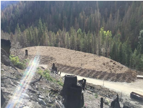
Photo 17 – Reclamation of ULRHEF powerhouse spoil (September 8, 2016).
