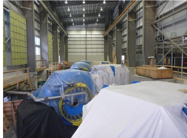
Photo 16 – Andritz mechanical works in the ULRHEF powerhouse (August 30, 2016).
