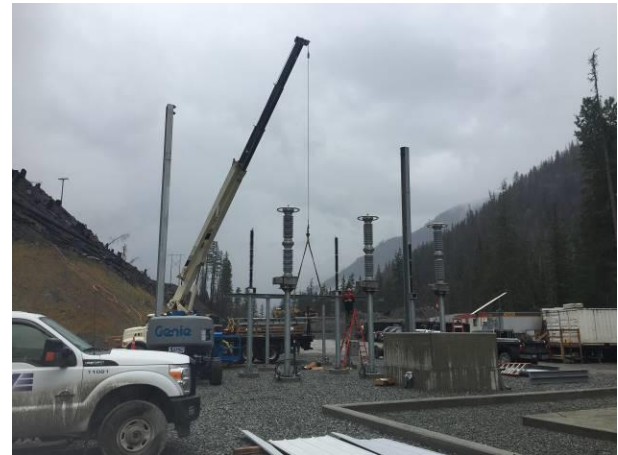
Photo 18 – Westpark construction of the switchyard at the ULRHEF powerhouse (August 31, 2016).
