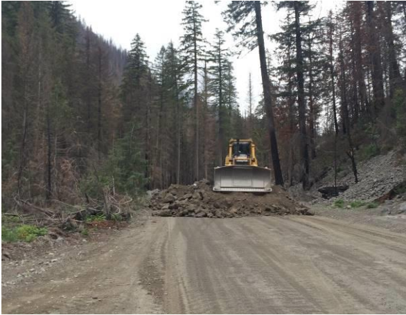
Photo 15 – Maintenance on the ULRHEF powerhouse access road (August 28, 2016).
