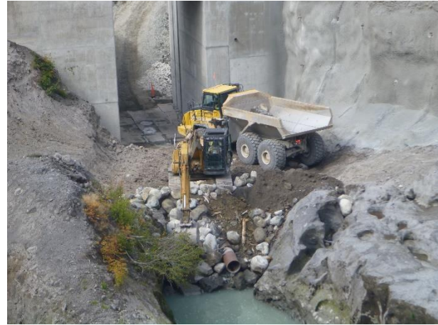
Photo 6 – Removal of the ULRHEF downstream cofferdam (September 6, 2016).
