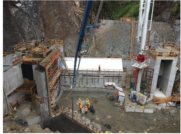
Photo 20 – Installation of BDRHEF Coanda screen (August 28, 2016).
