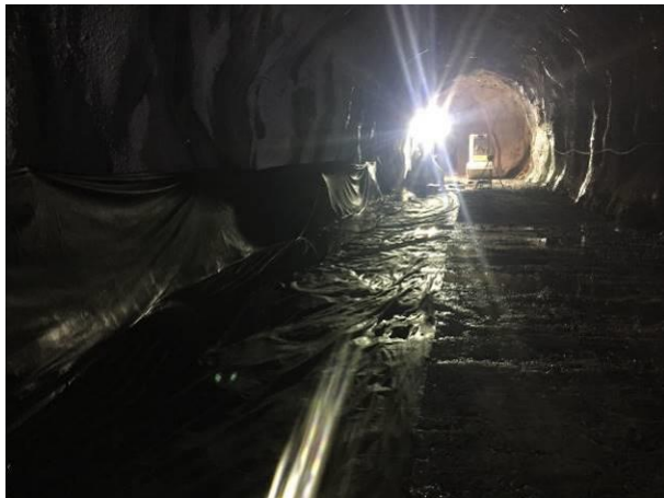
Photo 9 – Lower-tunnel portal (September 06, 2016).
