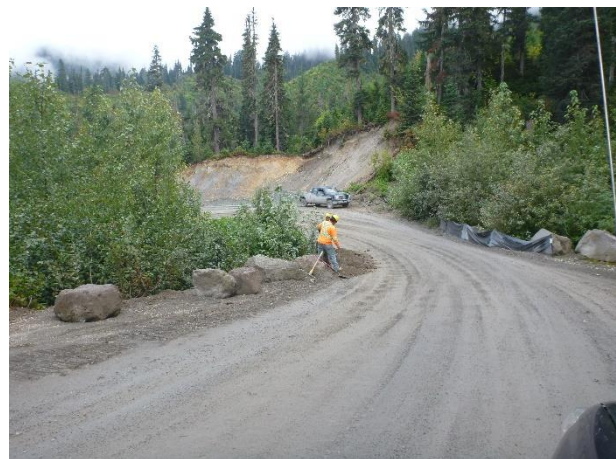
Photo 2 – Silt fence replacement at KM48 of the Lillooet River FSR (September 6, 2016).
