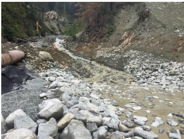
Photo 13 - Truckwash Creek fully diverted into the newly constructed channel (September 2, 2016).
