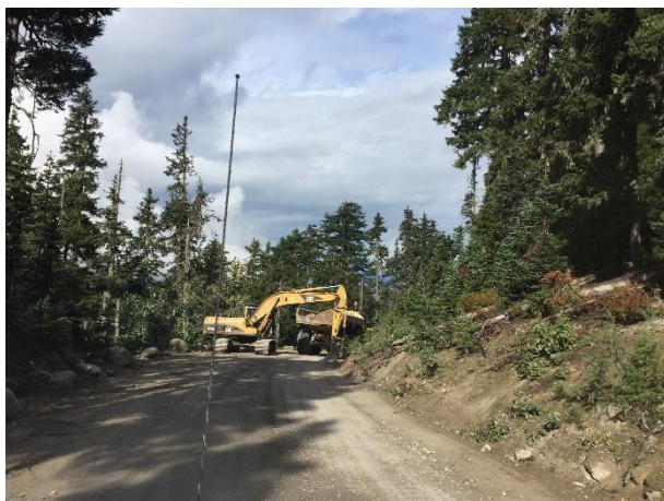
Photo 1 – Ditch maintenance at KM46 of the Lillooet River FSR (August 29, 2016).
