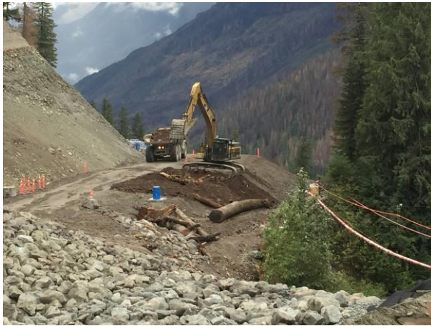
Photo 11 - Reclamation of the penstock right-of-way east of Truckwash Creek (September 1, 2016).
