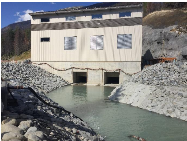
Photo 23 – BDRHEF powerhouse and tailrace (September 2, 2016).
