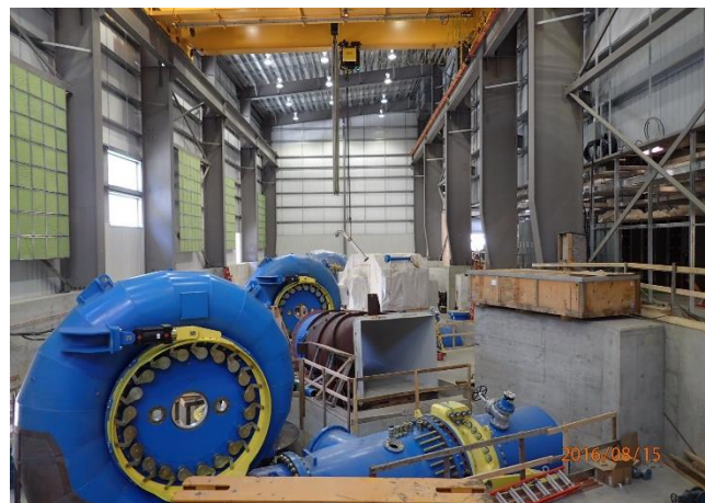
Photo 14 – Andritz mechanical works in the ULRHEF powerhouse (August 15, 2016).
