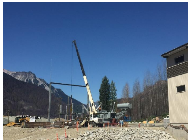
Photo 22 – Construction of switch yard adjacent to the BDRHEF powerhouse (August 17, 2016).
