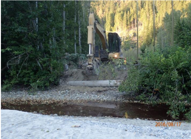
Photo 23 – Preparing sill logs for temporary bridge crossing (August 17, 2016).
