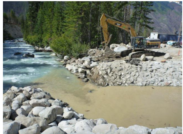
Photo 20 – BDRHEF tailrace excavation and armouring (August 23, 2016).
