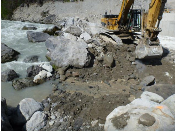
Photo 9 – Start of instream works at ULRHEF tailrace (August 24, 2016).
