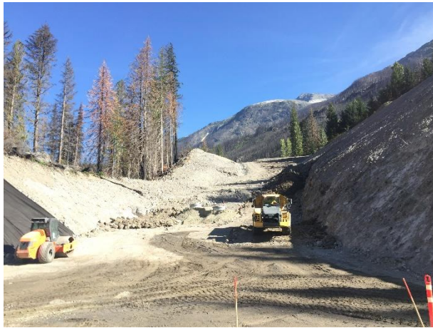
Photo 7 – Backfill and compaction near the powerhouse (August 19, 2016).
