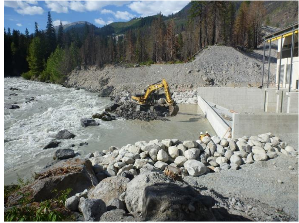
Photo 10 – Instream excavation of the tailrace tie-in. (August 24, 2016).
