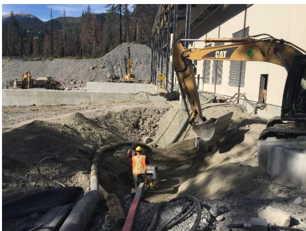
Photo 13 – Backfill and compaction around the powerhouse dewatering sump. (August 26, 2016).
