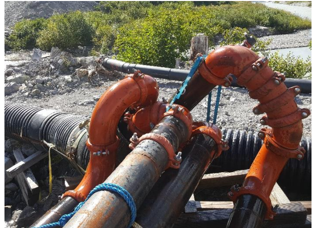
Photo 5 – Repairs to the leaking dewatering pipes (August 23, 2016).
