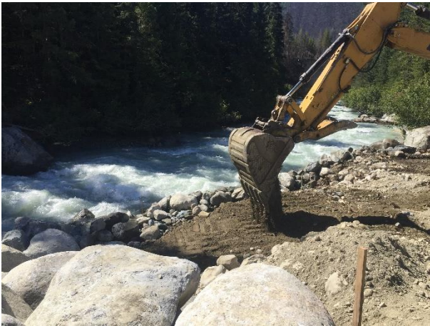
Photo 17 – Extension of a working pad to facilitate BDRHEF tailrace works (August 17, 2016).
