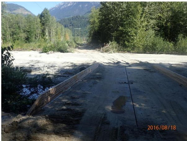
Photo 25 – Temporary access path used to access structure 140 (August 18, 2016).
