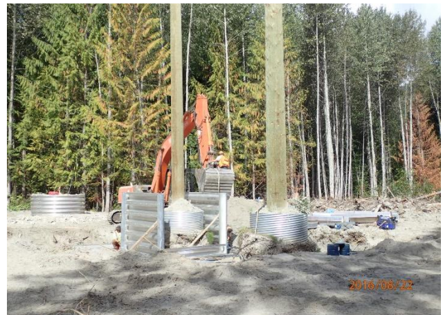
Photo 26 – Bin wall construction at structure 140 (August 22, 2016).
