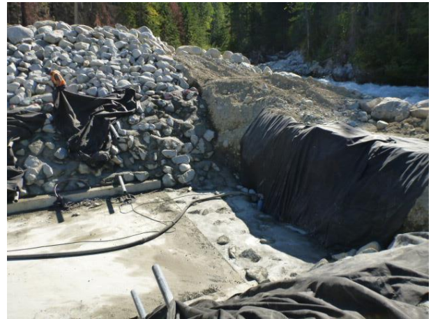
Photo 18 – Grouted riprap apron at BDRHEF tailrace completed in the dry (August 20, 2016).
