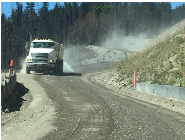
Photo 1 – Dust suppression at KM43.5 of the Lillooet River FSR (August 15, 2016).
