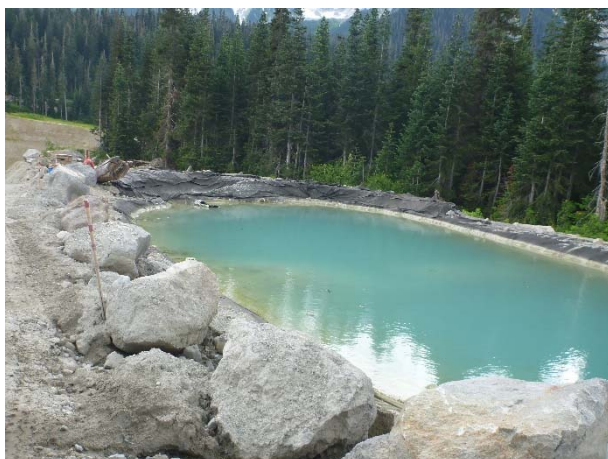
Photo 5 – ULRHEF upper tunnel water treatment system, pond No. 7 (July 17, 2016).
