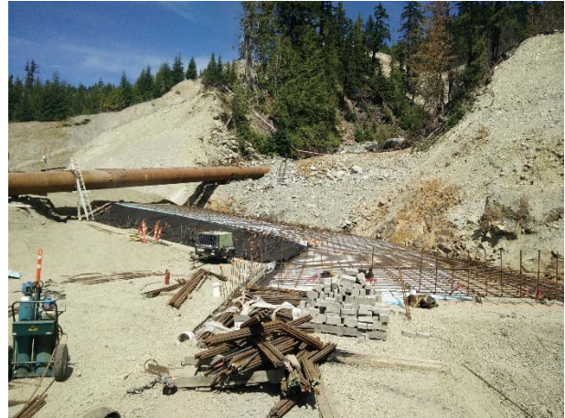
Photo 9 – Formwork and rebar for the Truckwash Creek crossing protection slab (July 28, 2016).
