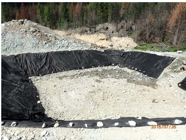
Photo 17 – Excavation of new BDRHEF lower tunnel portal pond (July 26, 2016).
