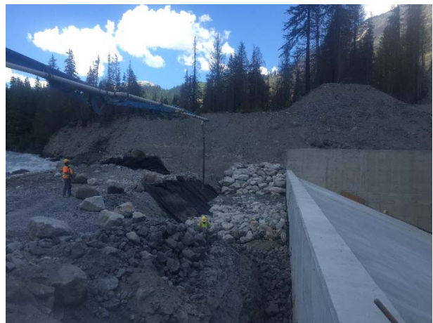
Photo 13 – Grouting riprap at the ULRHEF tailrace (July 26, 2016).
