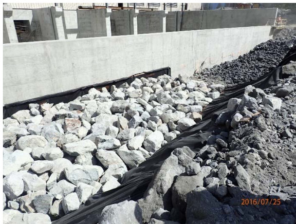
Photo 12 – Placement of riprap at the ULRHEF tailrace (July 25, 2016).
