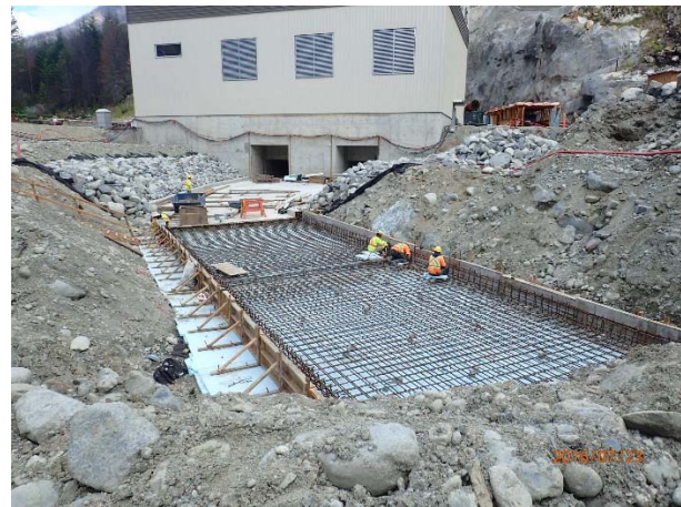
Photo 16 – Formwork and rebar BDRHEF tailrace (July 23, 2016).
