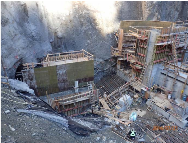
Photo 14 – Formwork and rebar for the tunnel-intake transition (July 21, 2016).
