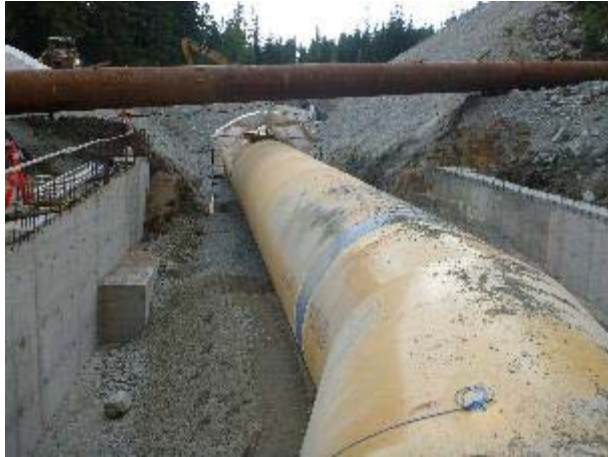
Photo 8 – Penstock welding and coating works through the Truckwash Creek crossing (July 17, 2016).
