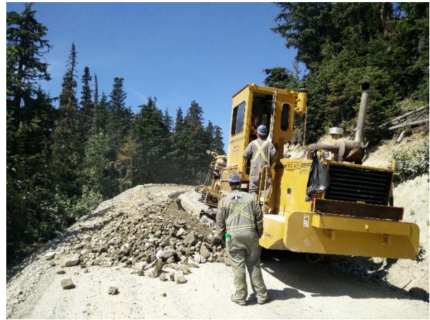
Photo 2 – Conduit trenching and installation on the Lillooet River FSR (July 28, 2016).
