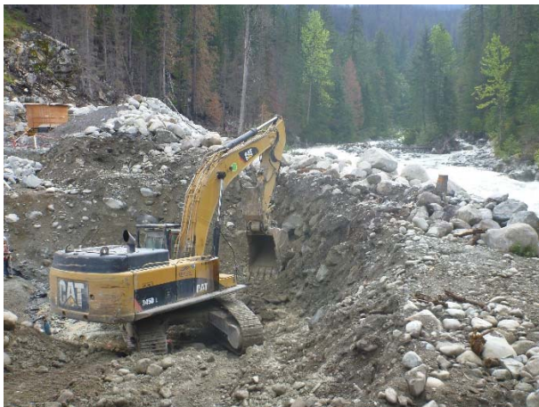
Photo 15 – Excavation of BDRHEF tailrace (July 17, 2016).
