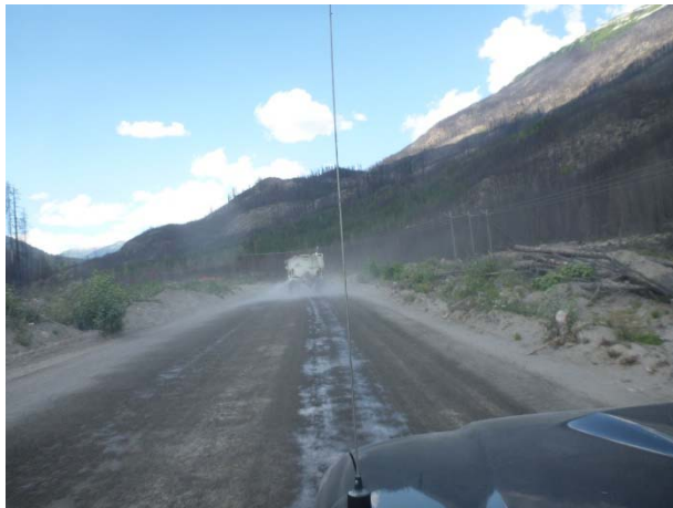
Photo 1 – Dust suppression application on the Lillooet River FSR (July 30, 2016).
