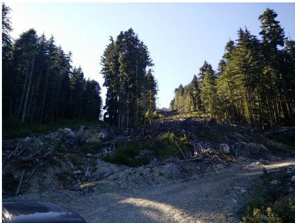
Photo 21 – Ground preparation and anchor installation for structure 316 (July 29, 2016).
