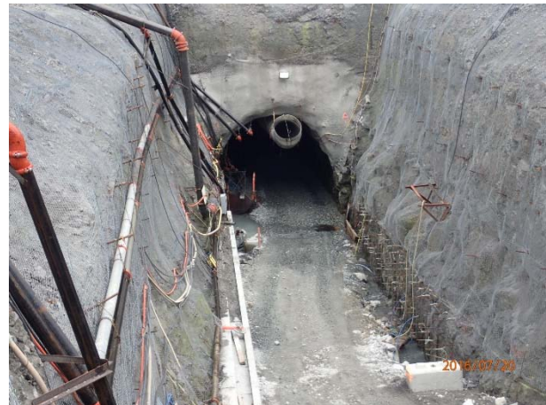
Photo 4 – ULRHEF upper tunnel portal and BEBO wall (July 20, 2016).
