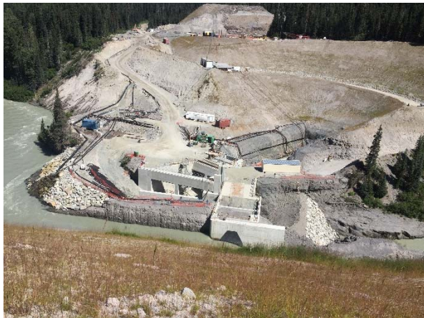
Photo 3 – ULRHEF intake structure (July 27, 2016).
