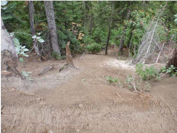
Photo 3 – Trenching material pushed to the downslope of the Lillooet River FSR between KM46.5 – 48 (August 8, 2016).
