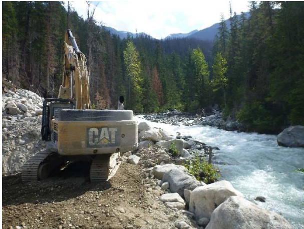
Photo 22 – Construction of access ramp at BDRHEF tailrace (August 7, 2016).
