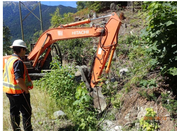
Photo 24 – Ditch cleaning near structure 230 (August 12, 2016).
