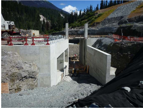
Photo 4 – Preparation for sluice gate installation (August 8, 2016).
