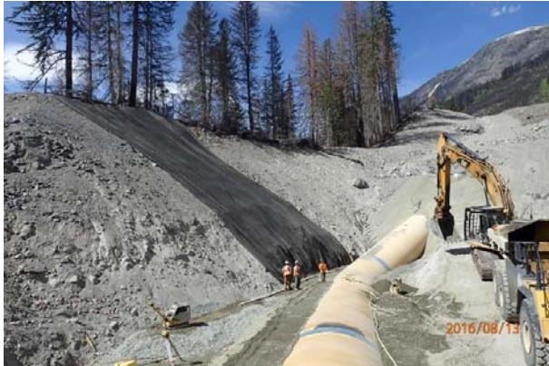
Photo 9 – Backfill and compaction of the penstock east of Truckwash Creek (August 13, 2016).
