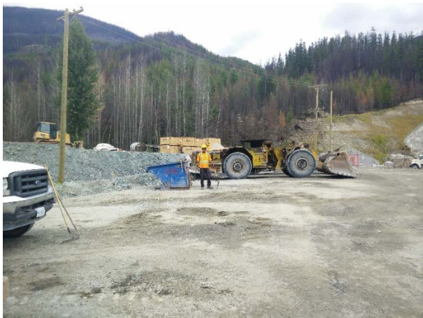
Photo 20 – Worker cleaning up oil spills at BDRHEF powerhouse designated parking area (August 9, 2016).
