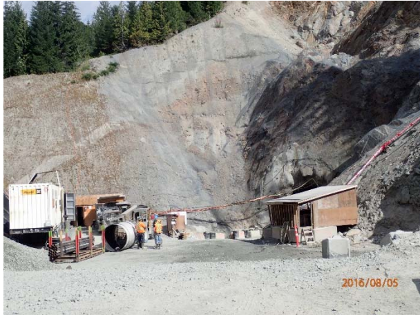
Photo 8 – Lower tunnel portal (August 5, 2016).
