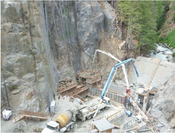
Photo 15 – Formwork, rebar, and concrete works at BDRHEF intake (August 1, 2016).
