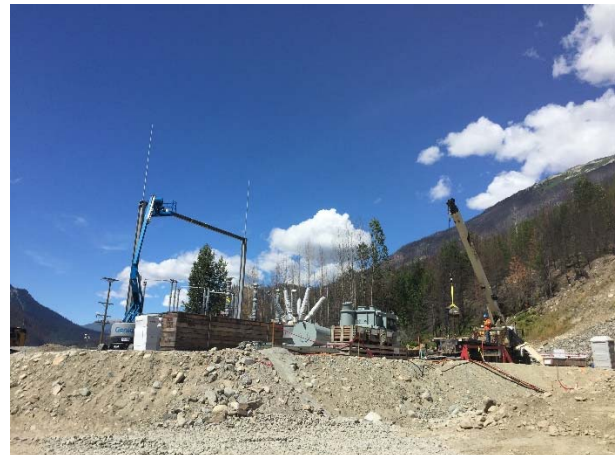
Photo 21 – Construction of the BDRHEF switch yard (August 11, 2016).
