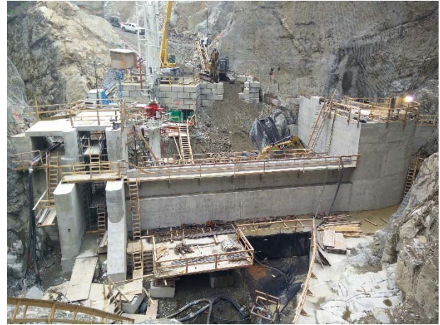
Photo 16 – Formwork and rebar at BDRHEF intake (August 9, 2016).
