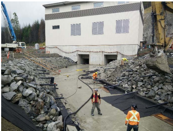
Photo 18 – Placement of rip rap at BDRHEF tailrace (August 8, 2016).
