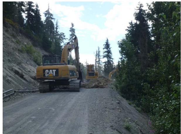
Photo 2 – Conduit trenching and installation on Lillooet River FSR (July 31, 2016).
