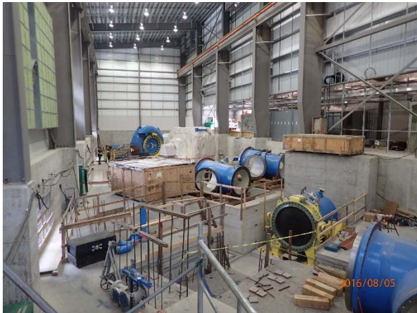
Photo 13 – Andritz mechanical works in the ULRHEF powerhouse (August 5, 2016).
