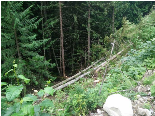
Photo 23 – Felled hazard trees and vegetation management in Segment 11 (August 10, 2016).
