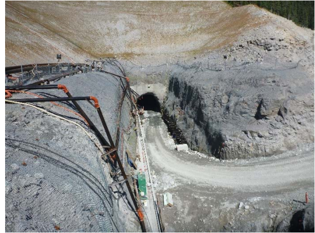
Photo 5 - ULRHEF upper tunnel portal and BEBO wall (August 2, 2016).
