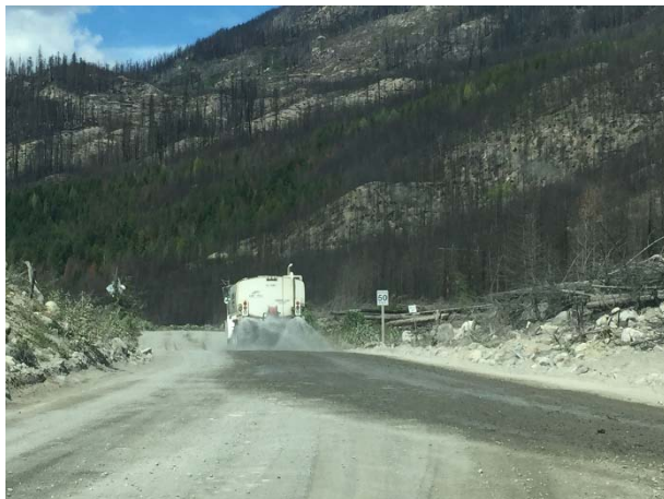
Photo 1 – Dust suppression application on the Lillooet River FSR (August 11, 2016).
