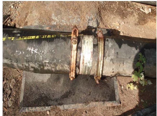
Photo 14 – Leaking hose repaired by CE to address ITM ULR#59 (August 10, 2016).
