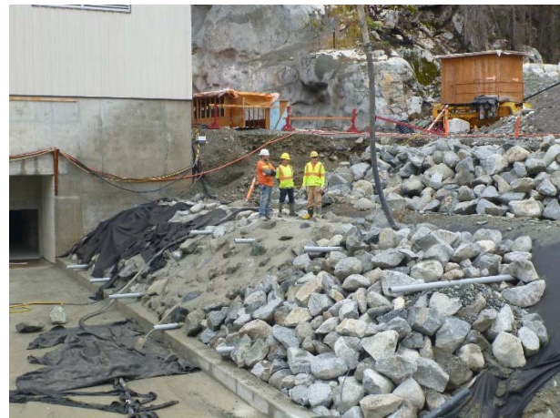
Photo 19 – Grouting riprap at BDRHEF tailrace (August 8, 2016).
