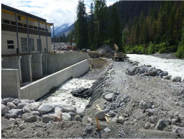
Photo 11 – Excavation and grouted rip rap at ULRHEF tailrace (July 31, 2016).
