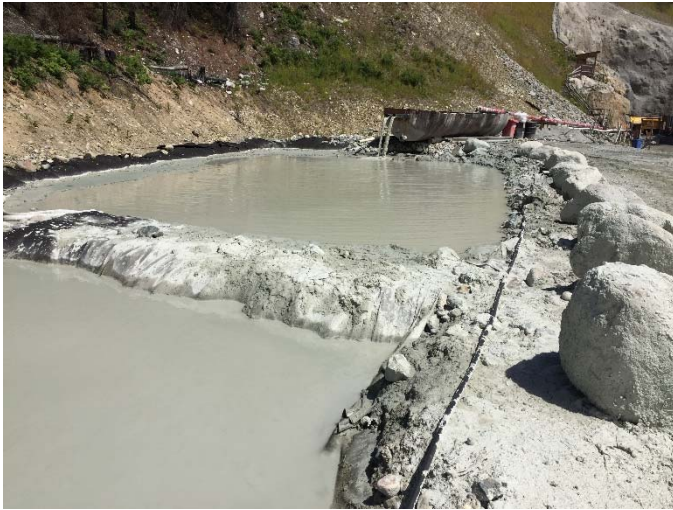
Photo 21 – BDRHEF downstream portal settling ponds (July 6, 2016).
