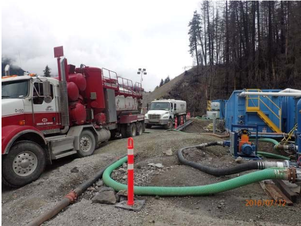
Photo 10 – Sediment removal from the active water treatment system at ASTR-03 (July 13, 2016).
