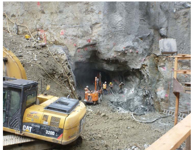
Photo 15 – Stabilization and Shotcrete activities on BDRHEF upper tunnel portal (July 3, 2016).
