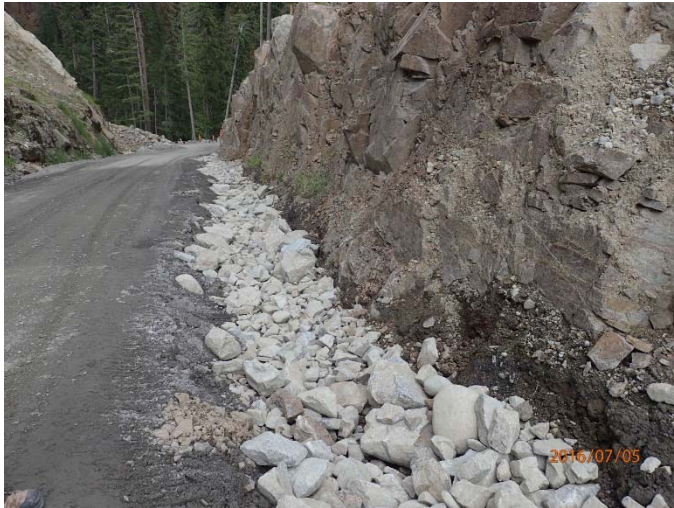
Photo 16 – Rock lined ditch at KM4.5 of BDRHEF intake access road (July 5, 2016).
