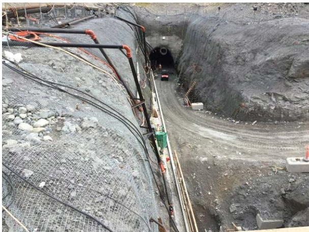
Photo 5 – ULRHEF u/s tunnel portal and BEBO wall (July 6, 2016).
