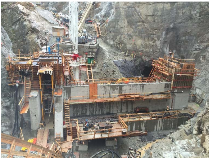
Photo 14 – Concrete works on BDRHEF intake structure (July 7, 2016).
