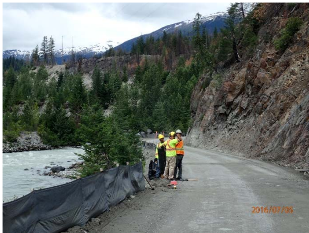
Photo 1 – Silt fence repairs at KM41.2 Lillooet River FSR (July 5, 2016).
