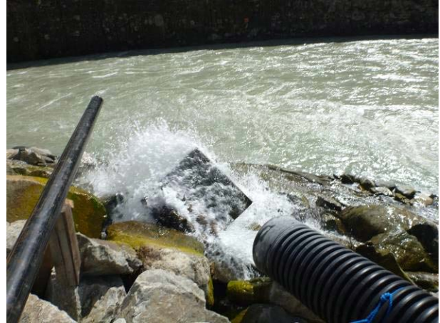
Photo 8 – Discharge of ULRHEF intake water treatment system back to Lillooet River meeting BCWQG (July 3, 2016).
