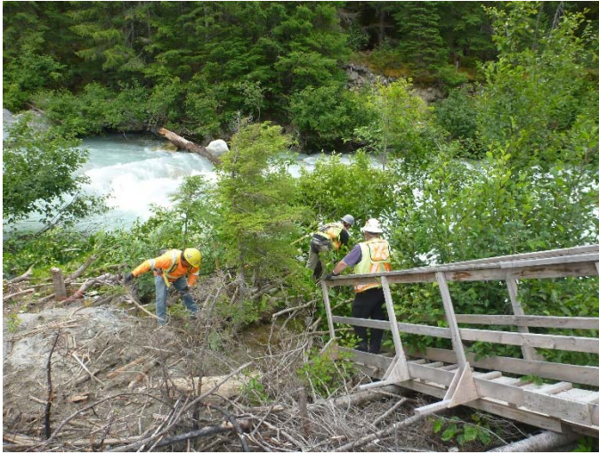
Photo 17 – Hand clearing of Vegetation at the tie-in location of BDRHEF tailrace (July 15, 2016).
