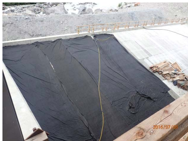
Photo 12 – Concrete curing at ULRHEF tailrace (July 5, 2016).
