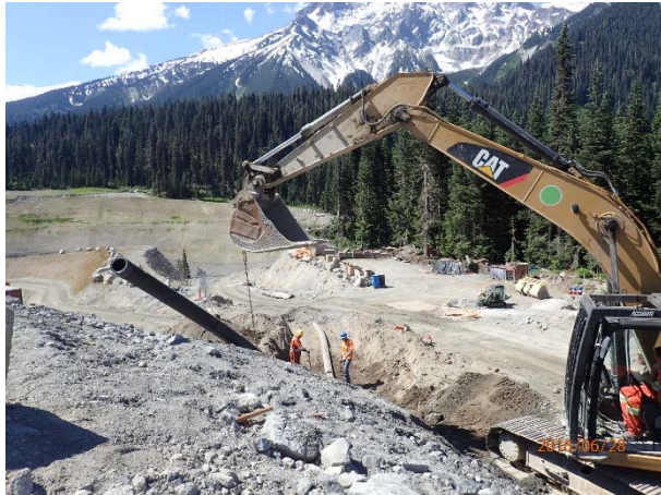
Photo 5 – Installing new pipes to increase dewatering capacity to the ULRHEF water treatment ponds (June 28, 2016).
