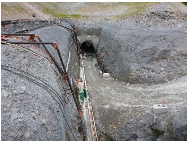
Photo 3 – Crew working on the dewatering pipes at the ULRHEF upper tunnel portal and BEBO wall work areas (June 24, 2016).
