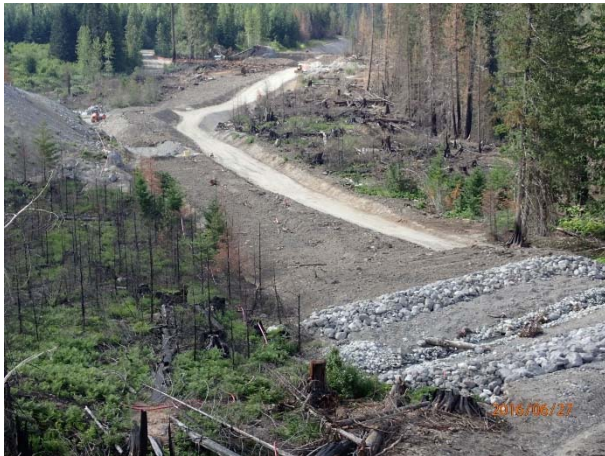
Photo 11 – Overview of penstock alignment at ASTR-04 crossing with organic material and woody debris placement (June 27, 2016).
