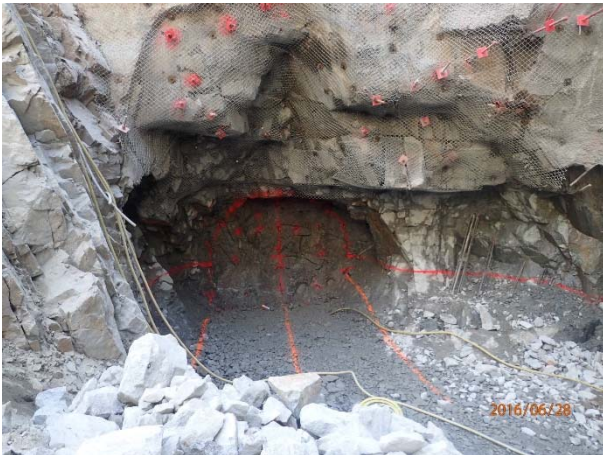
Photo 16 – Drilling pattern for BDRHEF upstream tunnel portal excavation (June 28, 2016).
