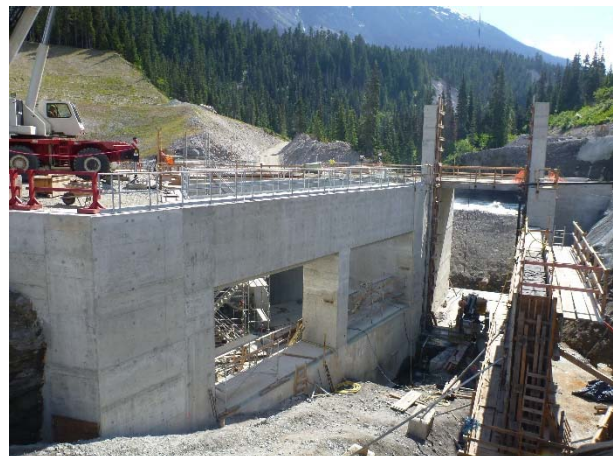
Photo 4 – Rebar and formwork for the ULRHEF sluiceway training wall (June 21, 2016).
