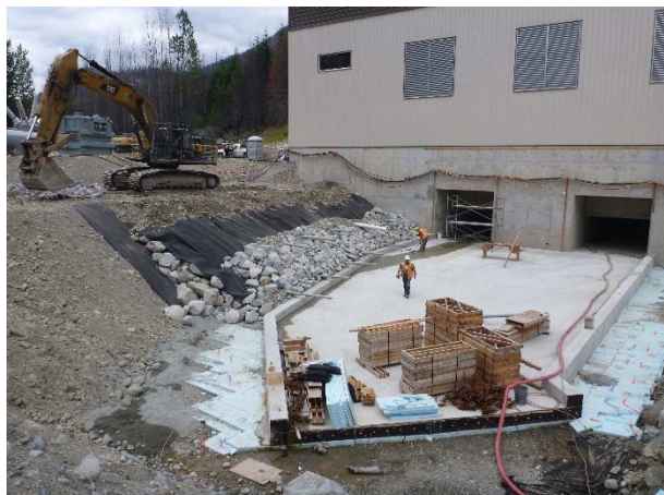
Photo 19– Placing riprap protection along the edges of the tailrace (July 2, 2016).
