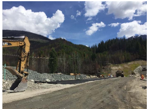
Photo 18 – CE removed hydrocarbon-contaminated soil and lined the parking area near the mechanic laydown along the BDRHEF powerhouse access road (June 29, 2016).
