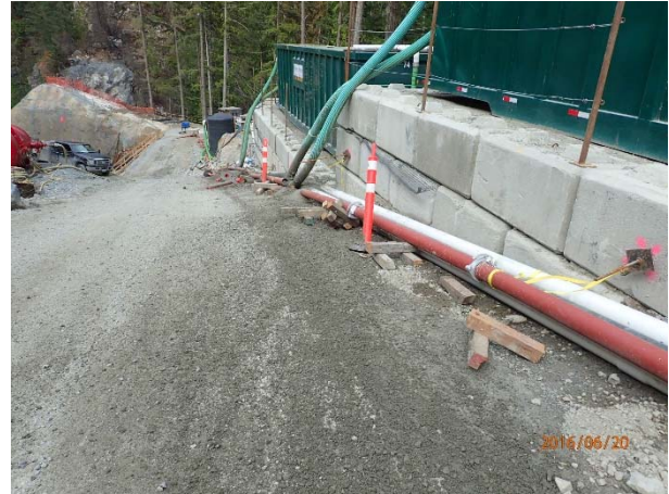
Photo 15 – Concrete delivery pipe supplying the stationary concrete boom arm failed along BDRHEF intake access road (June 20, 2016).
