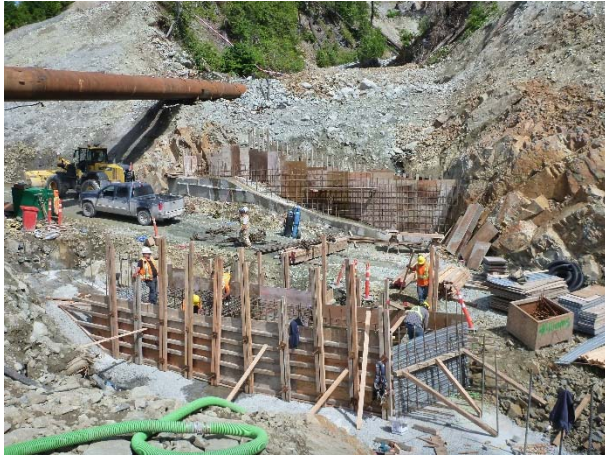
Photo 9 – Rebar and formwork installation for protection of the penstock at the Truckwash Creek crossing (June 25, 2016).
