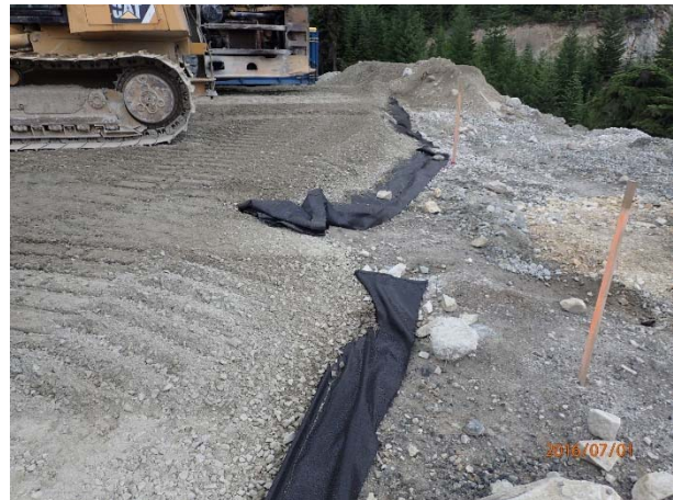
Photo 8 – CE removed small hydrocarbon spots within the parking area for the mechanics laydown and lined the area with impermeable geo-fabric topped with road base material (July 1, 2016).
