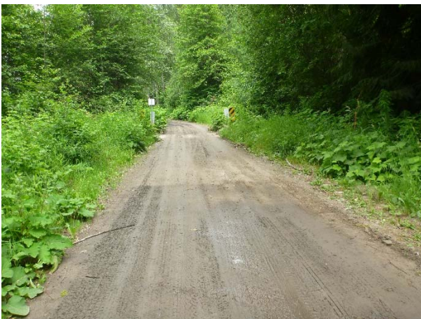
Photo 21 – Dust suppression product application along the Miller Bench FSR. Notice the gap left at the watercourse crossing (June 24, 2016).
