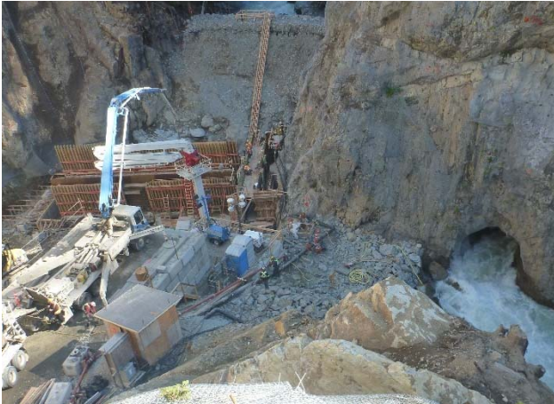
Photo 14 – Formwork, rebar, and concrete works at BDRHEF Intake structure (June 21, 2016).
