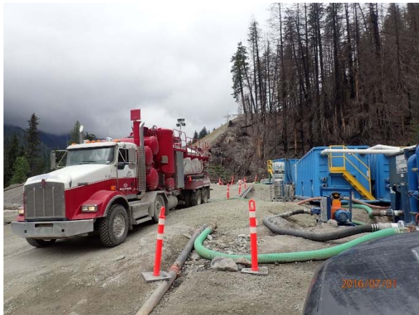
Photo 7 – Sediment removal from the lower tunnel water treatment system (July 1, 2016).
