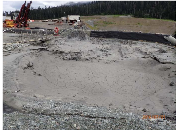
Photo 6 – Cell #1 of the ULRHEF intake water treatment system following 5 days of inactivity in the tunnel and at the intake due to elevated landslide risk (July 1, 2016).
