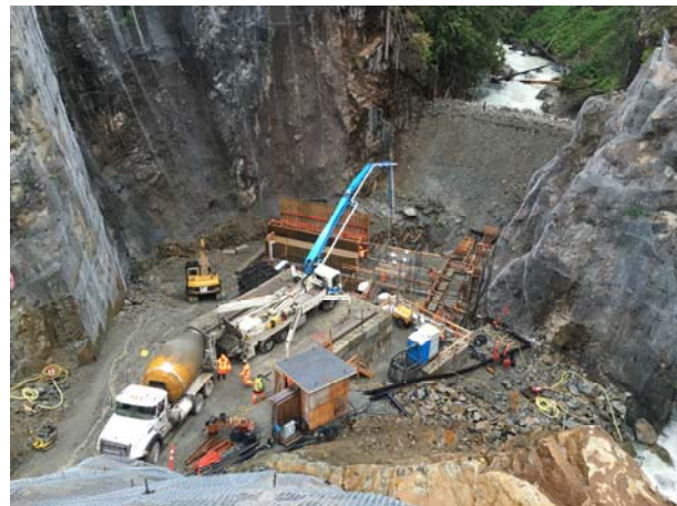
Photo 14 – Formwork, rebar, and concrete works at Boulder Creek Intake Structure (June 13, 2016).
