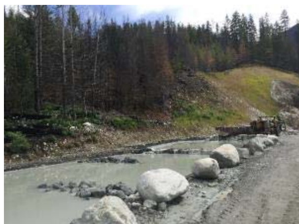
Photo 19 – BDRHEF downstream portal settling ponds (June 14, 2016).
