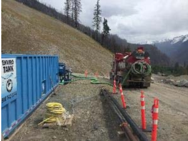
Photo 7 – Sediment removal from the lower tunnel water treatment system (June 17, 2016).
