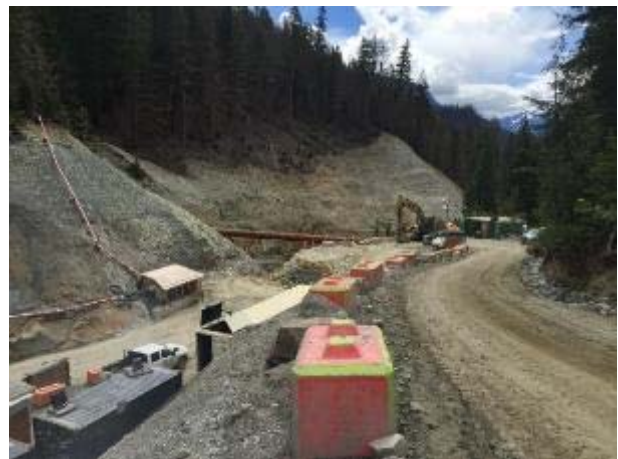
Photo 9 – Penstock excavation through Truckwash Creek (June 16, 2016).
