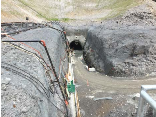
Photo 3 – Upper tunnel portal and BEBO wall (June 6, 2016).
