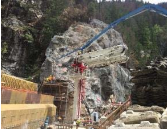
Photo 15 – Installation of placing boom for reinforced concrete works (June 15, 2016).
