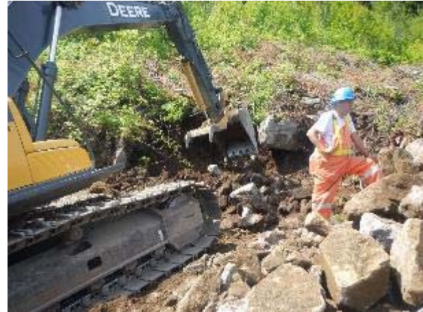
Photo 21 – Pole anchor excavations partially within 269a RVMA (June 7, 2016).
