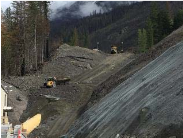
Photo 10 – Penstock slope above ULRHEF powerhouse (June 13, 2016).
