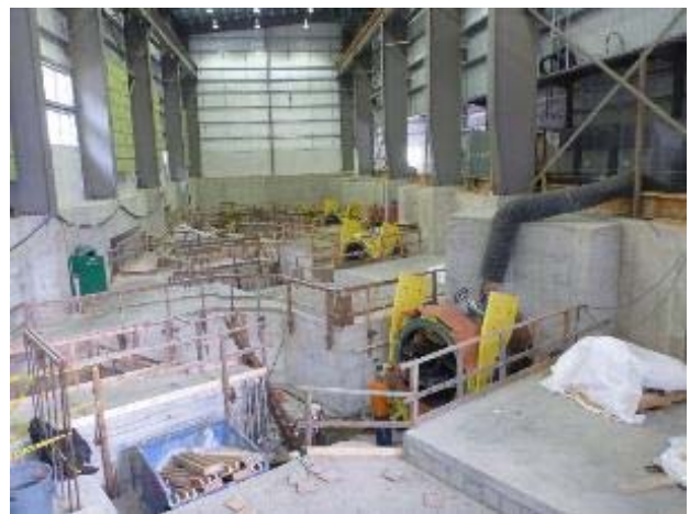
Photo 12 – Mechanical works in the ULRHEF powerhouse (June 8, 2016).
