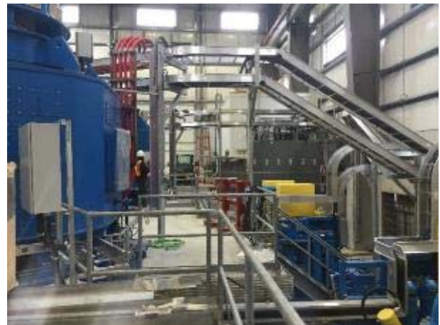
Photo 17 –Electrical component installation in BDRHEF powerhouse (June 15, 2016).
