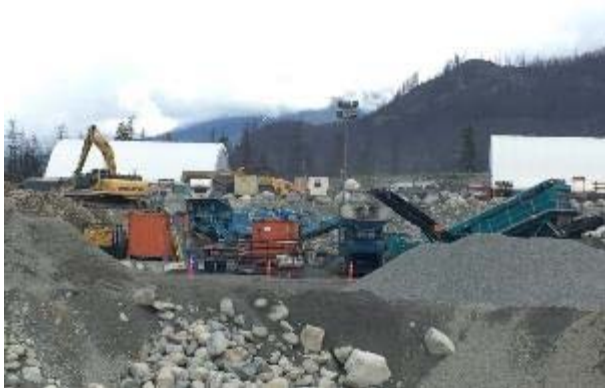
Photo 1 – Crusher and Screener at the KM38 laydown (June 15, 2016).
