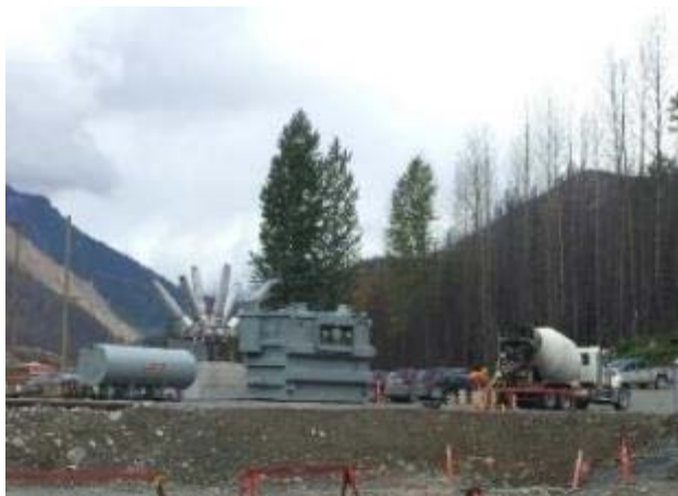
Photo 18– Concrete works at BDRHEF switchyard (June 15, 2016).
