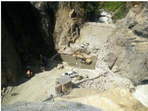
Photo 13 – Ground preparation for footings of Boulder Creek Intake structure (June 5, 2016).
