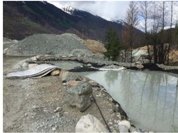
Photo 22 – BDRHEF Downstream Tunnel Portal settling ponds (May 29, 2016).
