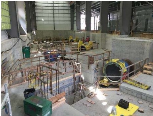
Photo 17 – Installation of turbine inlet valve at ULRHEF powerhouse (June 02, 2016).
