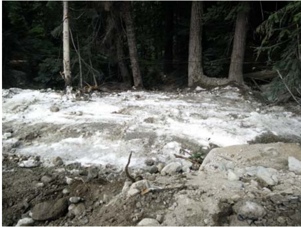
Photo 8 – Removal of sediment from Mountain Goat Winter Range (May 24, 2016).
