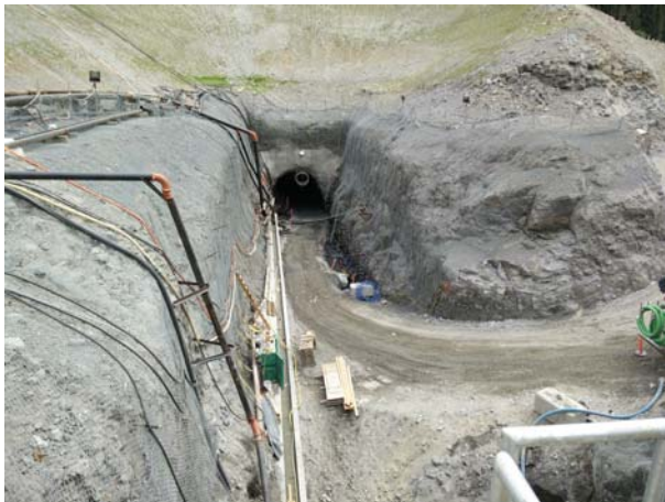
Photo 2 – Upstream Tunnel Portal and BEBO wall (May 23, 2016).
