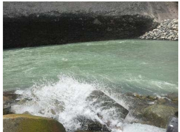
Photo 7 – Discharge of ULRHEF intake water treatment system (June 01, 2016).
