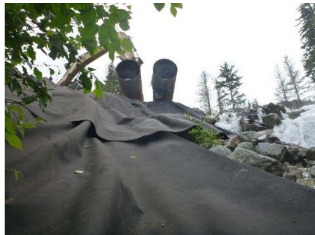
Photo 10 – Armoured outlet of Truckwash Creek bypass pipe outlet (June 02, 2016).
