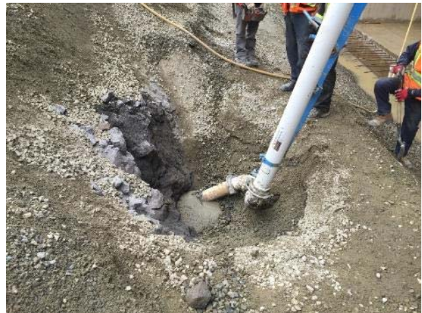
Photo 18 - Filling of ULRHEF tailrace depression (May 26, 2016).
