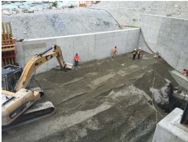
Photo 15 – Backfill and compaction of ULRHEF tailrace (May 27, 2016).
