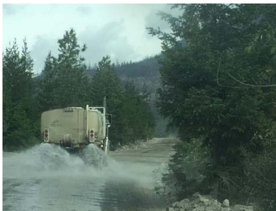
Photo 1 – CE water truck in use for dust suppression on the Lillooet River FSR (May 26, 2016).
