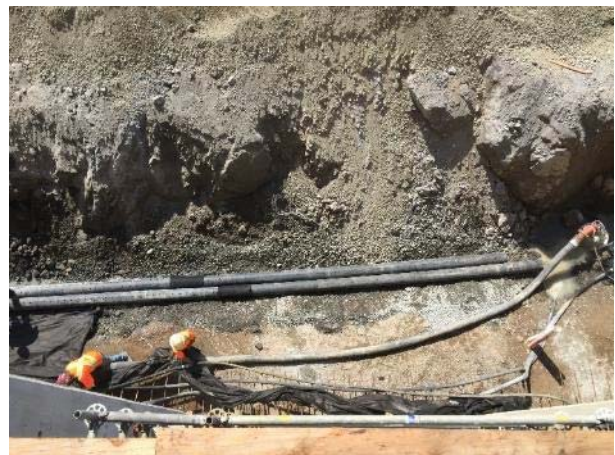
Photo 14 – Installation of perforated pipe at ULRHEF tailrace (May 25, 2016).
