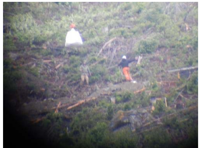
Photo 24 – Ground prep in Segment 15 (May 24, 2016).
