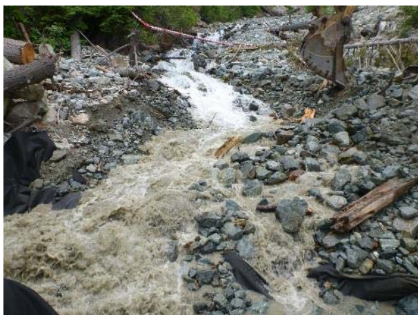
Photo 11 – Actively diverting Truckwash Creek (June 03, 2016).
