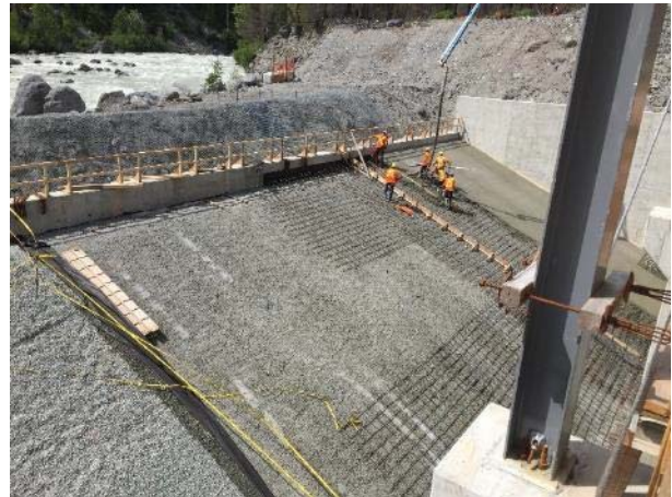
Photo 16 – Rebar, formwork, and concrete at ULRHEF tailrace (June 02, 2016).
