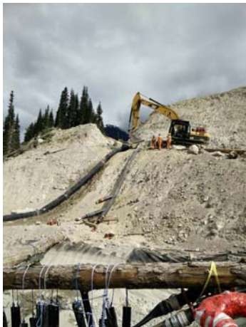
Photo 6 – Assembly and installation of 12” HDPE discharge line (May 23, 2016).
