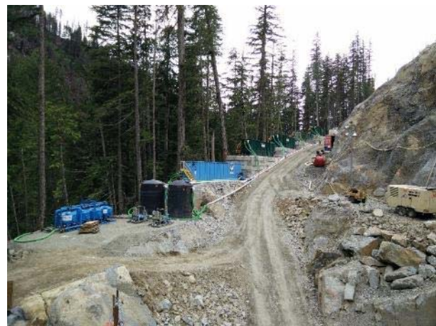
Photo 20 – Installation of water treatment system at Boulder Intake (May 23, 2016).
