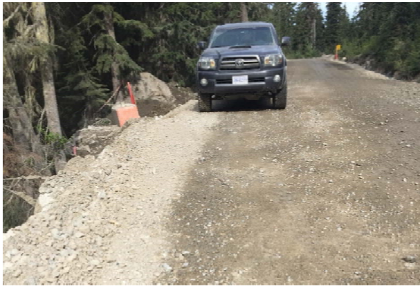
Photo 1– Dust suppression applied to control fugitive dust (May 15, 2016).
