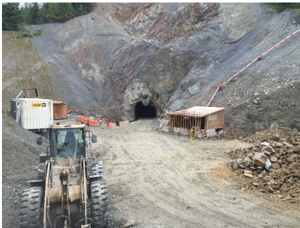
Photo 9 – Conditions and the lower tunnel portal entrance (May 18, 2016).
