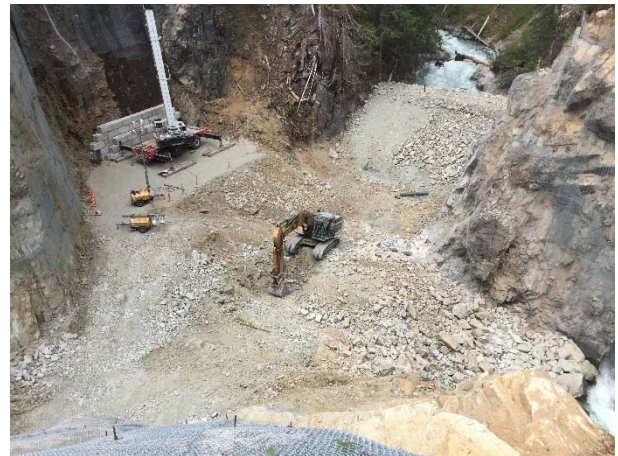
Photo 20 – Bulk excavation of the intake footprint (May 17, 2016).
