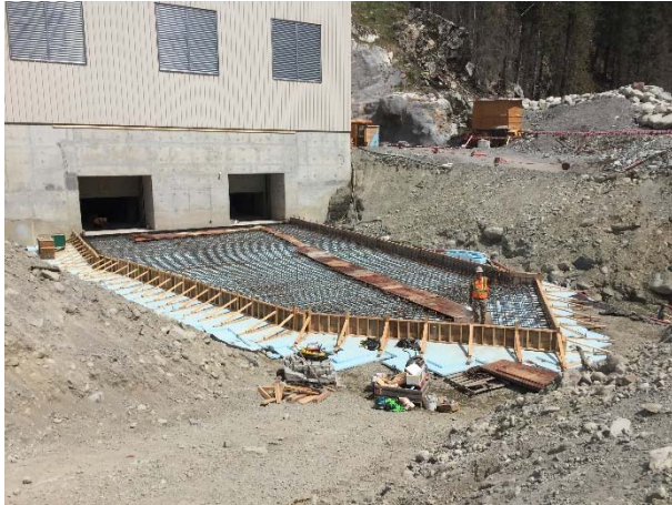
Photo 21 – Rebar and formwork installed at the BDRHEF powerhouse tailrace (May 17, 2016).
