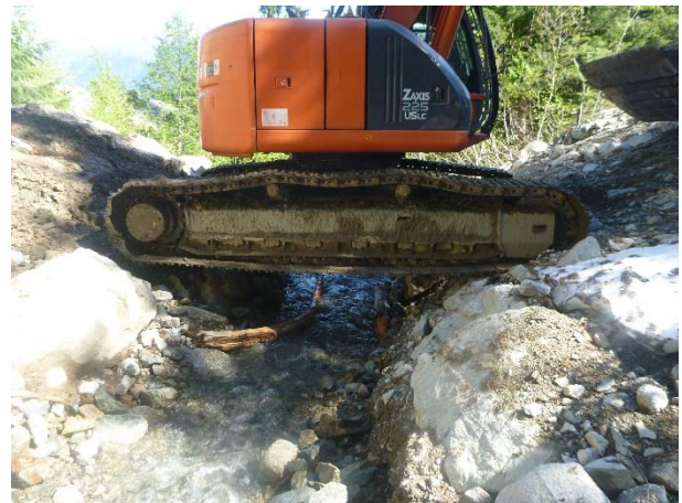
Photo 26 – Excavator performing one-time crossing of stream 272a (Segment 11; May 10, 2016).
