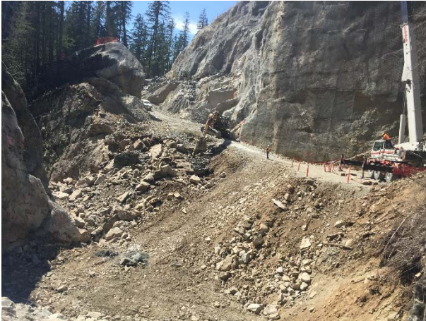
Photo 17 – Excavating rock following a blast at the BDRHEF intake (May 14, 2016).
