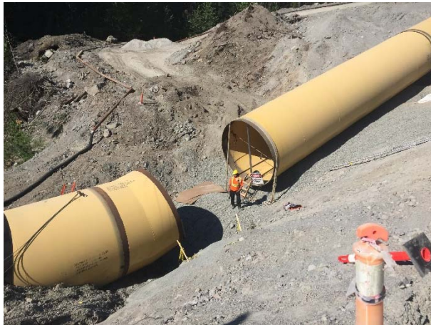
Photo 11– Welding penstock near the ASTR-03 crossing (May 14, 2016).
