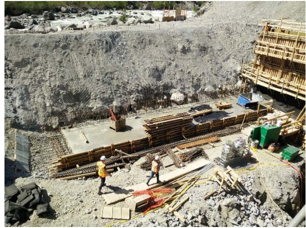
Photo 10 – Rebar and form work for the tailrace at ULHEF powerhouse (May 7, 2016).
