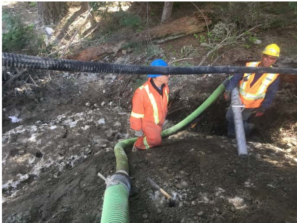
Photo 7– Removal of snow and sediment from Mountain Goat Winter Range via vacuum truck (May 4, 2016).
