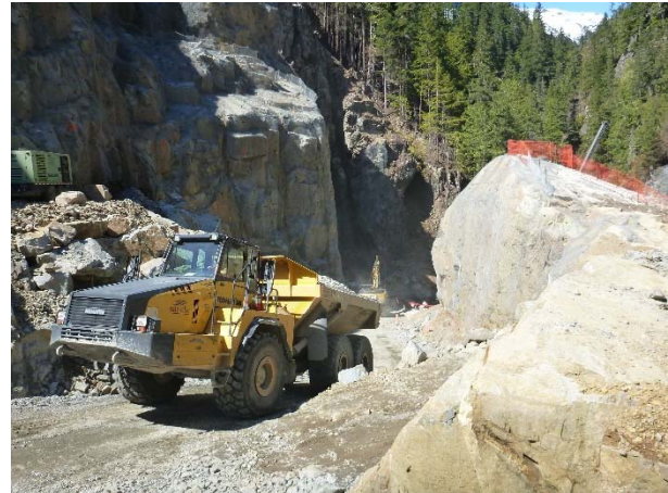
Photo 14 – Hauling material from the bulk excavation of the intake footprint (May 5, 2016).
