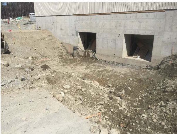
Photo 15 – Start of excavation of the BDRHEF powerhouse tailrace (April 30, 2016).
