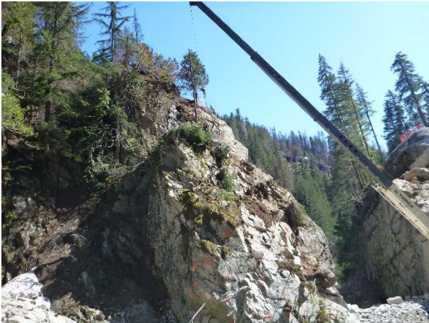
Photo 13 – Rock scaling and consolidation work above the future sluiceway location (May 5, 2016).
