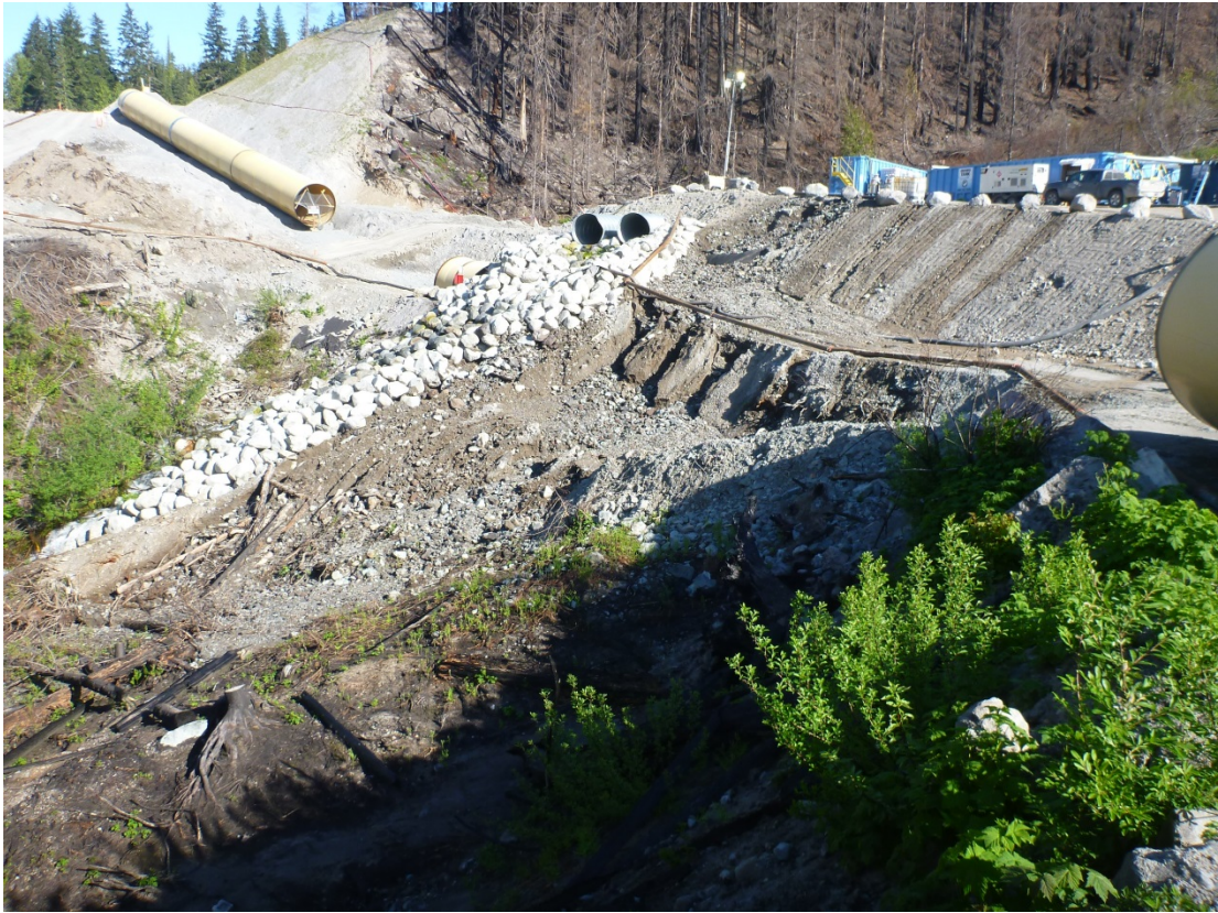
3. Extend of the erosion as seen daytime the next day.
