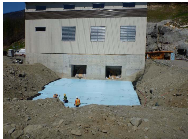
Photo 16 – Installing sheet foam at the base to the tailrace (May 5, 2016).
