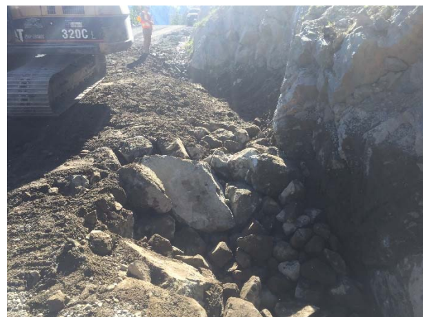
Photo 12 – BDRHEF intake access road ditch maintenance and culvert repairs (May 1, 2016).
