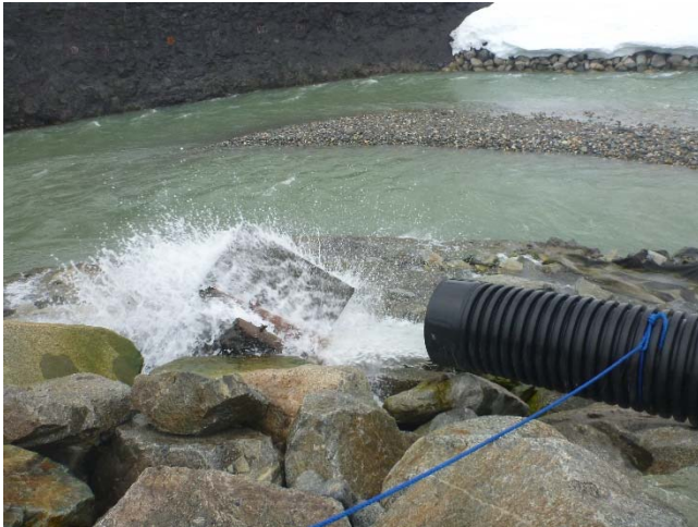
Photo 7 – Discharge of ULRHEF upstream tunnel water treatment system (April 16, 2016).
