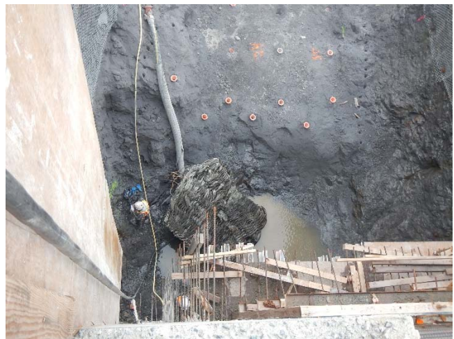
Photo 4 – Blasting at the BEBO wall (April 17, 2016).
