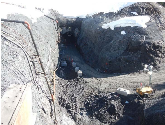
Photo 3 – ULR Upstream tunnel portal and BEBO wall excavation (April 10, 2016).
