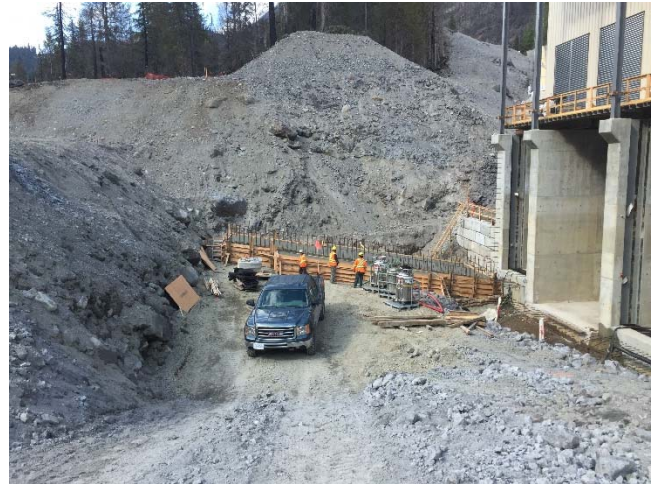
Photo 11 – Tailrace footing at ULRHEF powerhouse behind the natural earth berm (April 21, 2014).
