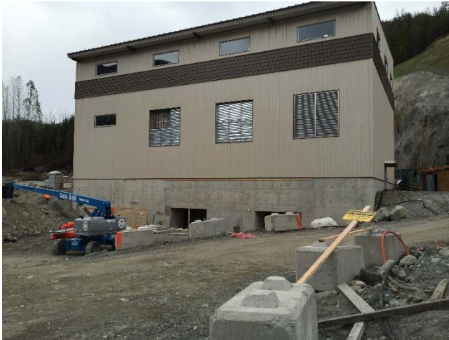
Photo 14 – Current conditions at the BDRHEF powerhouse (April 21, 2016).
