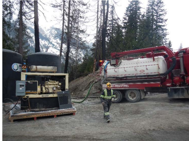
Photo 9 – Vacuum truck cleaning sediment from the active water treatment system along the penstock access road (April 15, 2016).
