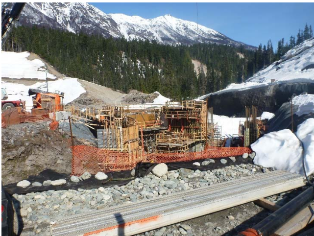
Photo 5 – Rebar, formwork, and concrete works at the ULHEF intake (April 18, 2016).
