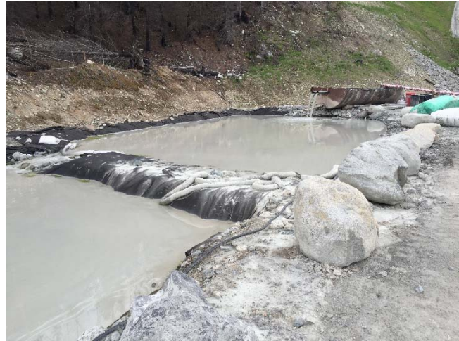
Photo 15 – BDRHEF downstream portal settling ponds (April 21, 2016).
