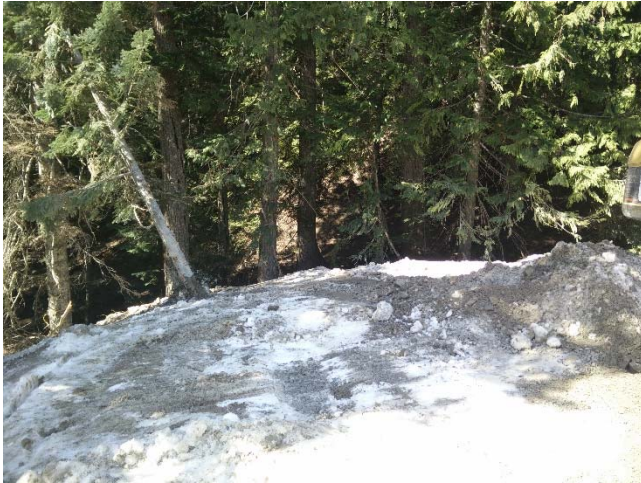
Photo 8 – Removal of snow and sediment from Mountain Goat replacement area (April 19, 2016).
