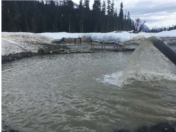
Photo 7 – Dewatering of upper portal water into treatment system (April 2, 2016).
