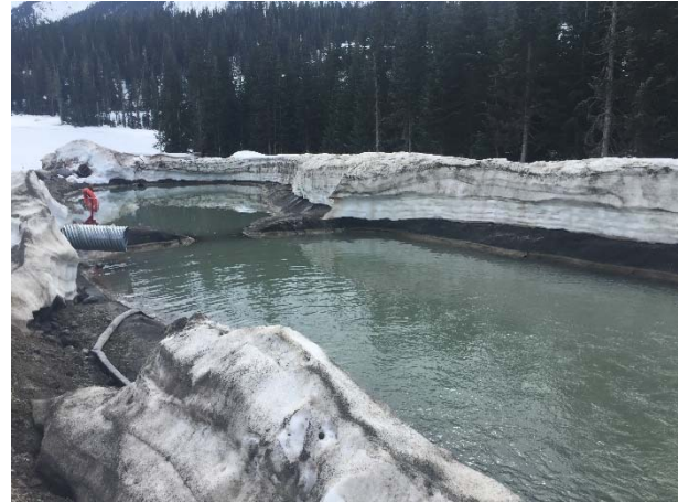
Photo 8 – Pond 6 and 7 of upper tunnel water treatment system (April 2, 2016).
