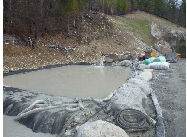
Photo 14 – BDRHEF downstream portal settling ponds (April 04, 2016).
