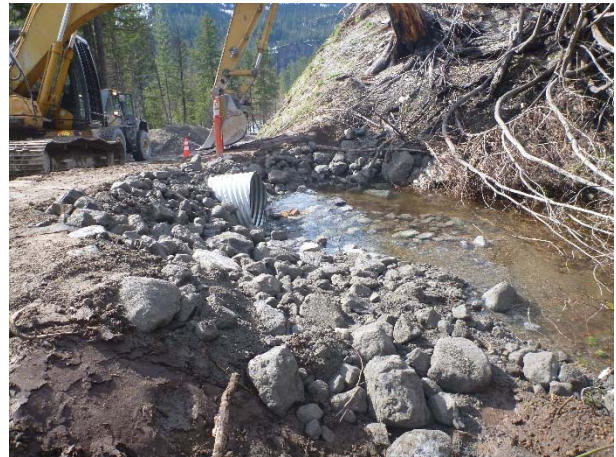
Photo 4 – KM43 culvert repair completed (April 7, 2016).
