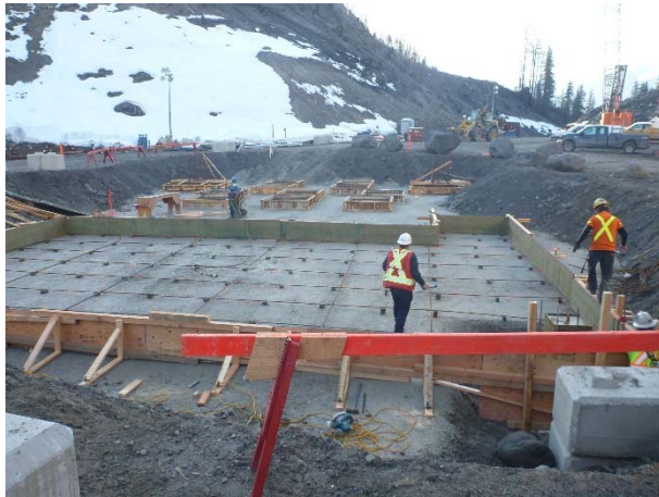
Photo 11 – Installation of formwork and rebar for the powerhouse switch yard (April 8, 2016).
