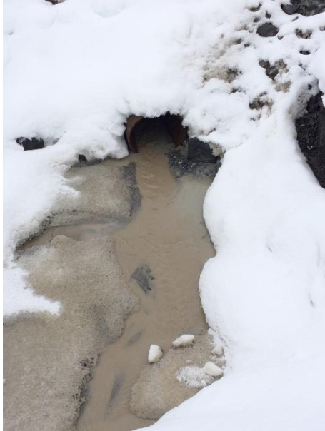
Photo 1 – Site discharge at KM49 being directed to the Lillooet River was over-range on the 2020we turbidity meter yesterday. (March 15, 2016)
