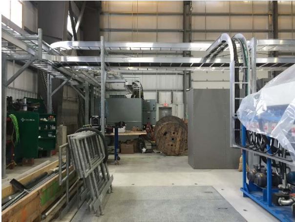
Photo 13 – Conditions inside the powerhouse (March 24, 2016).
