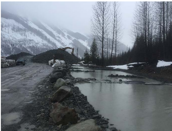
Photo 15 – BDRHEF sediment ponds (March 23, 2016).
