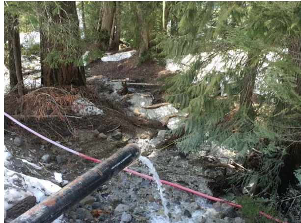
Photo 8 – Water continues to discharge from the ULRHEF downstream tunnel infiltration ponds despite the treatment system being active. The IEM is under the understanding that an upgraded water treatment system is on order (March 26, 2016).
