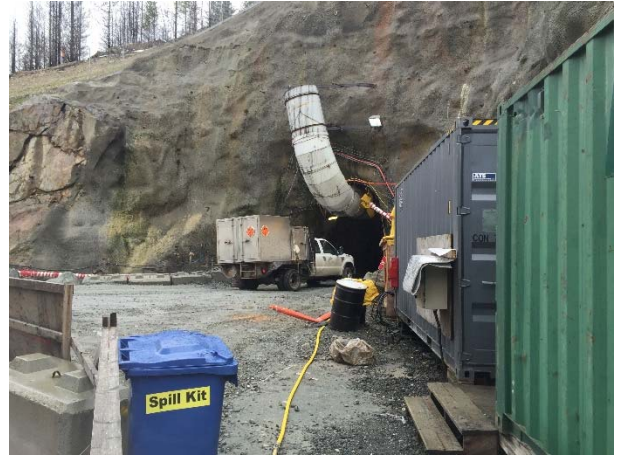
Photo 14 – BDRHEF downstream tunnel portal (March 24, 2016).
