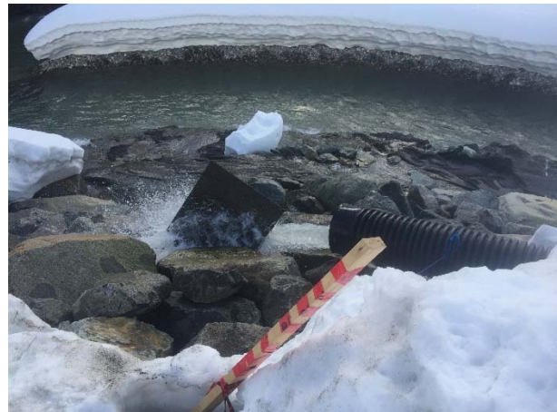
Photo 4 – Discharge from ULRHEF sediment basins to Lillooet River during canopy tube installation (drilling) in the tunnel (March 22, 2016).
