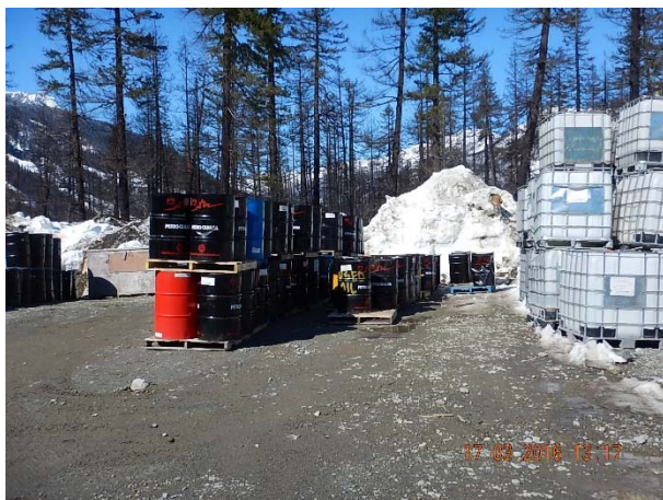
Photo 1 – Hazardous materials stored at the KM38 laydown stored temporarily prior to off-site disposal (March 17, 2016).
