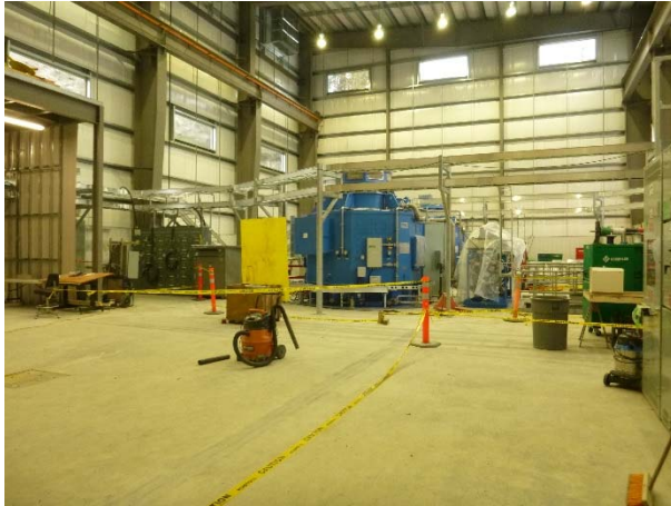
Photo 12 – Current conditions inside the BDRHEF powerhouse (March 6, 2016).
