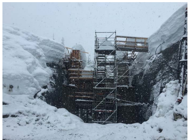
Photo 6 – ULRHEF intake structure work remains on hold (Mach 12, 2016).
