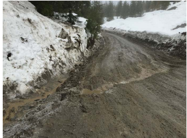
Photo 10 – Cross-ditching installed to direct road runoff to the ditch line (March 6, 2016).
