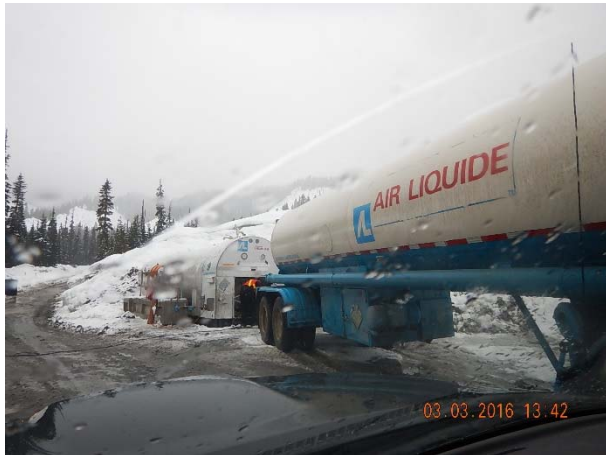
Photo 3 – Delivery of the bulk CO 2 system to support the water treatment system at the ULRHEF intake (March 3, 2016).
