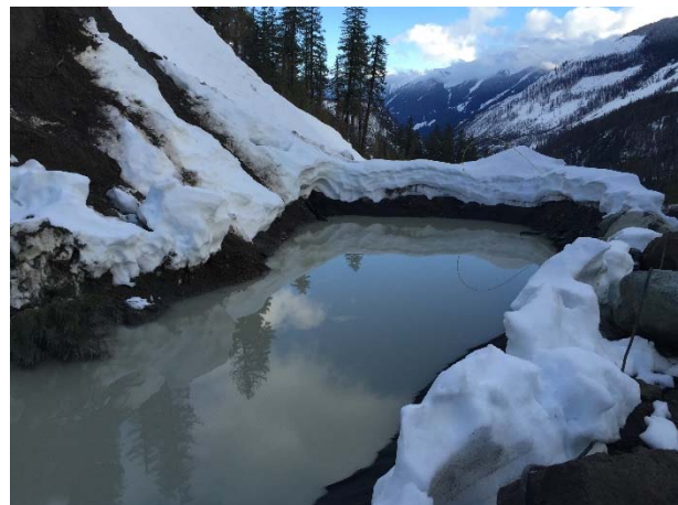
Photo 8 – ULRHEF downstream tunnel infiltration ponds continue to outlet despite the treatment system being active (March 7, 2016).
