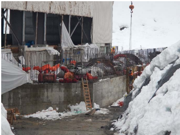
Photo 11 – Current conditions at the ULRHEF powerhouse (March 8, 2016).
