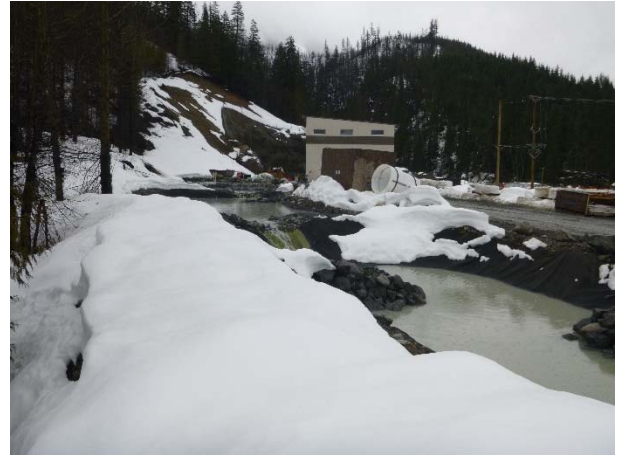
Photo 13 – BDRHEF downstream tunnel portal, powerhouse, and settling ponds (March 6, 2016).
