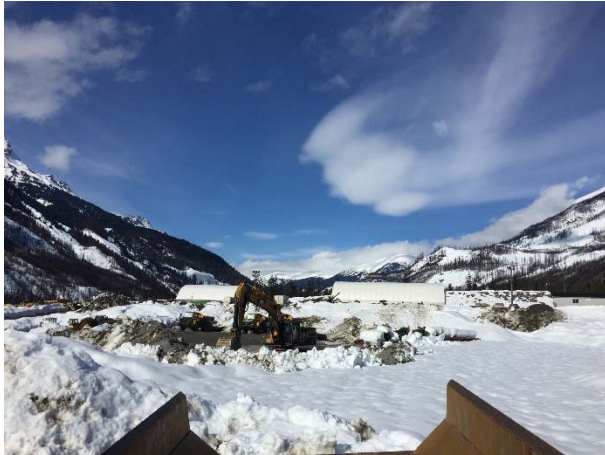
Photo 1 – Current conditions at the KM38 crusher pad (February 27, 2016).
