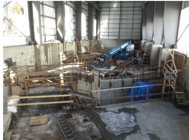
Photo 14 – Current conditions inside the ULRHEF powerhouse (February 27, 2016).
