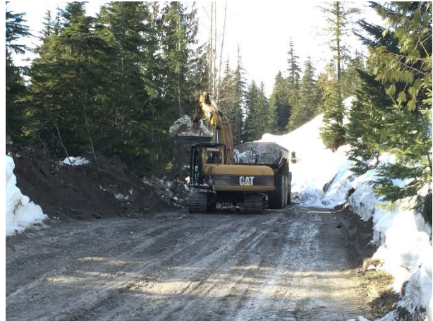
Photo 10 – Ditching of the downstream tunnel portal access road (February 27, 2016).
