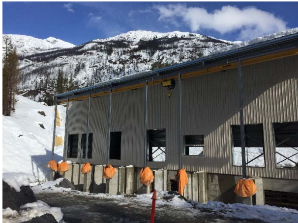
Photo 13 – Current conditions at the ULRHEF powerhouse (February 27, 2016).
