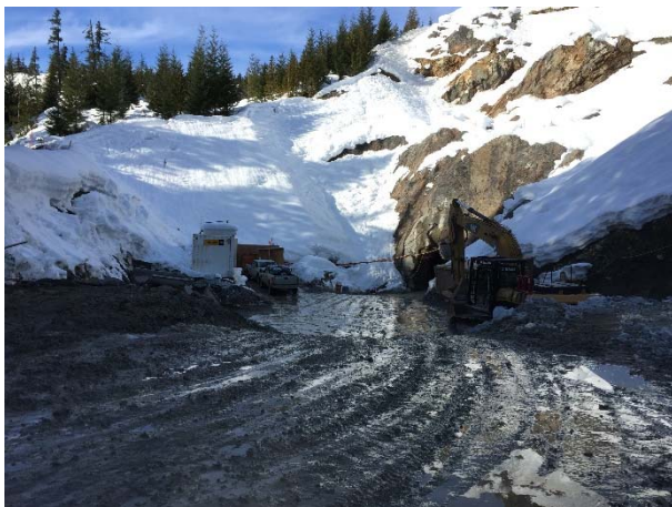
Photo 11 – Current conditions at the downstream tunnel portal (February 27, 2016).
