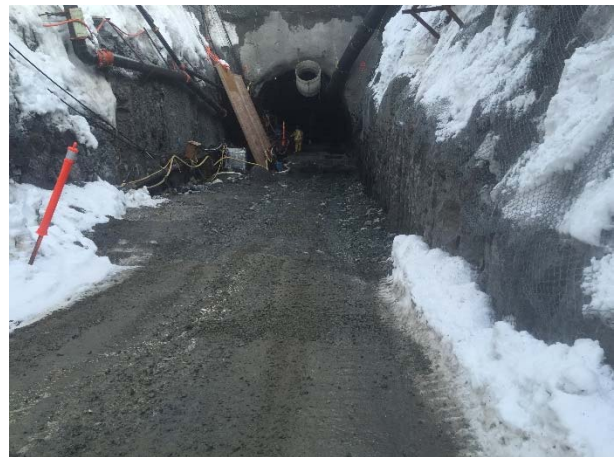
Photo 8 – Current conditions at the ULRHEF upstream tunnel portal access road (February 24, 2016).
