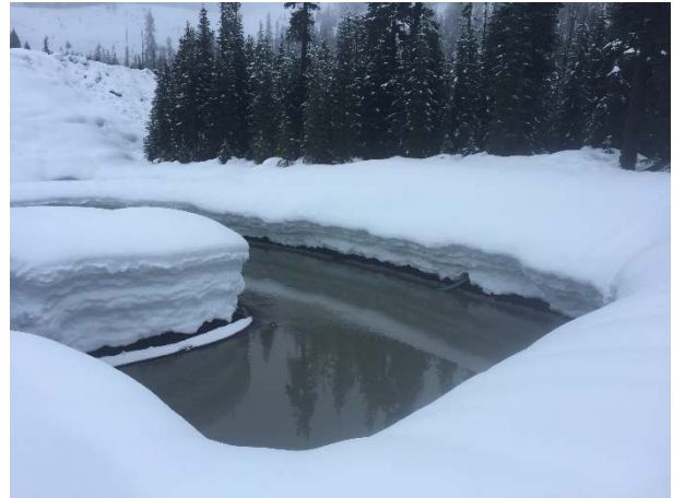
Photo 6 – The second cell of the ULRHEF sediment basins at the discharge of the primary treatment system. (February 14, 2016).
