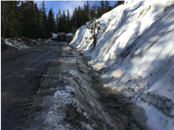
Photo 9 – Ditching of the downstream tunnel portal access road (February 27, 2016).
