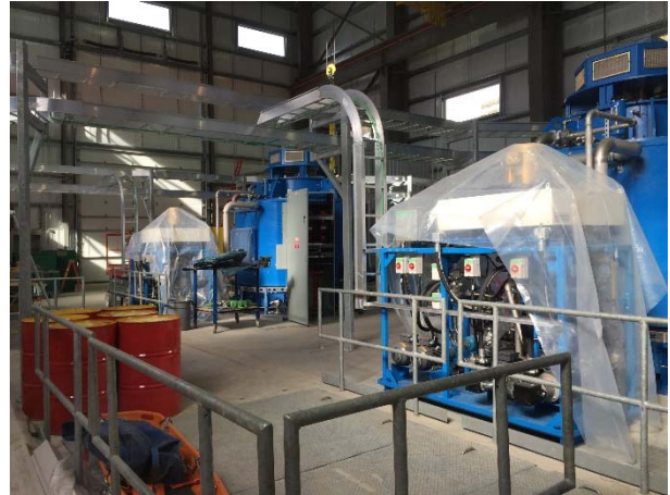
Photo 16 – Electrical component installation inside BDRHEF Powerhouse (February 27, 2016).
