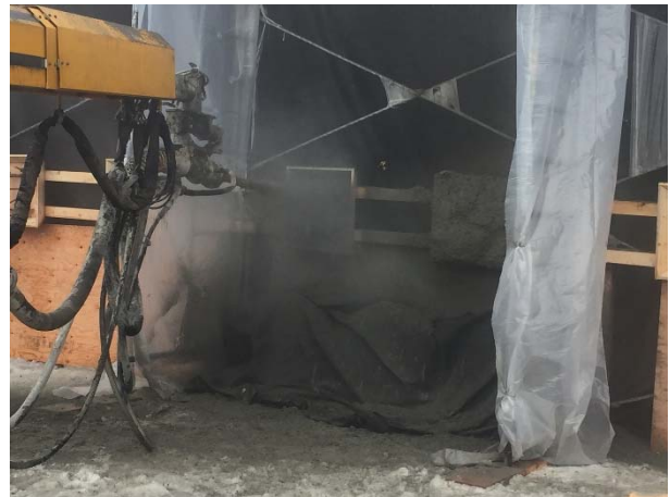
Photo 18 – Shotcrete testing station at BDRHEF downstream tunnel portal, (February 18, 2016).
