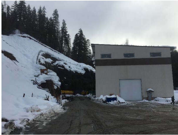
Photo 9 – Current conditions at the BDRHEF tunnel portal and powerhouse (February 9, 2016).
