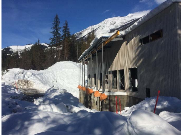
Photo 7 – Current conditions at the ULRHEF powerhouse (February 8, 2016).
