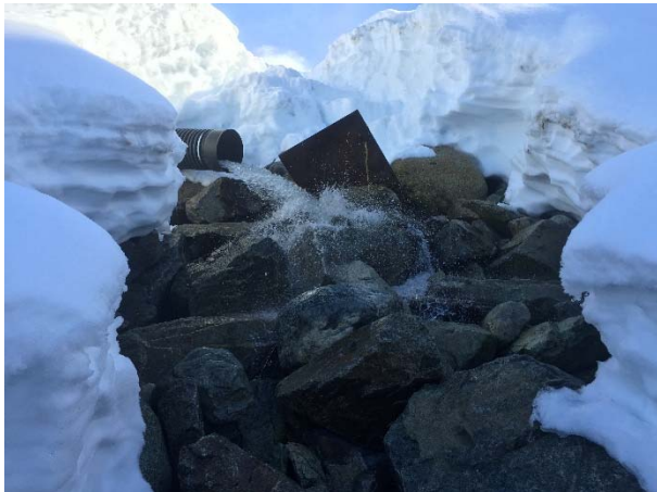
Photo 4 – Discharge from ULRHEF sediment basins to Lillooet River during mucking in the tunnel (February 8, 2015).
