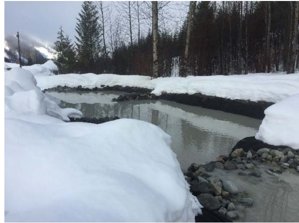
Photo 10 – BDRHEF downstream portal settling ponds (February 9, 2016).
