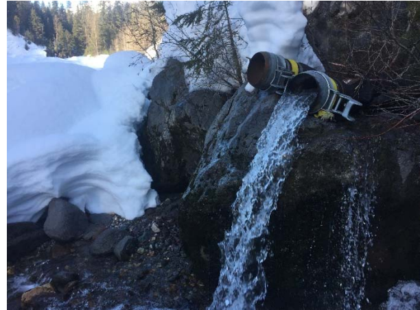
Photo 8 – ULRHEF powerhouse seepage water dewatered to the Lillooet River (February 8, 2016).
