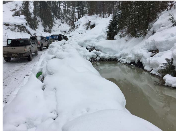
Photo 6 – ULRHEF downstream tunnel infiltration ponds (February 3, 2016).
