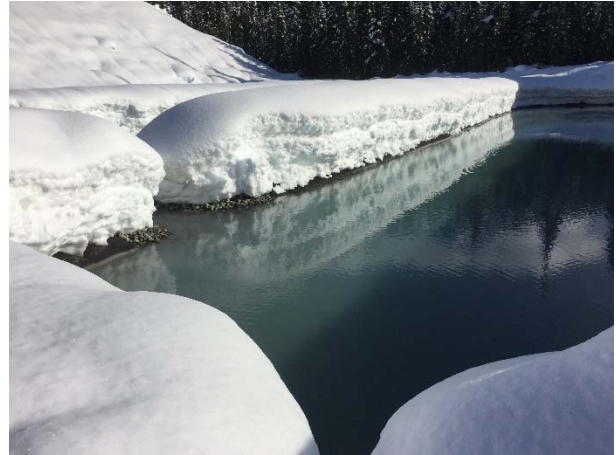
Photo 3 – The second cell of the ULRHEF sediment basins following a blast in the tunnel; water was visibly clear downstream of treatment system (February 8, 2015).
