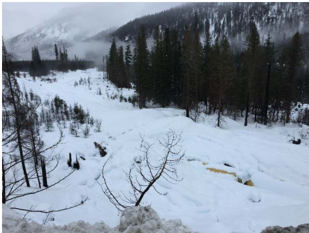
Photo 17 – ULRHEF Penstock shutdown for winter (January 29, 2016).
