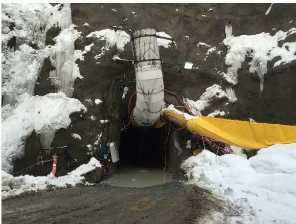
Photo 20 – Current conditions at BDRHEF downstream Tunnel Portal (January 26, 2016).
