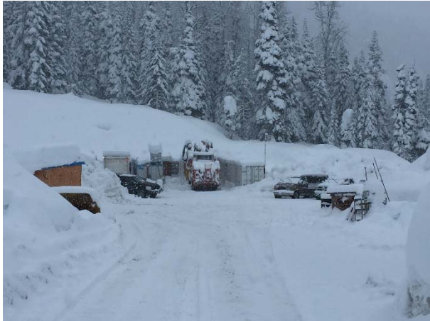
Photo 9 – Laydown area at KM49 of the Lillooet River FSR for ULRHEF grouting works (January 26, 2016).
