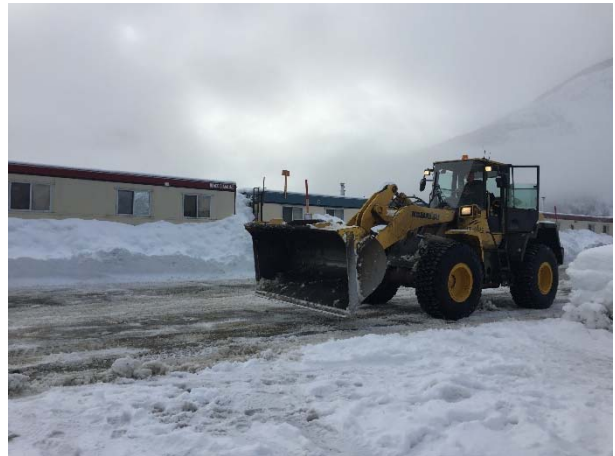
Photo 4 – Snow removal on pad 3 at the construction camp (January 26, 2016).
