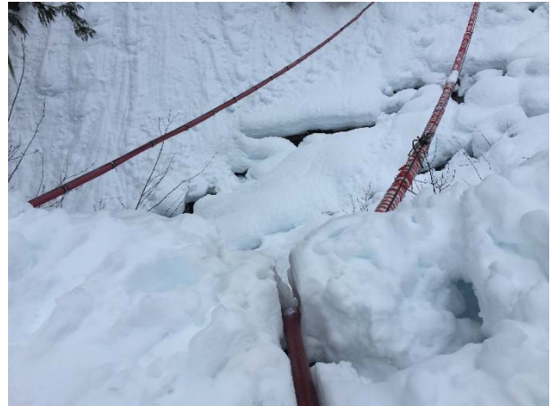
Photo 16 – Outlet of the treatment system into Truckwash Creek (January 27, 2016).
