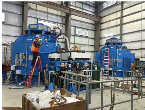
Photo 21 – Mechanical and electrical component installation inside BDRHEF Powerhouse (January 26, 2016).
