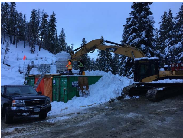
Photo 5 – Snow removal off buildings at the downstream tunnel portal laydown (January 26, 2016).
