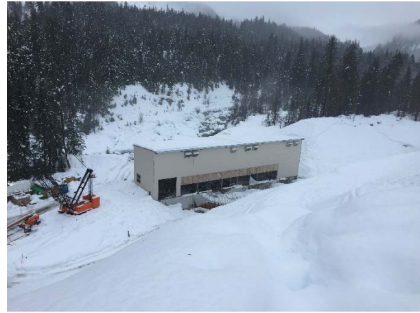
Photo 19 – ULRHEF powerhouse superstructure construction suspended until April 2016 (January 27, 2016).
