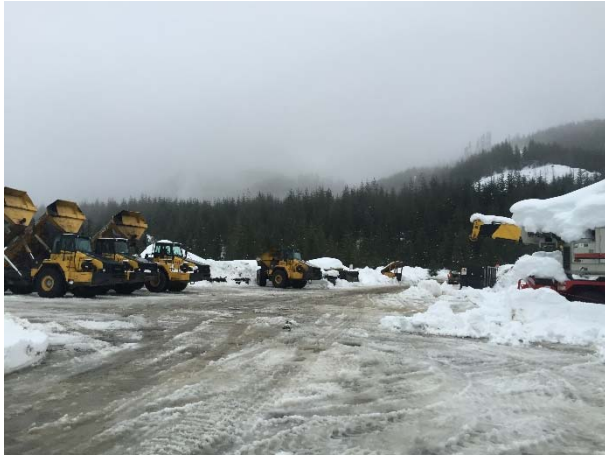
Photo 1 – Current conditions of the crusher pad at the KM38 laydown (January 27, 2016).
