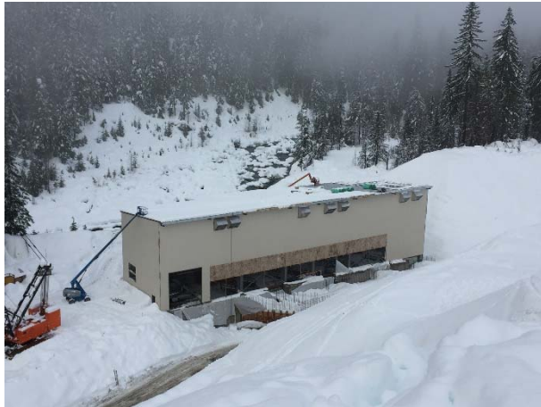
Photo 18 – ULRHEF powerhouse superstructure construction (January 19, 2016).
