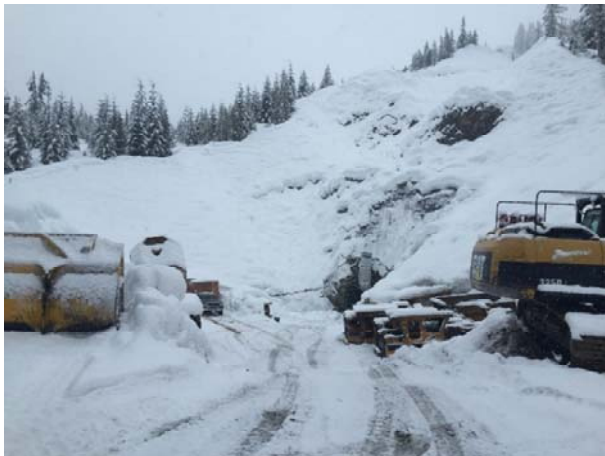
Photo 11 – Current conditions of ULRHEF Downstream Portal (January 26, 2016).
