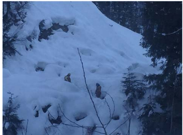
Photo 8 – Repairing the piping system at the primary ULRHEF downstream tunnel infiltration ponds so water can be direct to the second set of infiltration ponds (January 9, 2015).
