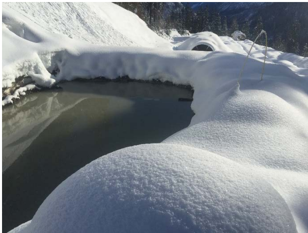
Photo 7 – Water discharging from the primary infiltration ponds at the ULRHEF downstream tunnel is no longer infiltrating in a vegetated area and is flowing over a steep bank at the toe of the penstock fill (January 8, 2016).
