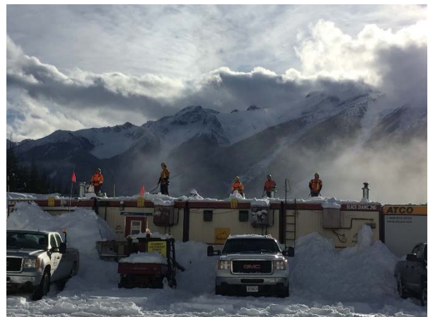
Photo 4 – Removing snow from the roofs at the ULHP camp following heavy snowfall (January 13).
