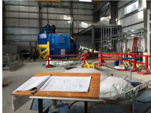
Photo 13 – Preparing the generators for installation inside the BDRHEF powerhouse. (January 13, 2016).
