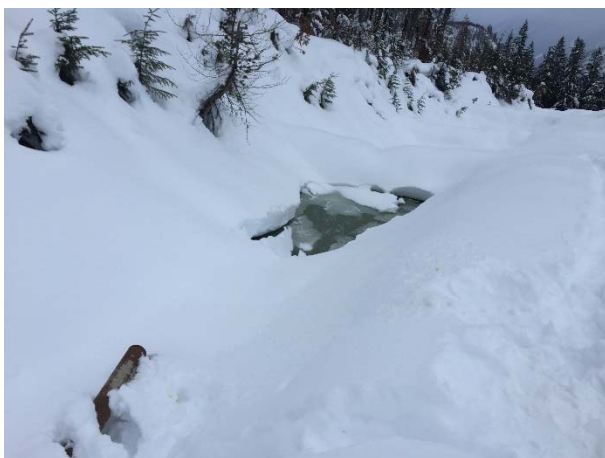
Photo 9 –ULRHEF downstream tunnel seepage and process water being directed to the second set of infiltration ponds (January 11, 2016).
