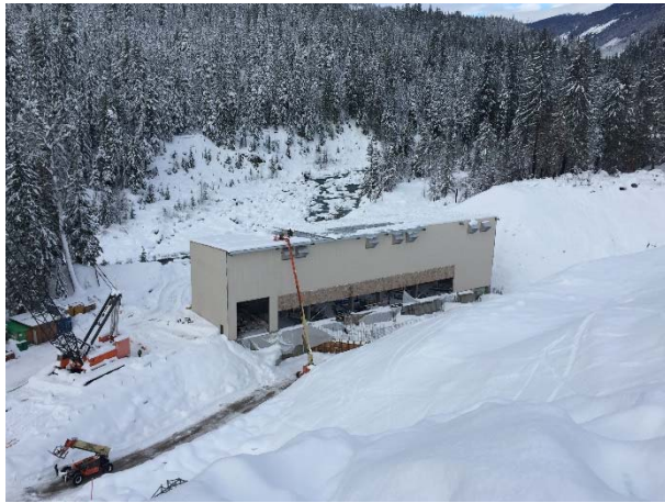
Photo 10 – ULRHEF powerhouse construction (January 7, 2016).
