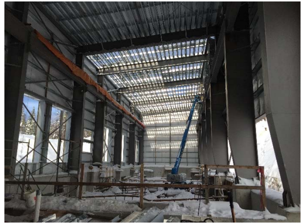
Photo 11 – ULRHEF powerhouse construction (January 13, 2016).
