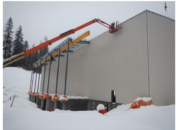
Photo 7 – ULRHEF powerhouse construction (December 13, 2015).
