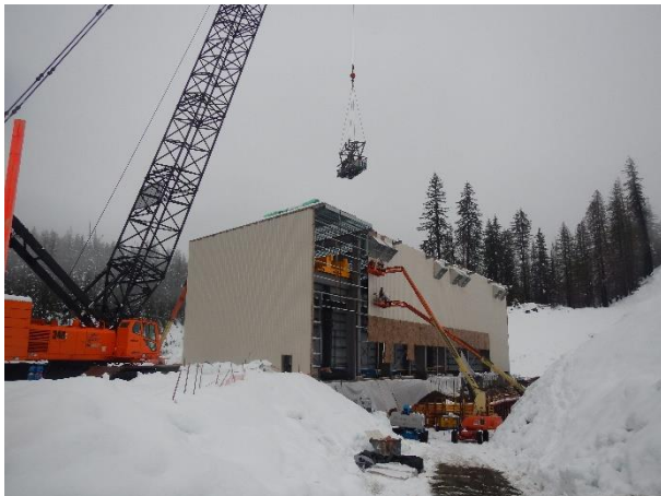
Photo 6 – ULRHEF powerhouse construction (December 13, 2015).
