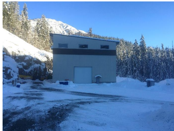
Photo 9 – Conditions at the BDRHEF tunnel portal and powerhouse during Christmas shutdown (December 30, 2015).
