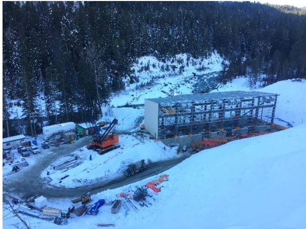
Photo 5 – Current conditions at the ULRHEF powerhouse (November 26, 2015).
