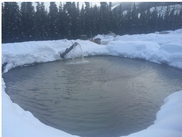
Photo 1 – Seepage water pumped to ULRHEF intake sediment basins during grout injection (December 9, 2015).
