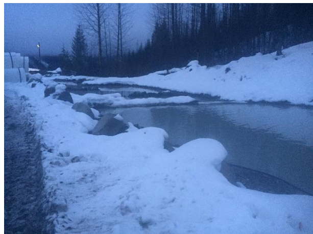
Photo 8 – BDRHEF downstream portal settling ponds (December 9, 2015).
