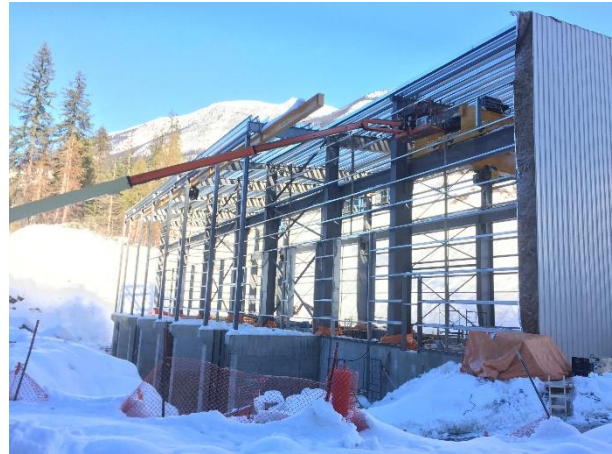
Photo 6 – Current conditions at the ULRHEF powerhouse (November 27, 2015).
