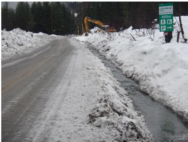
Photo 1 – Maintenance of ditch at KM42 of the Lillooet River FSR (December 4, 2015)
