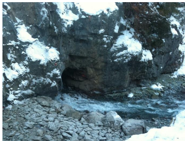
Photo 12 – Partial downstream cofferdam constructed at BDRHEF Intake (November 30, 2015).
