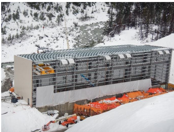
Photo 9 – Current conditions at the ULRHEF powerhouse (December 4, 2015).
