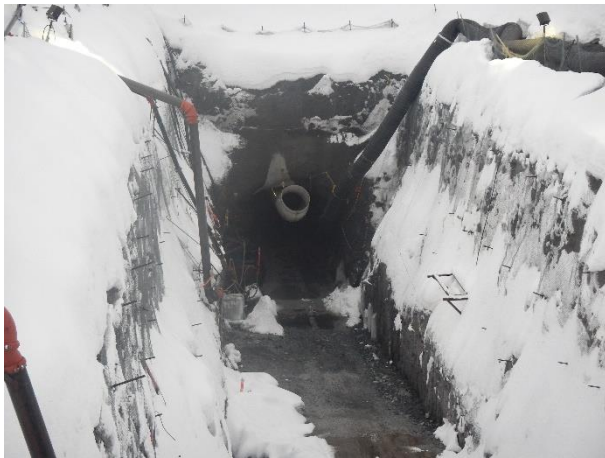
Photo 3 – ULRHEF upstream tunnel portal (December 2, 2015).
