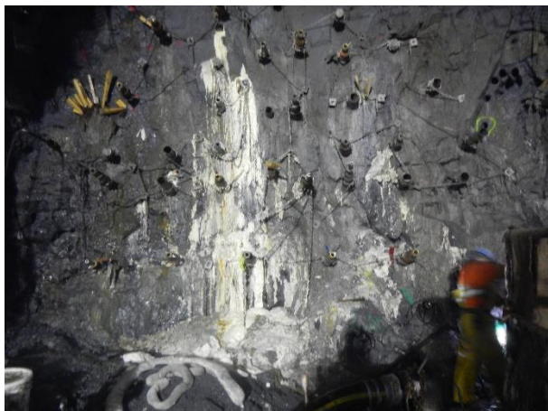
Photo 7 – Grouting at the face of ULRHEF upstream tunnel portal (December 5, 2015).
