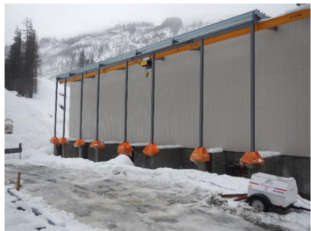
Photo 10 – Current conditions at the ULRHEF powerhouse (December 4, 2015).
