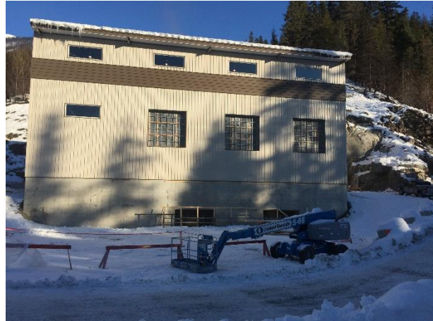
Photo 29 – BDRHEF powerhouse structure (November 27, 2015).
