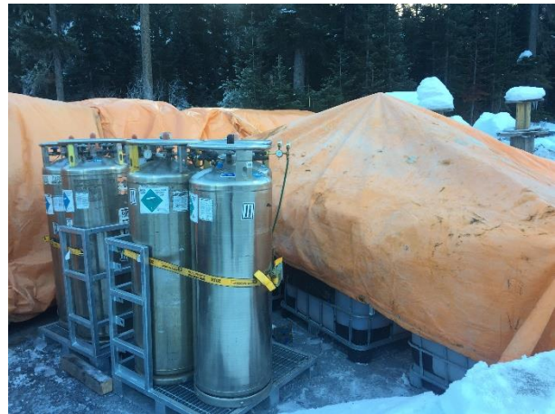
Photo 2 – Active water treatment system with CO 2 tanks at ULRHEF intake (November 28, 2015).
