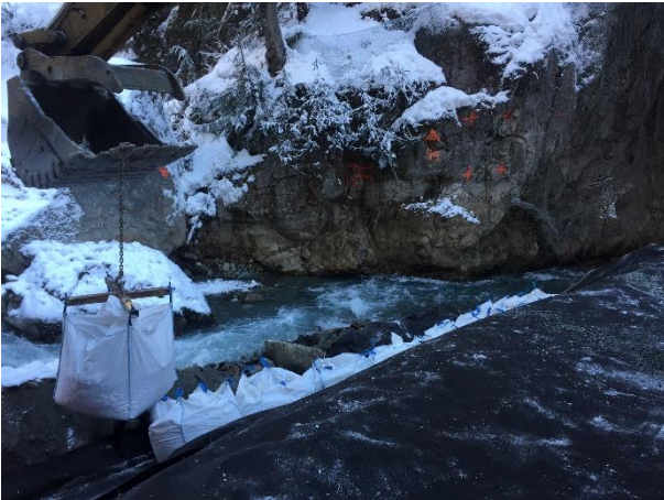
Photo 18 – Excavator placing mega-bags in trench for upstream cofferdam construction (November 24, 2015).
