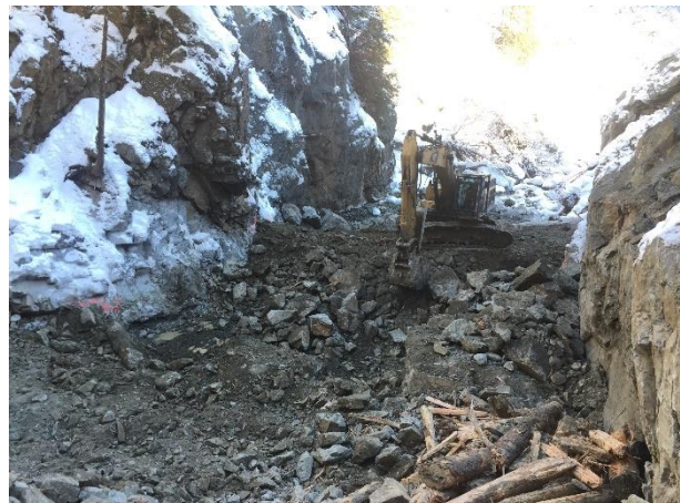
Photo 23 – Final stage of downstream cofferdam construction (November 28, 2015).
