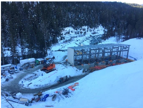
Photo 11 – Current conditions at the ULRHEF powerhouse (November 26, 2015).
