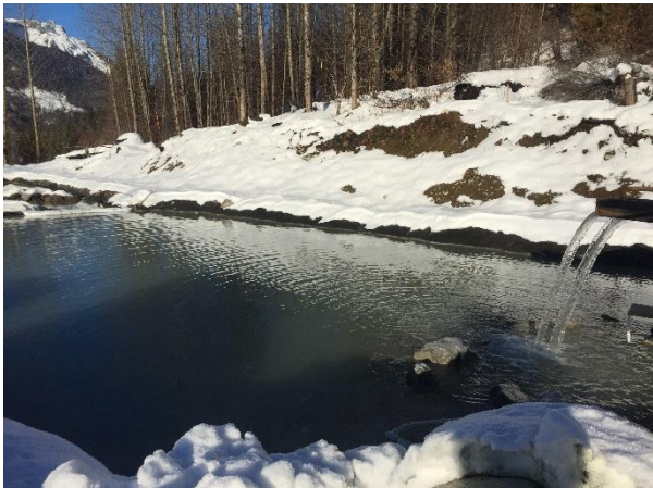
Photo 30 – BDRHEF tunnel portal settling ponds (November 27, 2015).
