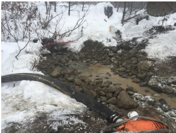
Photo 7 – Backfill of sump completed and natural flows restored to ASTR-04 (November 23, 2015).
