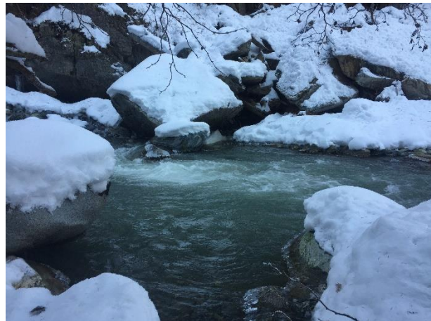
Photo 27 – Flows clearing in Boulder Creek at the water quality compliance station following downstream cofferdam construction (November 28, 2015).
