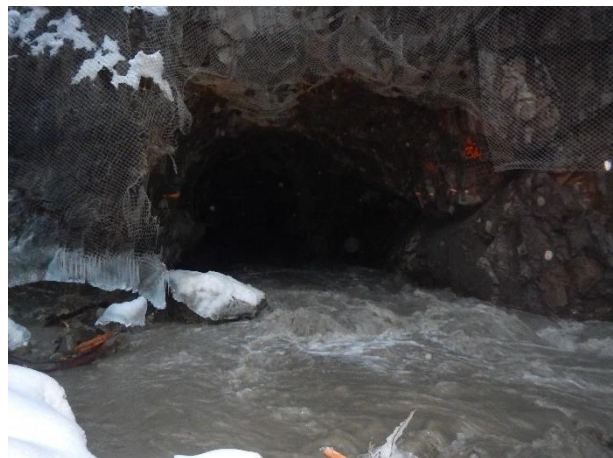
Photo 17 – Diversion tunnel exit following plug removal and creek diversion (November 22, 2015).
