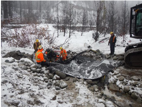
Photo 9 – Replacement of impermeable geotextile membrane to prevent subsurface flow (November 23, 2015).
