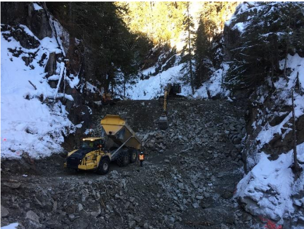
Photo 20 – Final stage of upstream cofferdam construction (November 26, 2015).
