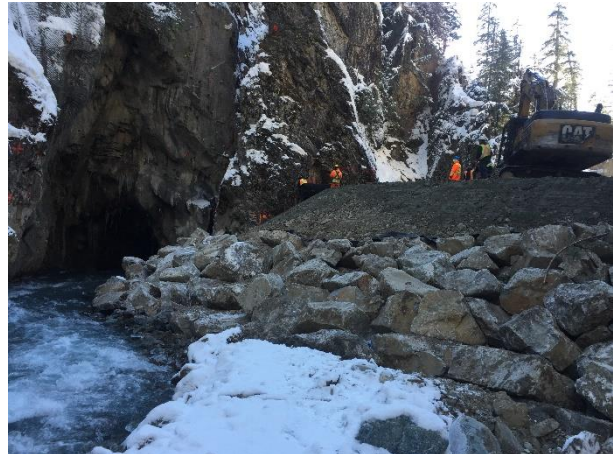
Photo 19 – The upstream cofferdam near completion with rock armouring (November 25, 2015).
