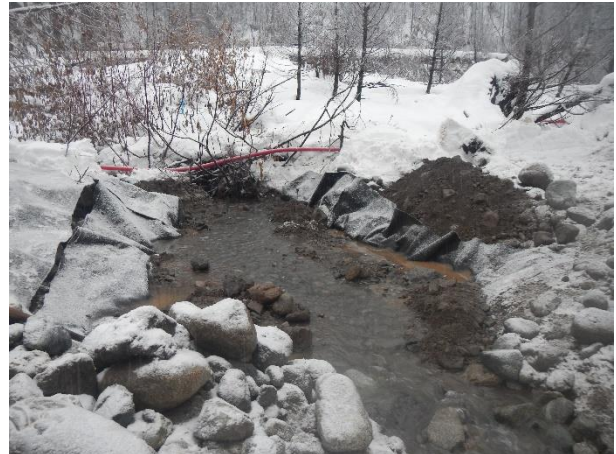
Photo 10 – Natural flows restored following membrane replacement and sump backfill (November 23, 2015).
