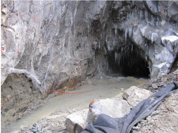
Photo 13 – Upstream cofferdam with geomembrane and rock armouring (November 22, 2015).
