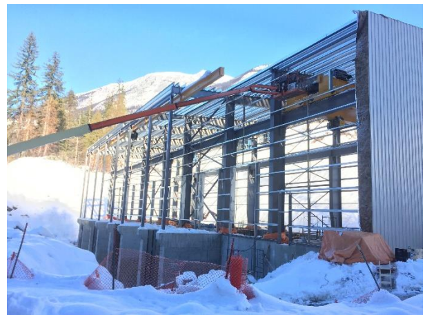
Photo 12 – Current conditions at the ULRHEF powerhouse (November 27, 2015).
