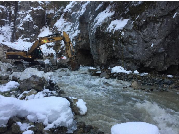
Photo 22 – Instream works for downstream cofferdam construction (November 28, 2015).
