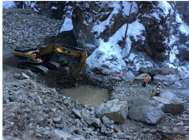
Photo 21 – Test pit below upstream cofferdam to assess bedrock conditions (November 27, 2015).
