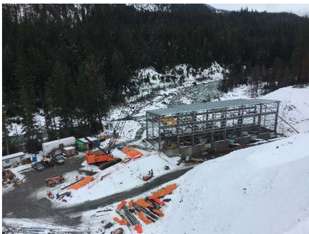
Photo 7 – Current conditions at the ULRHEF powerhouse (November 15, 2015).
