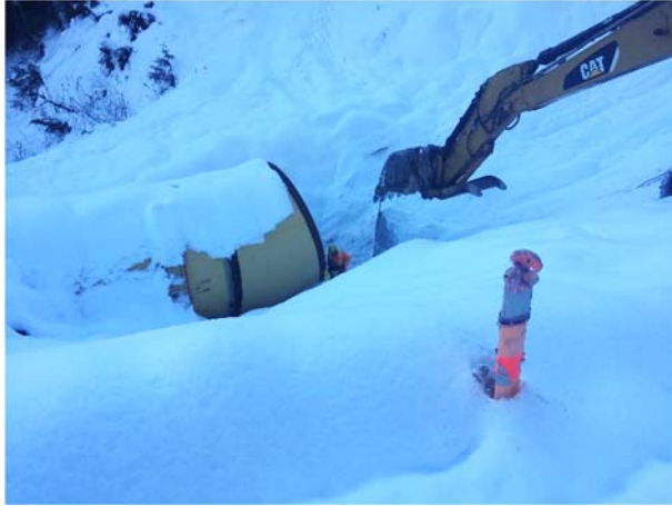
Photo 5 – Fence installed at end of penstock for winterization (November 20, 2015).
