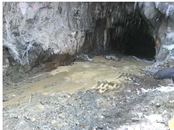
Photo 12 – Flow introduced slowly to the BDRHEF intake diversion tunnel (November 21, 2015).
