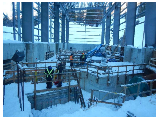
Photo 8 – ULRHEF powerhouse superstructure construction (November 20, 2015).
