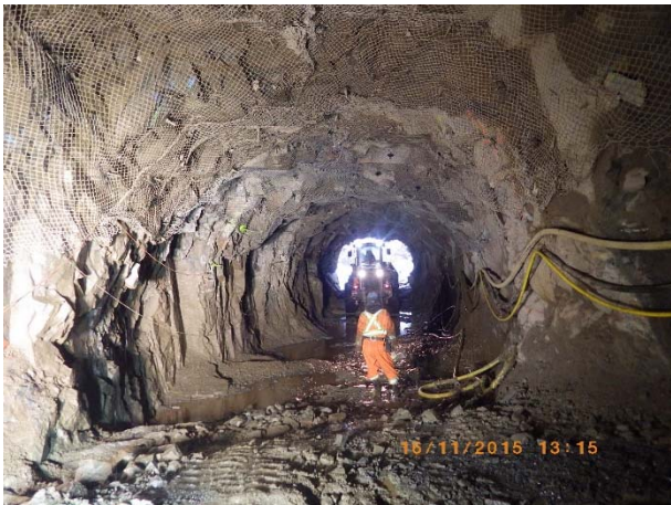
Photo 9 – Cleaning BDRHEF intake diversion tunnel prior to diversion works (November 17, 2015).
