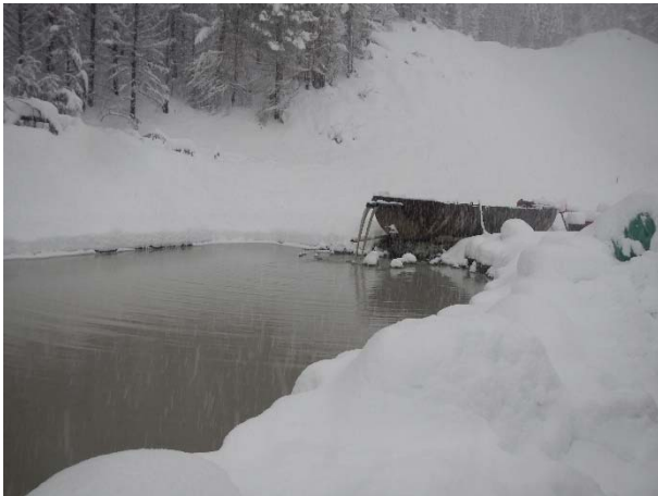
Photo 18 – BDRHEF downstream portal settling ponds (November 17, 2015).
