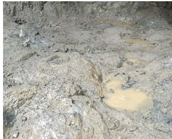
Photo 10 – BDRHEF intake diversion tunnel floor during inspection (November 18, 2015).
