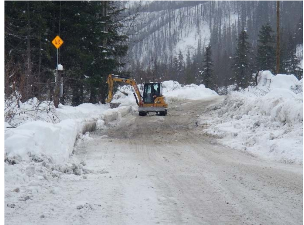
Photo 2 – Ditch maintenance at KM 41.75 on the Lillooet River FSR (November 18, 2015).
