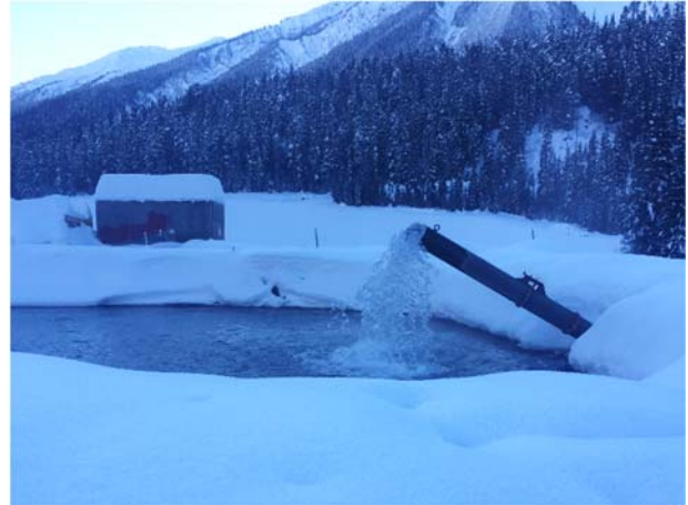
Photo 4 – Dewatering ULRHEF upstream tunnel seepage to the intake sediment basins (November 20, 2015).
