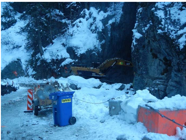
Photo 11 – BDRHEF intake diversion tunnel plug excavation works (November 21, 2015).
