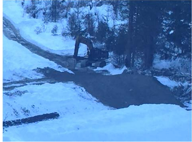
Photo 6 – ASTR04 crossing construction (November 20, 2015).
