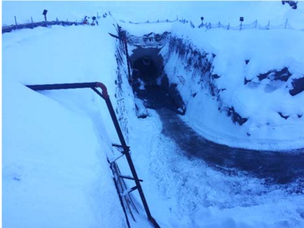
Photo 3 – Current conditions at the ULRHEF upstream tunnel portal (November 20, 2015).
