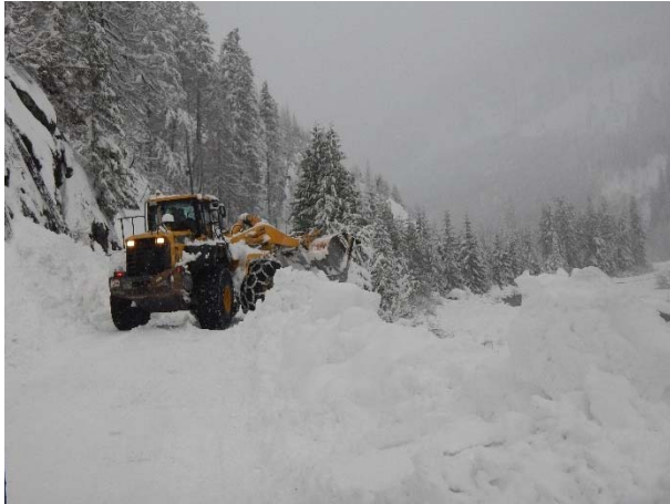
Photo 1 – Snow clearing on the BDRHEF intake access road (November 17, 2015).
