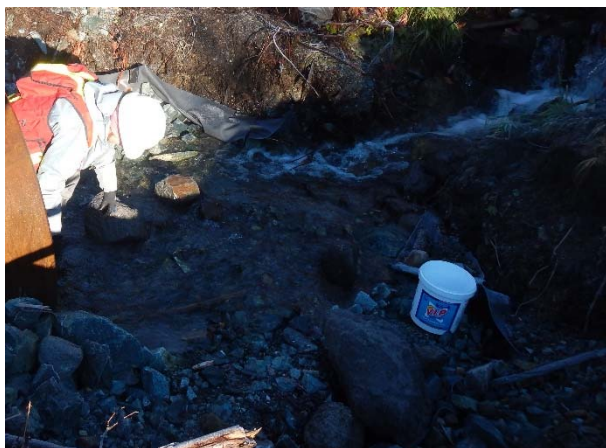
Photo 22 – Ecofish conducts CTF salvage upstream of ASTR04 culvert (November 9, 2015).
