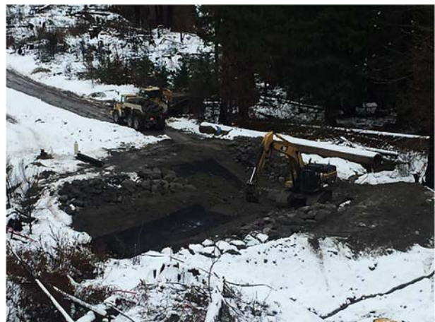
Photo 27 – ASTRO4 overdrain construction with active diversion in place (November 14, 2015).
