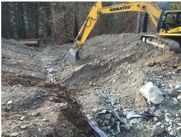
Photo 26 – ASTRO4 overdrain construction with active diversion in place (November 10, 2015).
