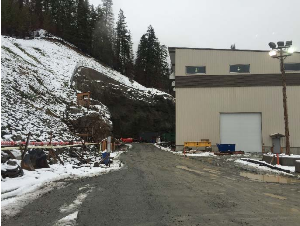
Photo 35 – BDRHEF tunnel portal and powerhouse structure (November 14, 2015).
