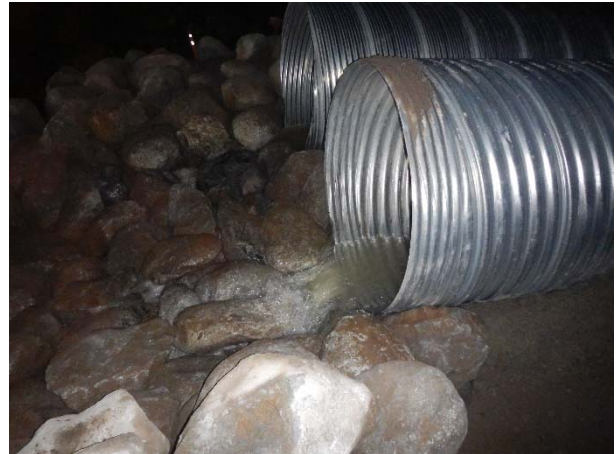
Photo 19 – Flows clearing of sediment following completion of over-drain works (November 8, 2015).
