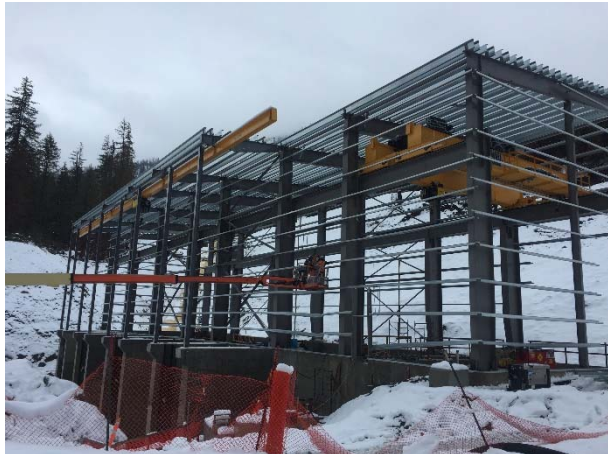
Photo 28 – Current conditions at the ULRHEF powerhouse (November 14, 2015).
