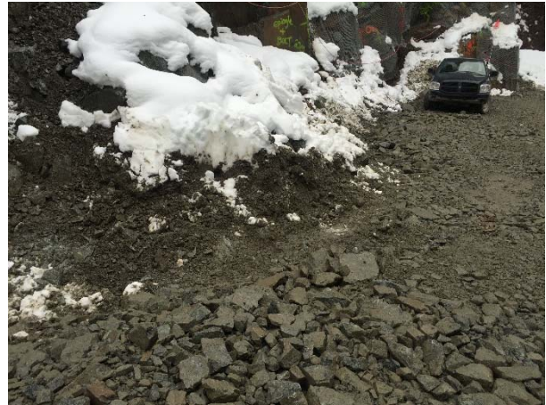
Photo 33 – Road capping and ditching installed on BDRHEF intake access ramp (November 10, 2015).
