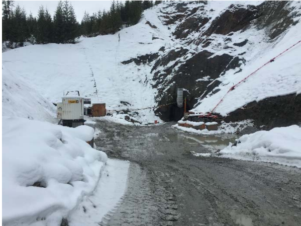
Photo 12 – Current conditions at the ULRHEF downstream tunnel portal (November 14, 2015).
