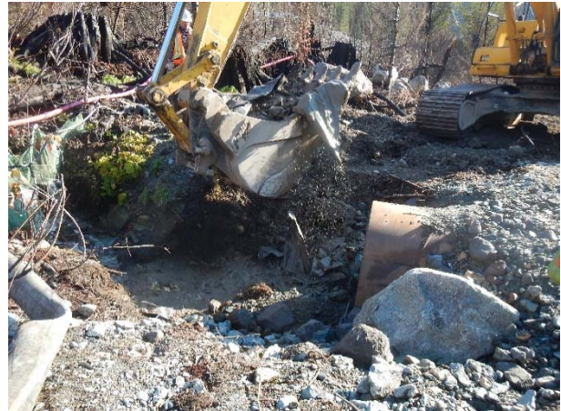
Photo 25 – Culvert removal at ASTRO4 with active diversion in place (November 9, 2015).
