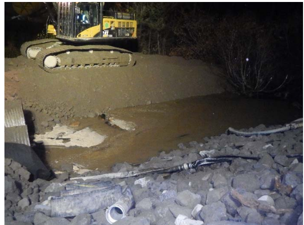
Photo 17 – Berm constructed to introduce flows to over-drain culverts (November 8, 2015).
