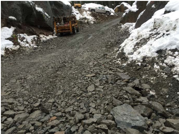
Photo 34 – Road capping and ditching installed on BDRHEF intake access ramp (November 10, 2015).
