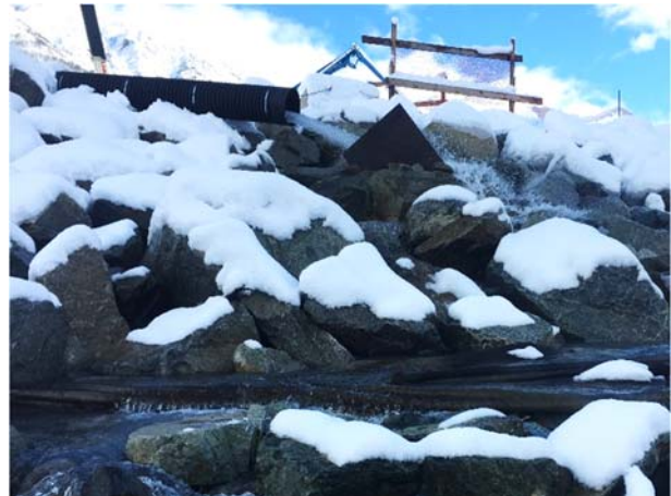
Photo 8 – ULRHEF intake sediment basin outlet pipe at Lillooet River (November 11, 2015).
