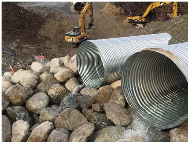
Photo 20 – ASTR03 over-drain with penstock crossing construction in background (November 10, 2015).
