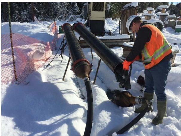
Photo 9 – Flocculant injection system refilled by CE's environmental management team at ULRHEF intake sediment basins (November 11, 2015).
