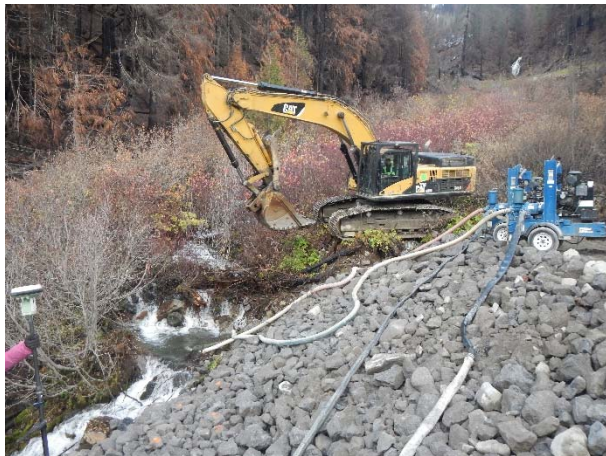
Photo 16 – Pump installation for active diversion at ASTR03 overdrain construction (November 8, 2015).
