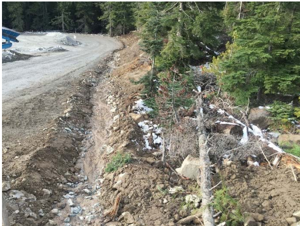
Photo 3 – Ditching completed at KM 45 on the Lillooet River FSR (November 11, 2015).
