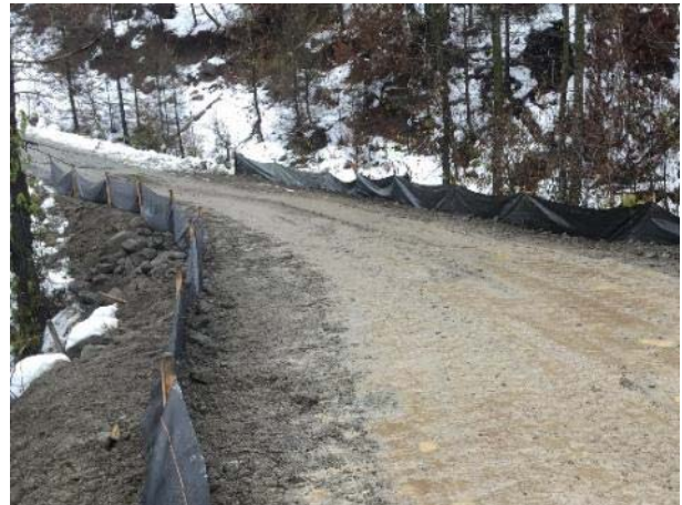
Photo 4 – Road lifted and silt fence re-installed on the haul road ASTR04 crossing (November 14, 2015).
