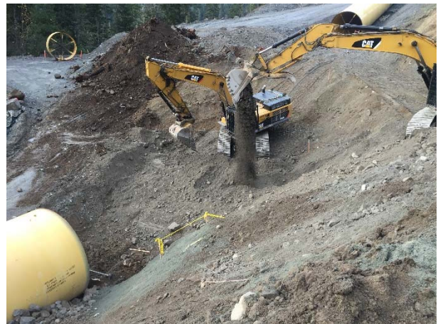
Photo 21 – ASTR03 penstock crossing construction (November 10, 2015).
