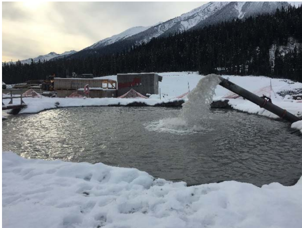
Photo 7 – First cell of ULRHEF intake sediment basins (November 11, 2015).
