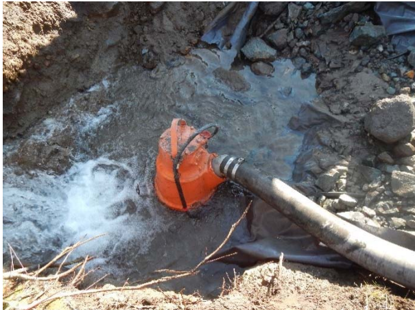
Photo 24 – 6” pump installed for ASTRO4 diversion (November 9, 2015).
